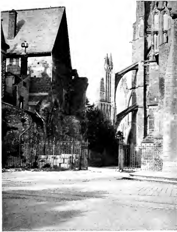
"THE ARMS OF FLYING-BUTTRESSES STRETCH FROM THE CATHEDRAL TO THESE . . . SUPPORTS."—TOURS.
