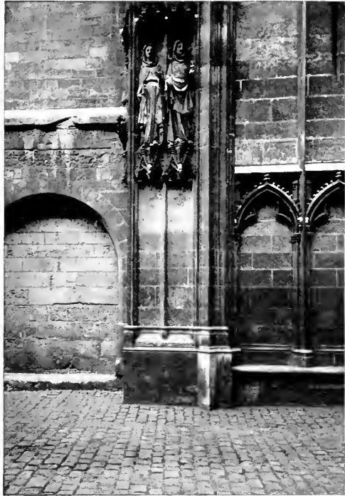
"THE DARK, LATERAL WALLS OF THE 'PASSAGEWAY' ARE ORNAMENTED WITH BLIND ARCADES AND STATUES OF SAINTS IN NICHEs."—ROUEN.
