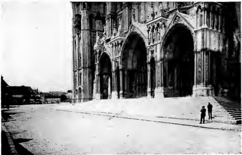
"PORCHES WERE ADDED TO THE . . . ENTRANCES OF THE TRANSEPTS."— CHARTRES.
