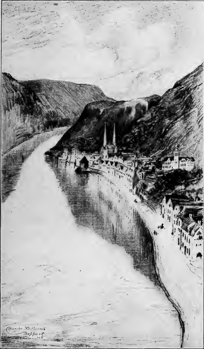
G ENERAL VIEW of BOPPART
