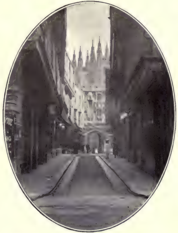
MERCERY LANE, LOOKING TO CHRIST CHURCH GATEWAY.
