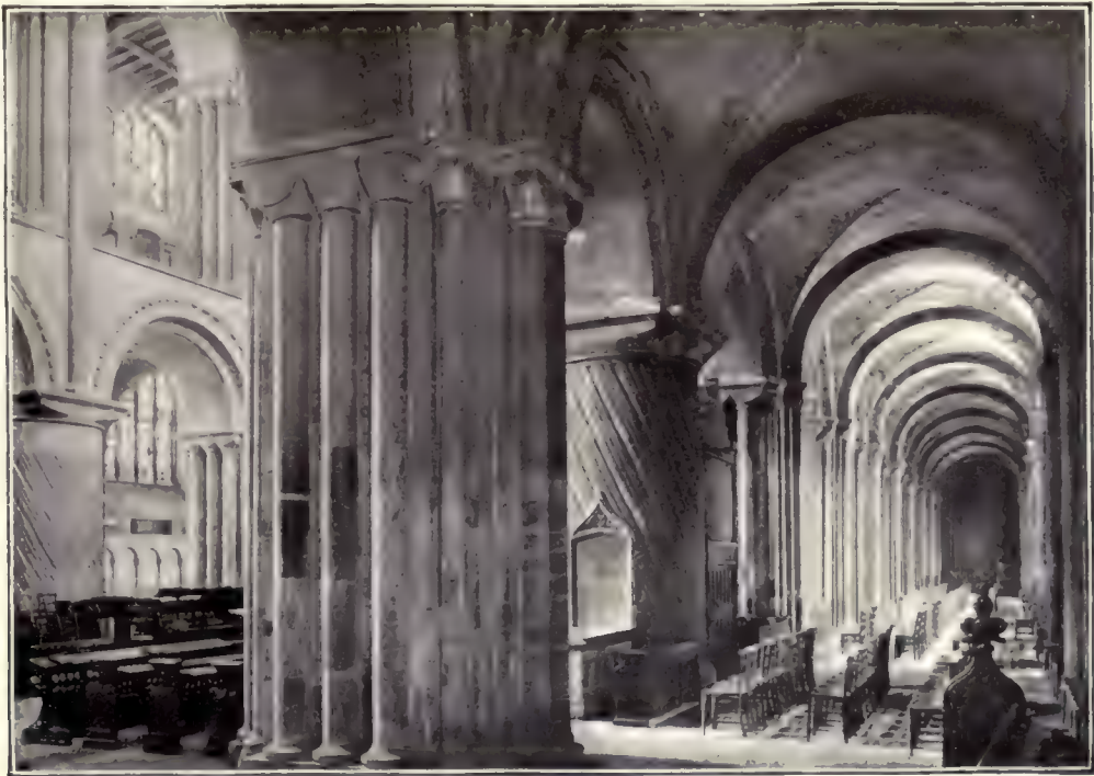
THE NORTH AISLE OF THE NAVE, LOOKING WEST.
