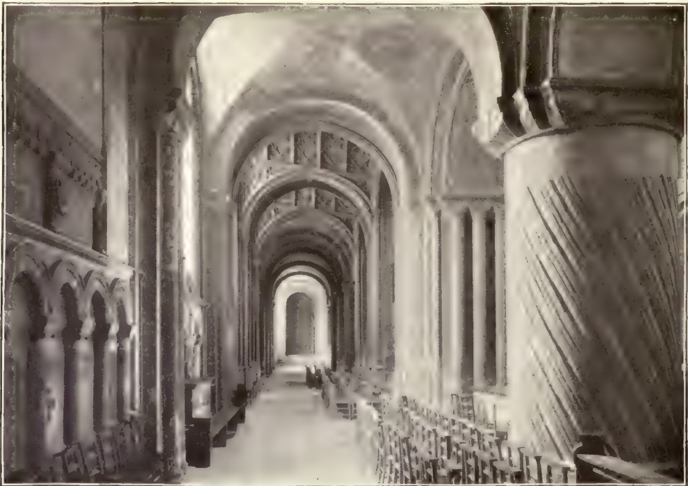
THE SOUTH AISLE OF THE NAVE, LOOKING WEST.
