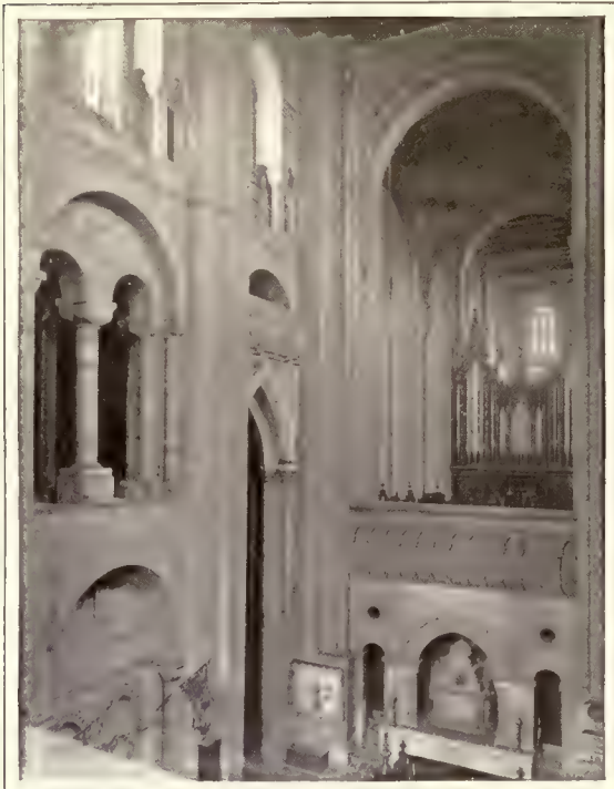
ONE OF THE PIERS THAT SUPPORT THE TOWER OF THE CATHEDRAL.
