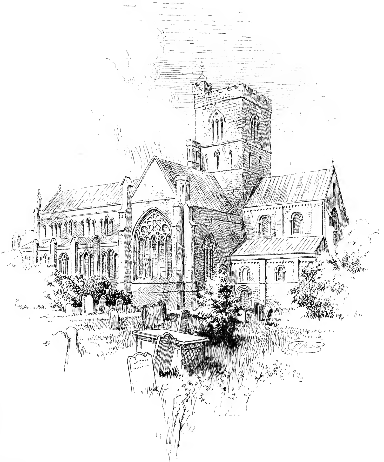
Carlisle from S E
