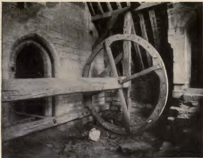
WINDLASS USED IN BUILDING PETERBOROUGH CATHEDRAL
