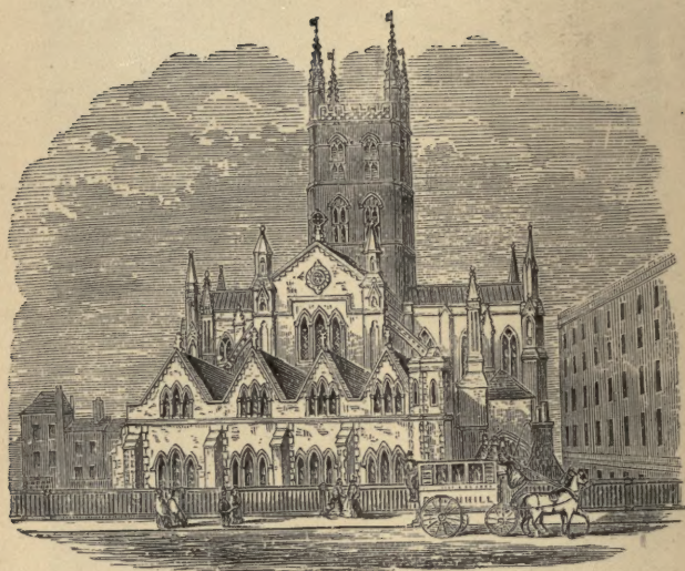
1b. EAST ASPECT. As seen from the Southern Approach to London Bridge.
