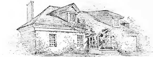
ST. JOSEPH'S CHAPEL HOUSE, DEER CREEK, HARFORD CO., MD. FROM A SKETCH BY GEO. A. TOWNSEND.
