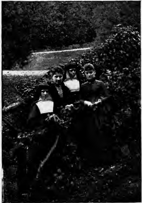
A GROUP AT THE BRIDGE.
