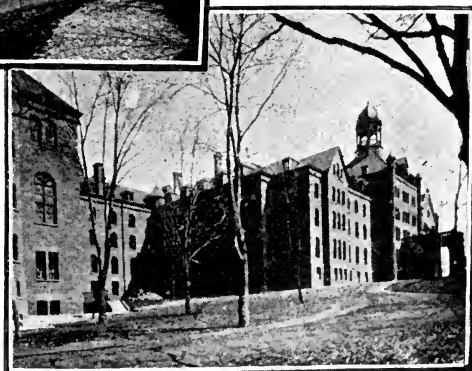
VIEWS ABOUT THE NEW CONVENT AFTER THE RESTORATION.
