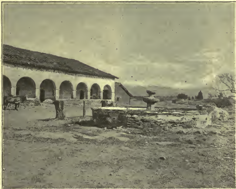
THEIR YEARLY ENCROACHMENTS LEAD TO THE VERY DOORS.
