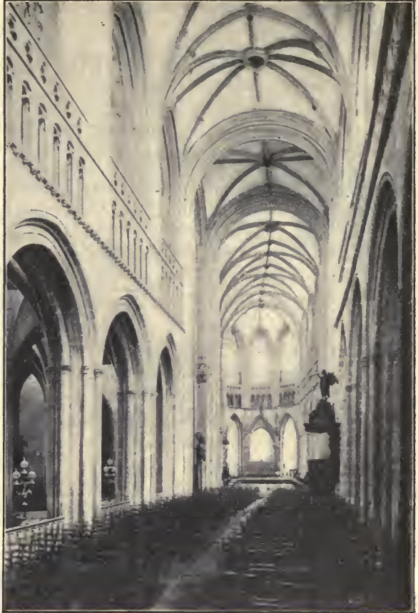
THE LEANING NAVE OF THE CATHEDRAL.
