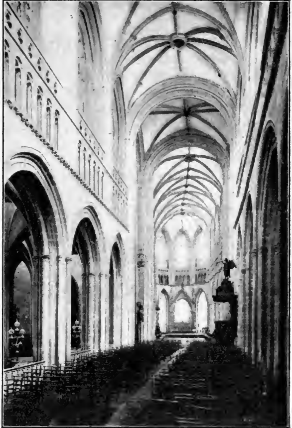
THE LEANING NAVE OF THE CATHEDRAL.
