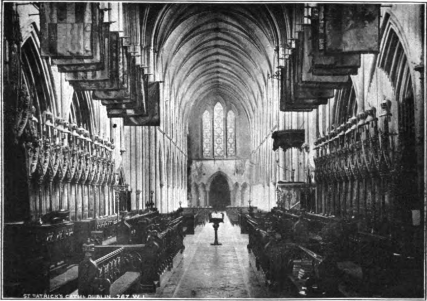
INTERIOR VIEW OF ST. PATRICK'S.
