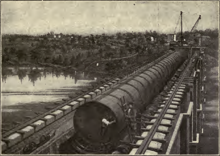
Laying 90-inch Pipe of Croton Aqueduct on High Bridge in 1861
