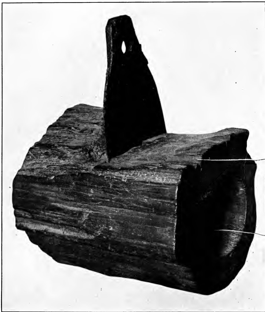
WATER GATE IN THE PIPES LAID BY THE MANHATTAN COMPANY, INCORPORATED APRIL 2, 1799
