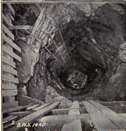
Contractor's plant at the top of a City Tunnel shaft (1); (2) a reinforced concrete caisson being sunk through sand and rock for a shaft in Brooklyn; (3) interior of a valve chamber on top of a finished shaft; (4) a shaft top nearing completion showing a riser pipe and shaft cap; (5) looking down into a shaft during the process of sinking; and (6) steel riser pipes in a shaft ready to be imbedded in concrete.
