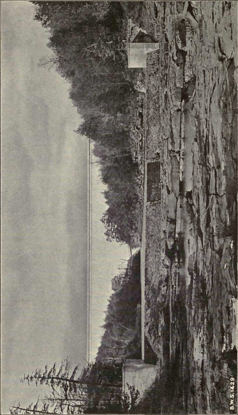
Downstream face of the masonry portion of Olive Bridge dam, from a point in the gorge. Note the rocky bed of Esopus creek and the low, rustic stone dam holding the water in the pool at the toe of the large dam.
