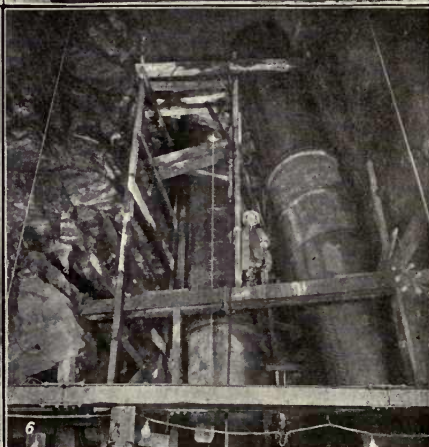
Contractor's plant at the top of a City Tunnel shaft (1); (2) a reinforced concrete caisson being sunk through sand and rock for a shaft in Brooklyn; (3) interior of a valve chamber on top of a finished shaft; (4) a shaft top nearing completion showing a riser pipe and shaft cap; (5) looking down into a shaft during the process of sinking; and (6) steel riser pipes in a shaft ready to be imbedded in concrete.
