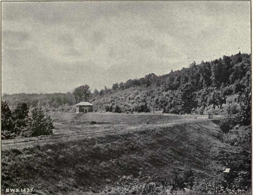
Peak gaging chamber in Catskill aqueduct south of Peak tunnel.
