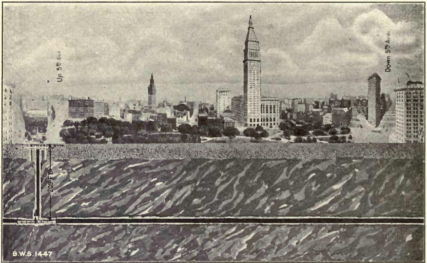
A full circle panorama of New York City's streets around Madison Square showing Shaft 18 and a portion of the City tunnel, in the rock more than 200 feet beneath the surface. Madison Square Garden tower, the Metropolitan tower and Flatiron Building are easily recognized from left to right.
