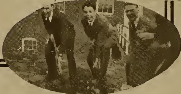
Midnight "Oil" The excavators.
