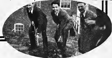
Midnight "Oil" The excavators.
