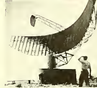
Forty-foot antenna of harbor surveillance radar.
