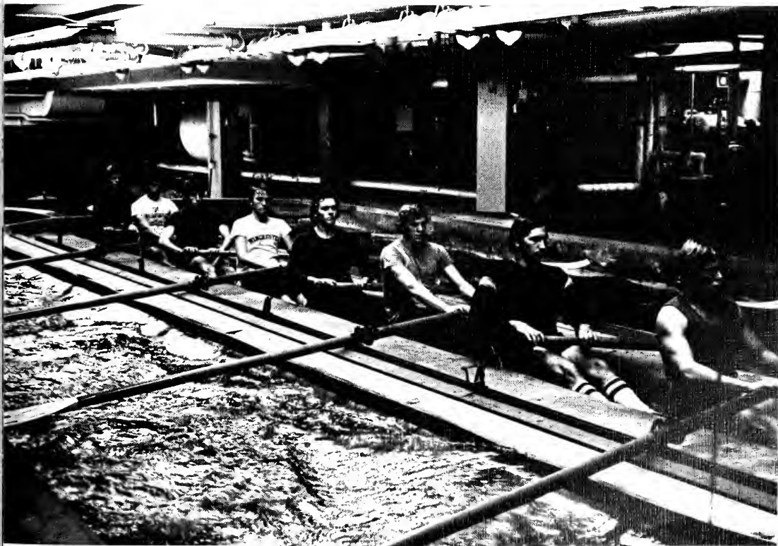
The crew tank, in the basement of the Cabot Cage
