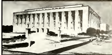
1938 The West Building, completed in '38, became Richards Hall in 1941.
