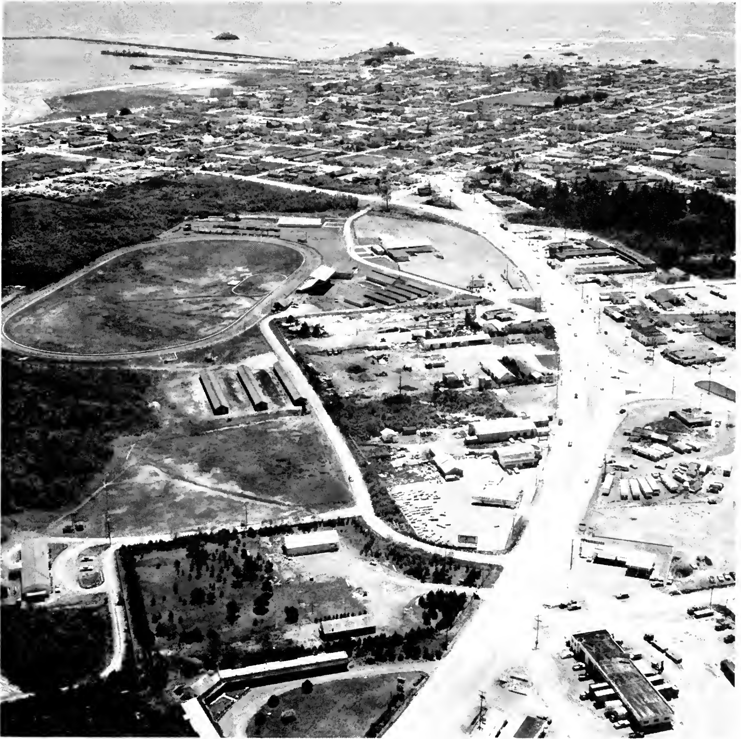
A recent improvement made US 101 through Crescent City in Del Norte County a one-way couplet with four-lane approaches. This southwest view shows the US 101-Northcrest Drive intersection in the right center.
