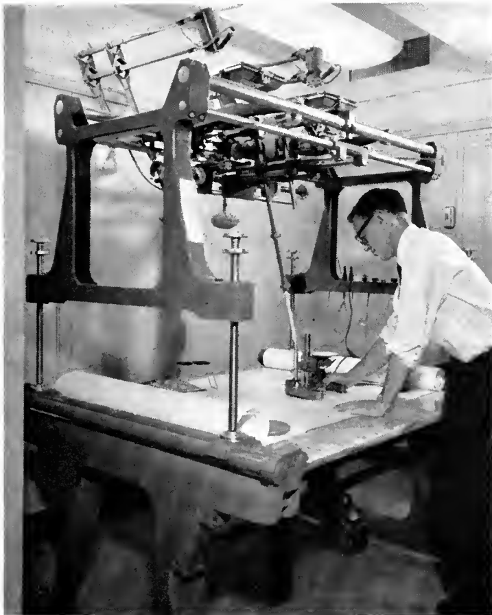
LEFT—Photogrammetrist Brennan Davis operates one version of stereo-platter, complicated mechanism for stereo-picture projection for map making. For accurate work, machine must be sturdy and built to close tolerance. RIGHT—Davis demonstrates use of stereo-platter. A three-dimensional image is projected on white disk. The operator wears special glasses, one lens red, the other blue, to get three-dimensional effect. The machine traces contours as operator allows apparent relief.
