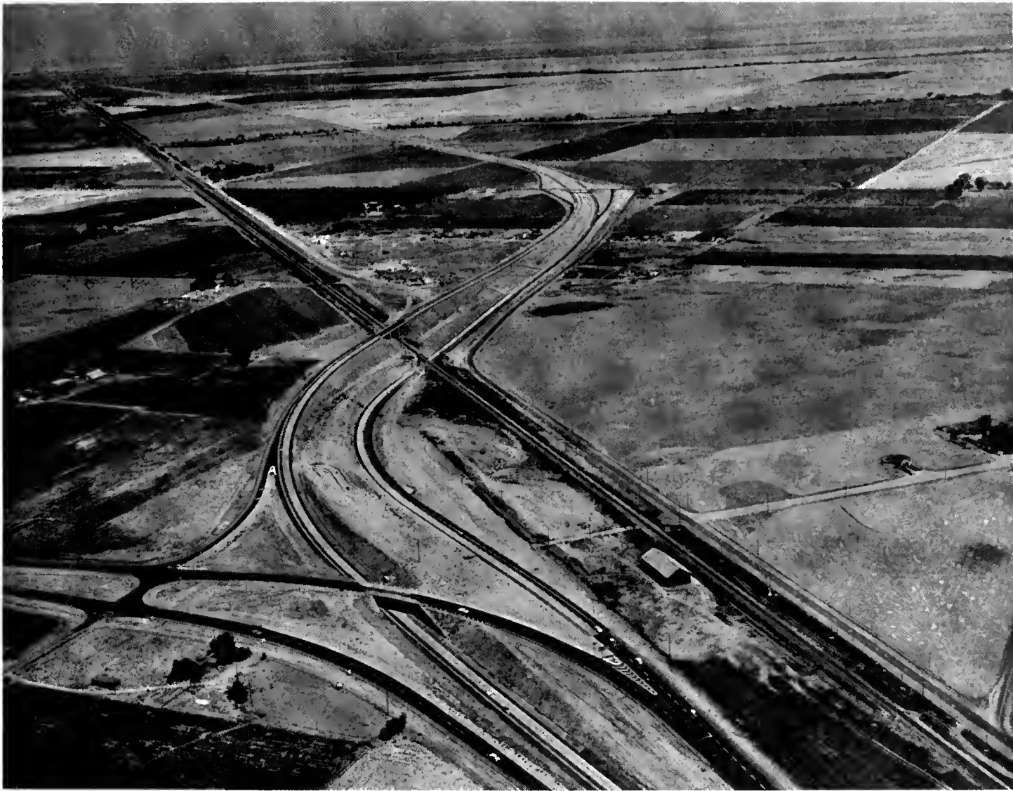
A view northward taken from the south end of the Chowchilla Bypass. The separation structure in the foreground connects US 99 and State Route 152. Beyond, the southbound lane crosses the railroad tracks on an overhead while the northbound lanes use an underpass.
