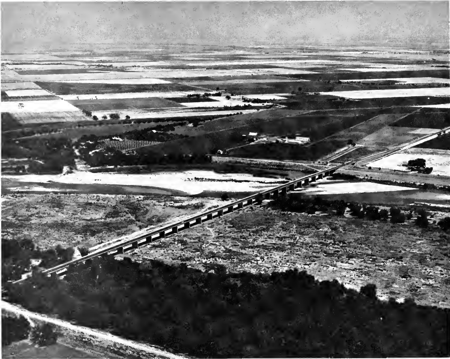
Replacing the structure washed out in the floods of December, 1955, this modern concrete girder bridge now carries traffic across the Feather River near Nicolaus. Cost of the bridge and its immediate approaches was $2,300,000. Site of the old bridge is marked by the open space through the trees of the town of Nicolaus (left center).
