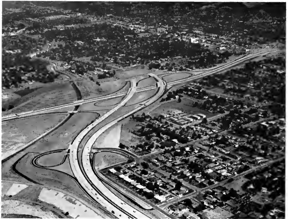
This view to the northeast along the Ventura Freeway shows the interchange with the San Diego Freeway.
