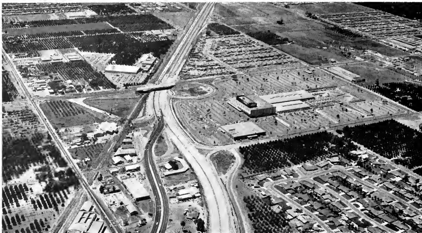
Looking northwest along Santa Ana Freeway under construction between City of Anaheim in foreground and City of Buena Park in background. In center is Broadway-Anaheim shopping center.
