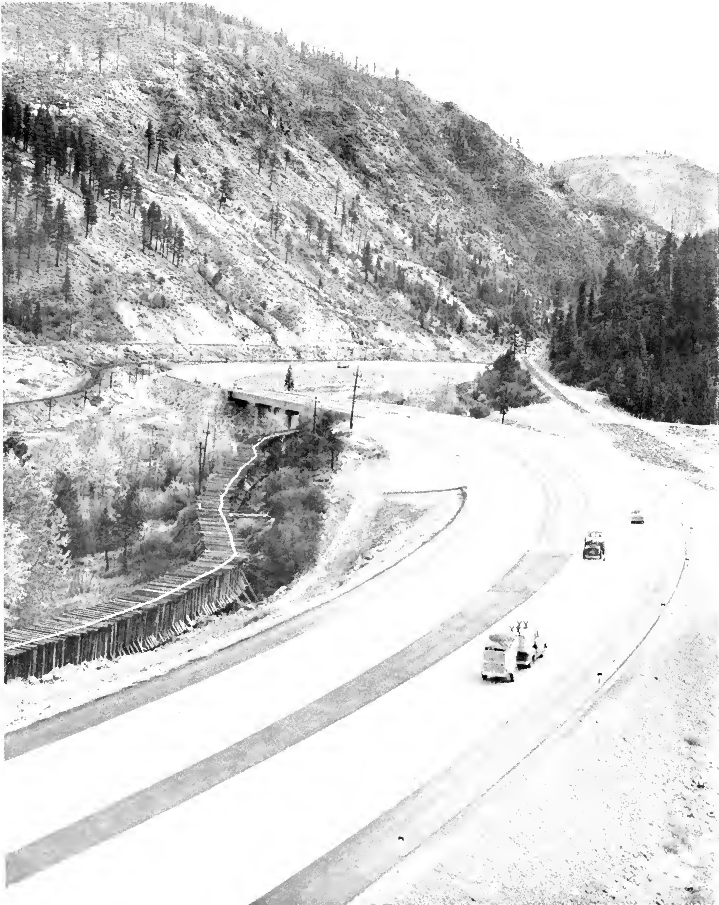
Recently completed section of US 40 (Interstate 80) in Truckee Canyon a few miles west of California Nevada state line (see page 2).
