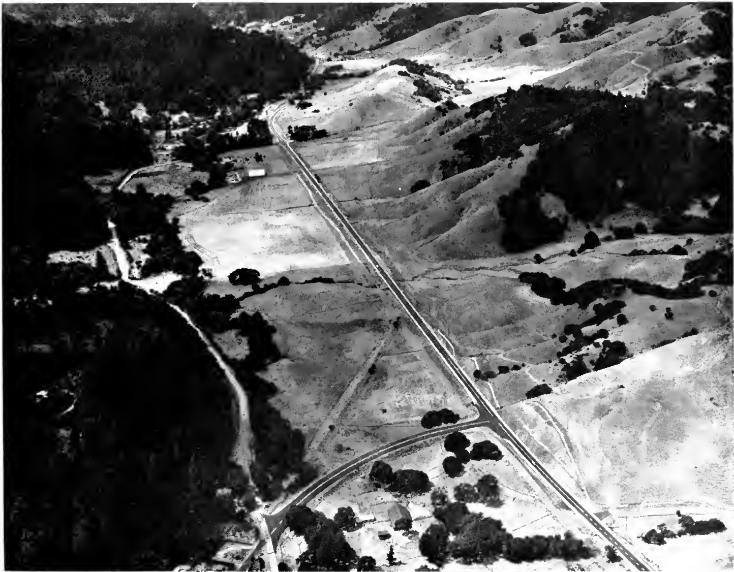
Marin County's Federal-aid Secondary Route 608, Sir Francis Drake Boulevard, recently completed under three contracts. Former route may be seen at left. Woodacre connection is in foreground.
