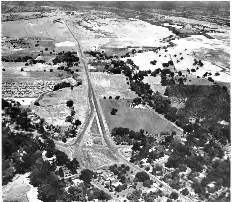
UPPER—Relocation of US 40 Alternate along the Feather River between Wicks Corner and Jarbo Gap. A dual-purpose bridge carrying the highway and railroad over the West Branch of the Feather River, which extends from left to right across the center of the picture, will connect the two visible construction areas. LOWER—An aerial view eastward of the State Sign Route 32 improvement between Chico and Hog Springs. A portion of the one-way couplet in Chico shows in the foreground.
