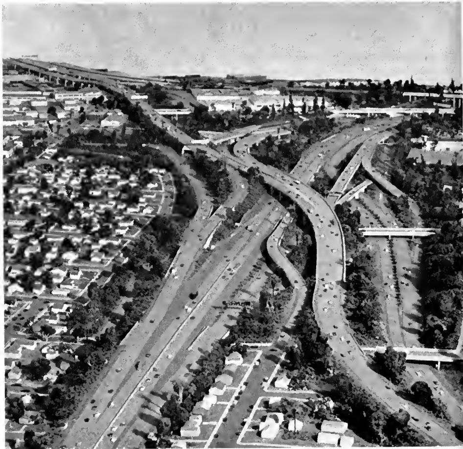
This closeup of the freeway model gives some idea of how the future East Los Angeles interchange will appear looking west along the Santa Ana Freeway
