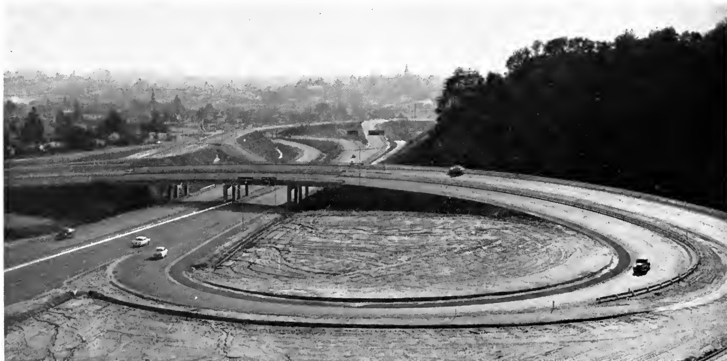
The Morrissey Avenue interchange in Santo Cruz. Beyond are the ramps connecting Sign Route 17 with Sign Route 1.
