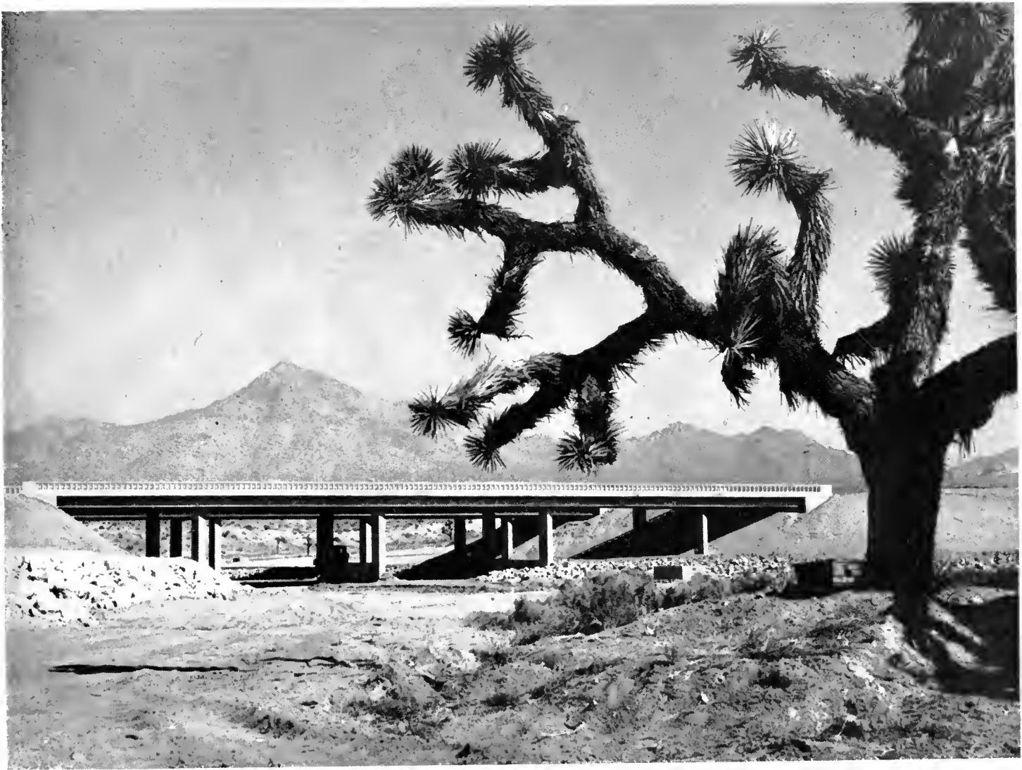
A typical drainage facility along the new freeway is the Bell Mountain Wash Bridge, shown above
