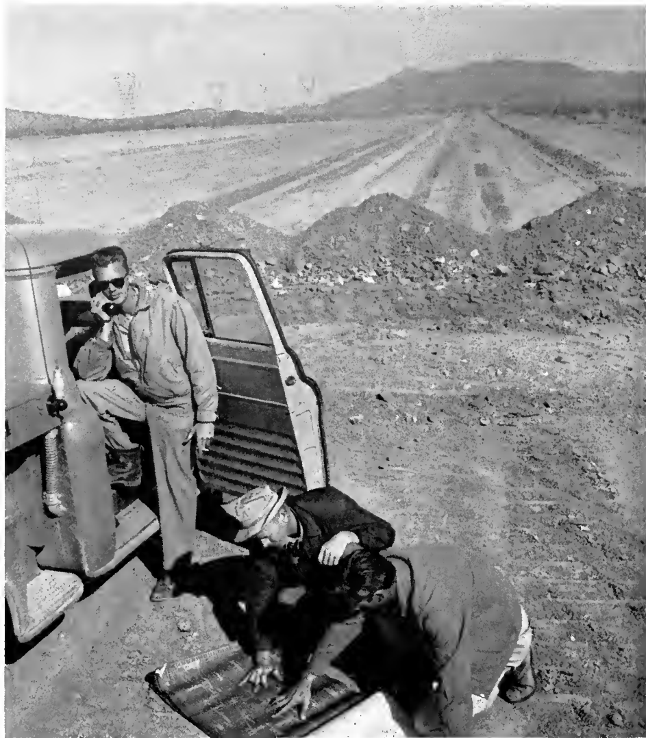
Inspectors using radio to check blueprints out in the wide open spaces on the Victorville-Borstow expressway are, left to right, W. T. Murray, Art Austin and R. H. T. Norton
