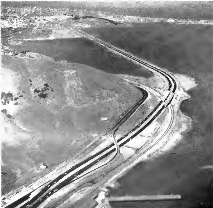
The Bayshore Freeway link between Candlestick Point in San Francisco and Sierra Point in San Mateo County was placed in operation in 1957. The new freeway section (left) is built on an earth fill across open water at the edge of San Francisco Bay. Below is a photograph taken in 1954 during an early stage of the project.
