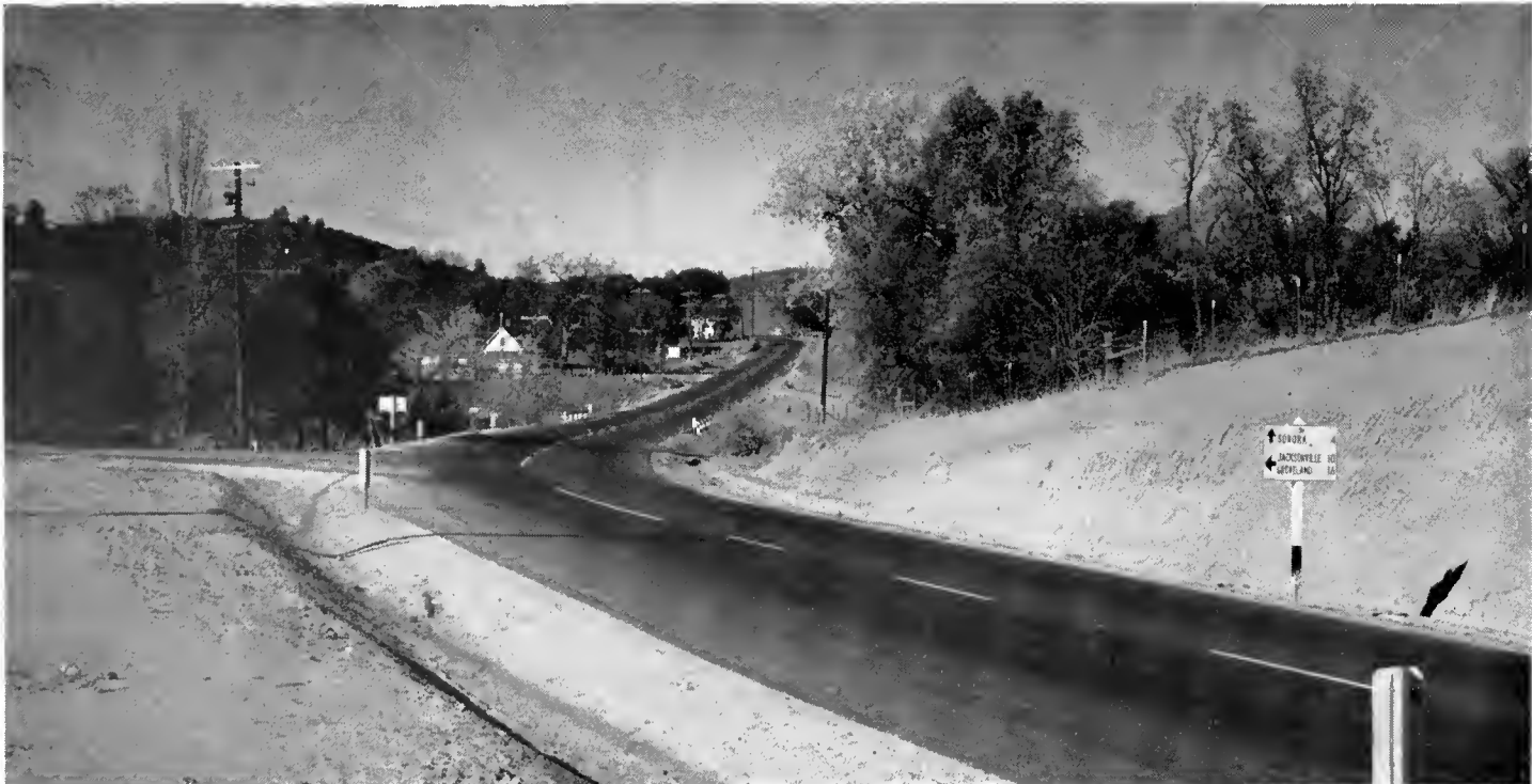
A section of the recently completed Tuolumne County Federal Aid Secondary project shows the Wards Ferry Road connection on the left
