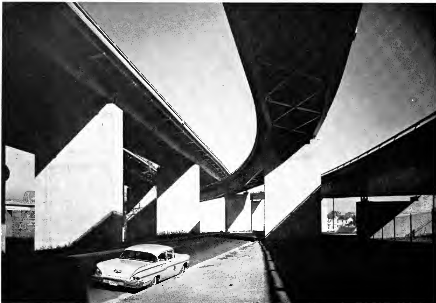
An interesting camera study of the southern approach ramps to the twin bridges taken from one of the city streets in Crockett.
