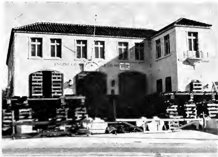
A fire station in the City of Los Angeles is relocated to clear right-of-way for the Hollywood Freeway. LEFT—Shows the building blocked up just before being moved. RIGHT—Shows the same building after it had been re-established and placed in use by the Los Angeles Fire Department in its new location.
