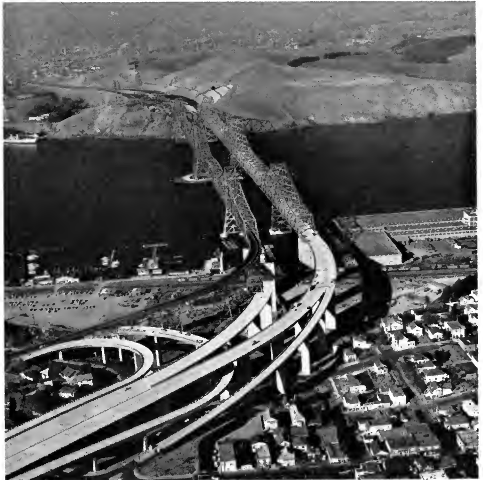
Symbolizing California's spectacular progress in highway development is the parallel Carquinez Bridge on US Highway 40 at Crckett (right) and its extensive freeway approaches which were opened in November, 1958. Construction began on the $46,000,000 toll project in late 1955.
