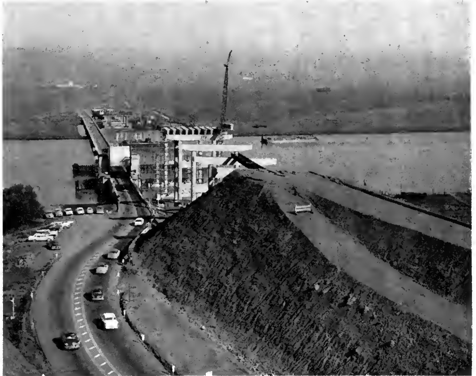
Looking east over the Petaluma Creek project. The partially completed fill in the foreground will be finished after two lanes of the new bridge are opened to traffic.
