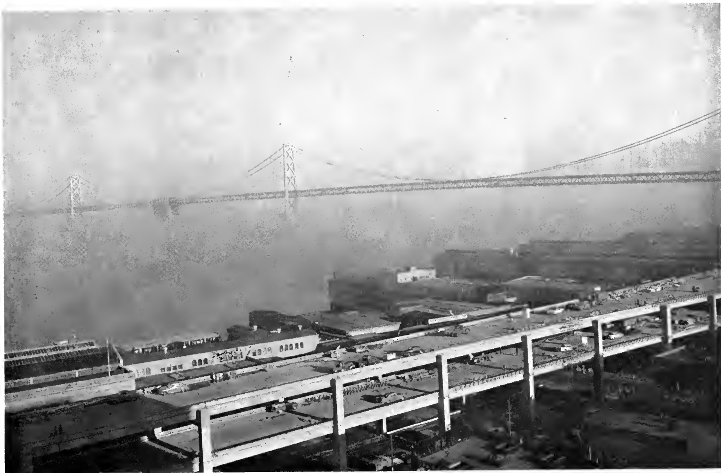
Another view of the Embarcadero Freeway Viaduct under construction looking eastward with the San Francisco-Oakland Bay Bridge rising out of the fog.
