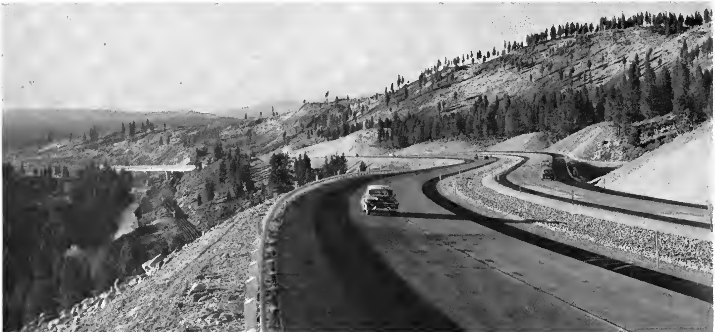
Baca Bridge and Overhead upper left with Southern Pacific freight passing beneath. Looking west near upper end of Truckee Canyon.
