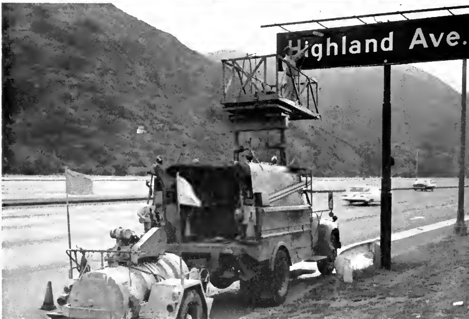
UPPER—On sections where an inside lane must be closed to wash signs, the work is done during a time when traffic is light, usually from daylight to 9 a.m. on Sunday. A flagman is always used to afford further protection to the men and equipment. LOWER—Signs such as this one on the Cahuenga Pass section of the Hollywood Freeway are cleaned from a tower lift on a truck parked on a paved shoulder.
