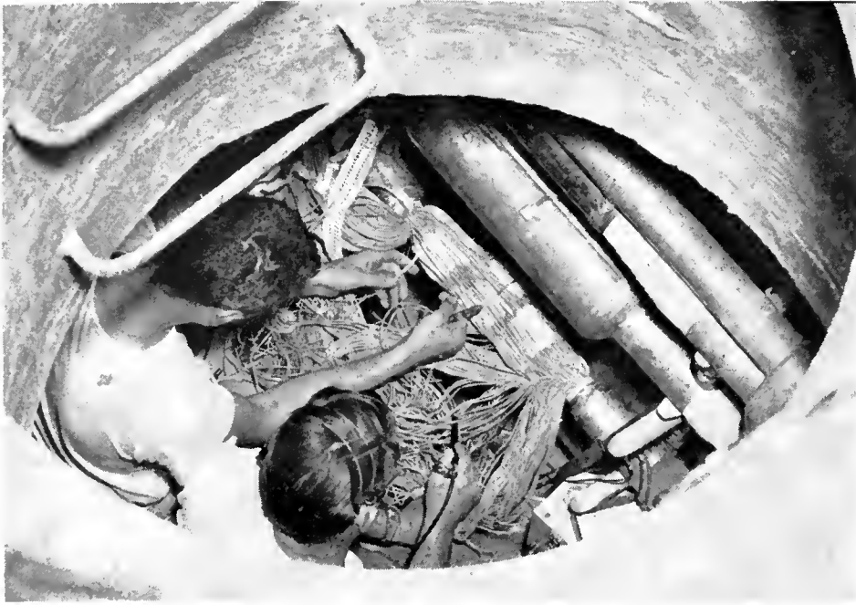
ABOVE—Skilled workmen splice one of the more complex telephone cables. RIGHT—Shows temporary relocation of telephone cables during the construction of the Hollywood Freeway at Vermont Avenue.
