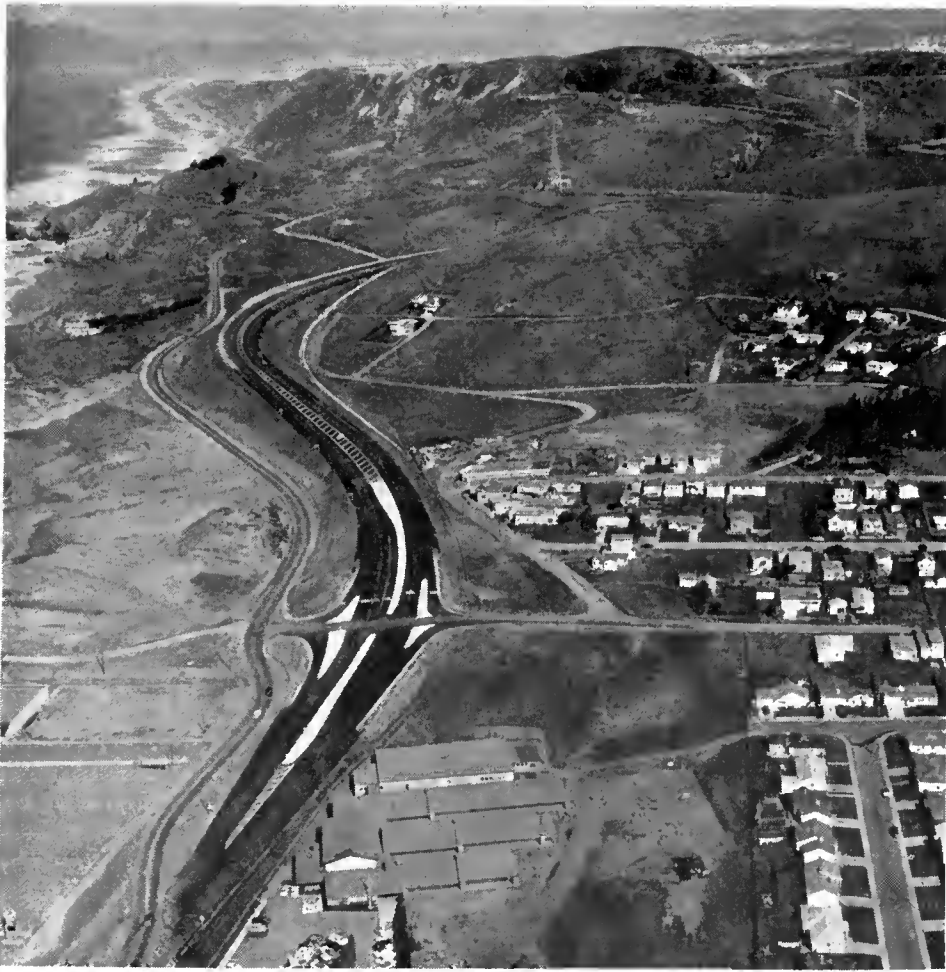
New expressway is being constructed on State Sign Route 1 between Pacifica and Skyline Boulevard just south of San Francisco. Note the old highway on the left which is benched into the bluffs to the north.
