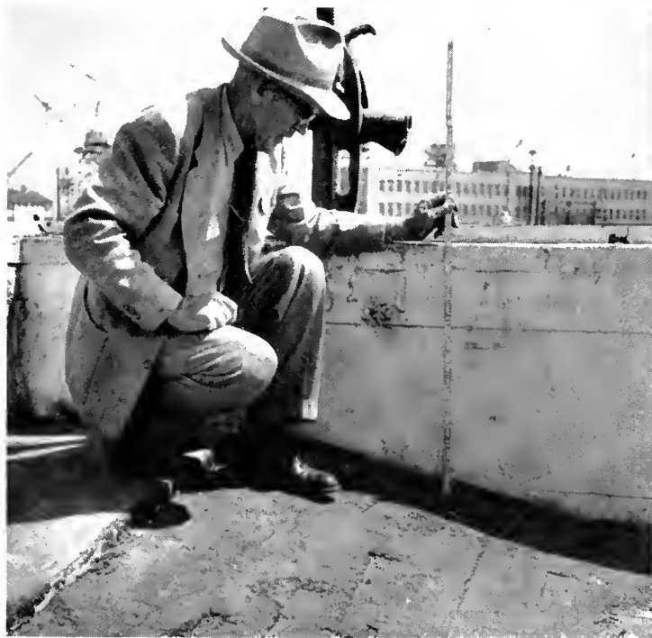
Slab floor of old building settled seriously on tide land fill. Archie Prescott of Navy Public Works here shows where supplementary asphalt ramp had to be built to accommodate warehouse rolling stack.
