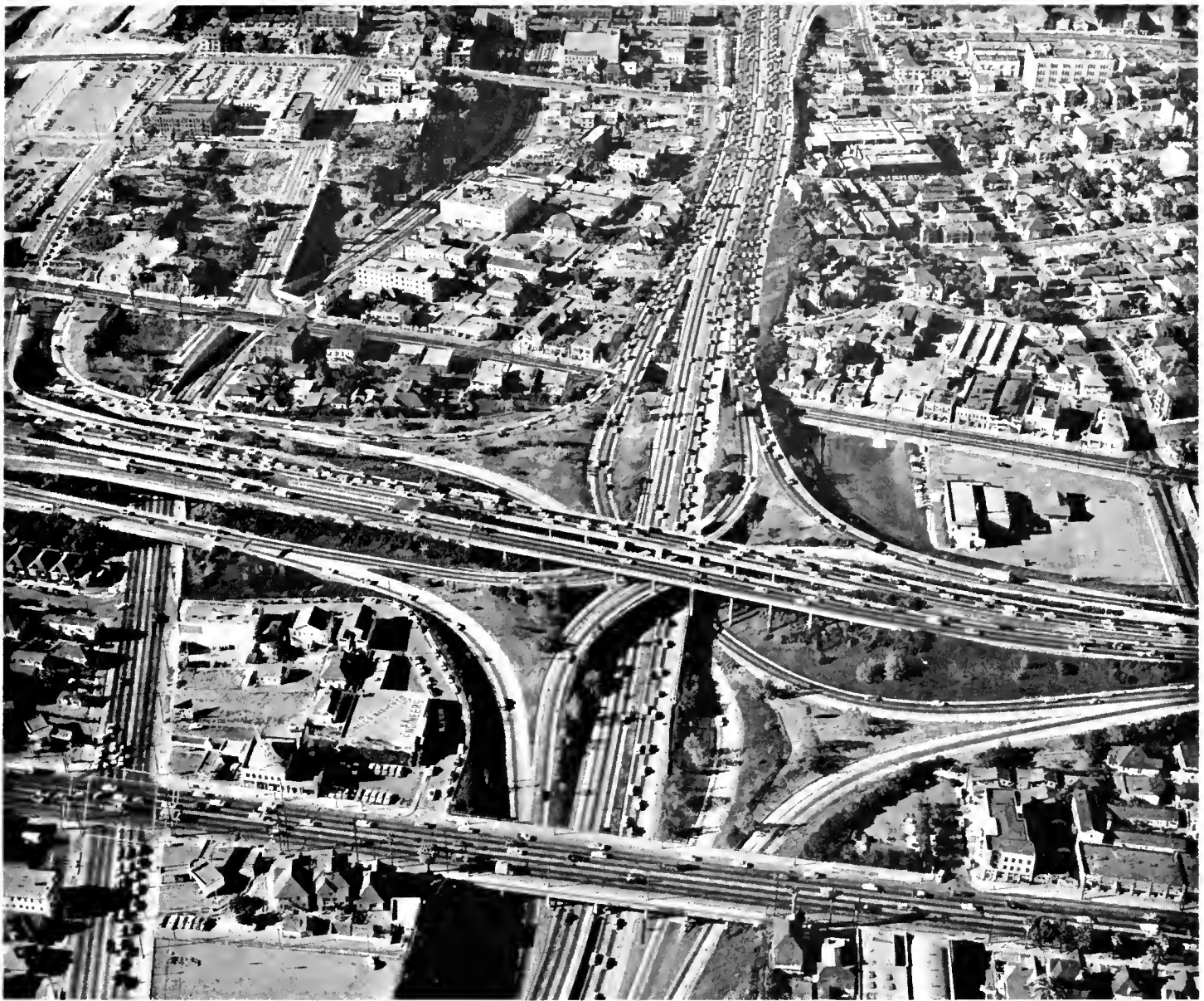
The much photographed yet always intriguing four-level structure in downtown Los Angeles. The camera looks south along the Pasadena-Harbor Freeway.
