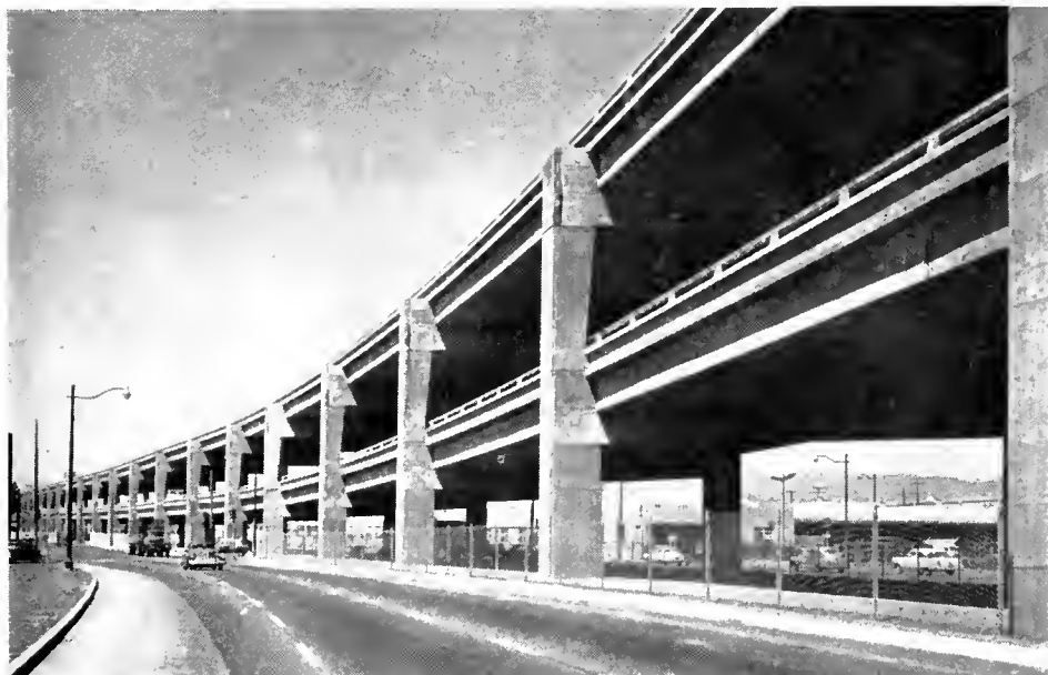
The Cypress Street Viaduct in Oakland, first double-deck freeway in the State, was completed and opened to traffic in 1957. It is a unit of the Eastshore Freeway.
