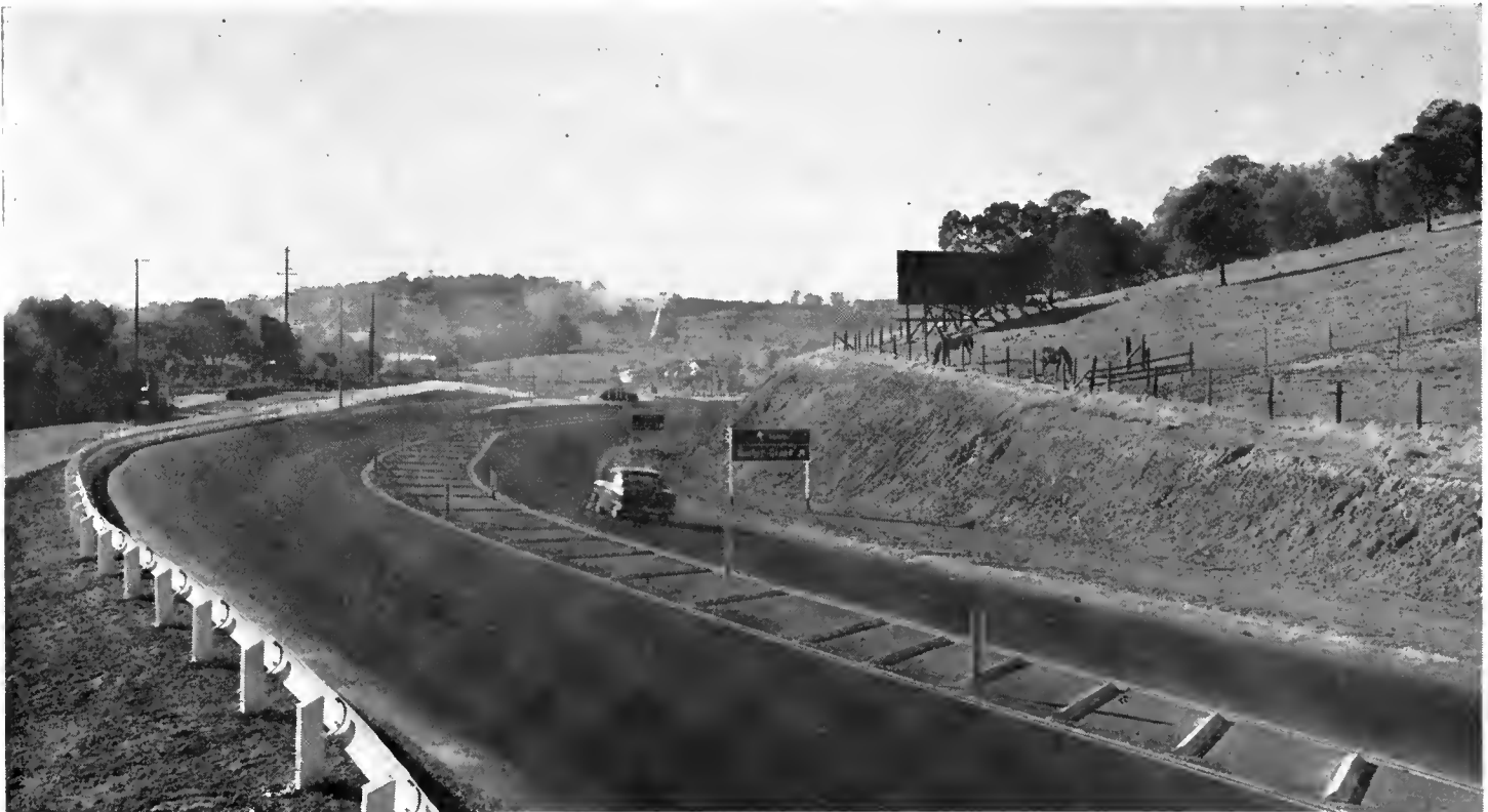
The Martell Junction looking northwest. The highway in the foreground is combined Sign Route 88-49 with Sign Route 88 to Ione bearing left and Sign Route 49 North bearing to the right.
