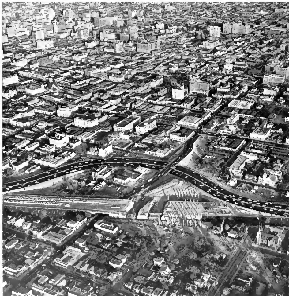
This view northeast toward downtown Los Angeles shows the detour now in operation on the Harbor Freeway while bridges for the future interchange with the Santa Monica Freeway are being constructed.
