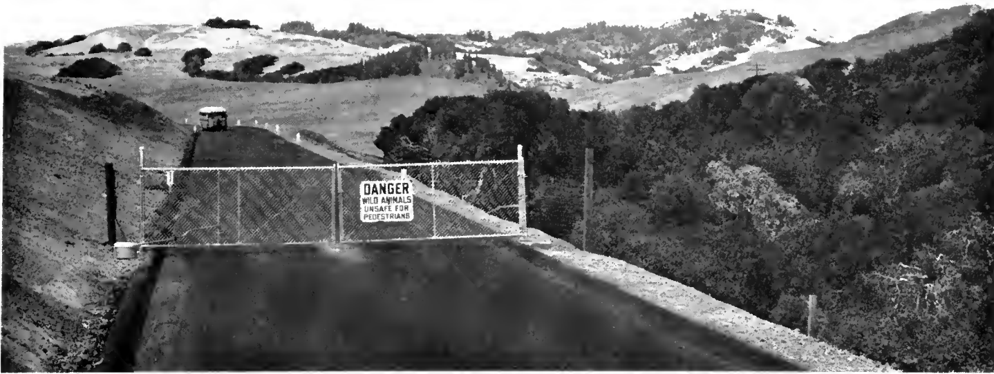
Reconstruction of the Hearst Castle access road was a co-operative project of the Division of Beaches and Parks and the Division of Highways. The castle can be seen on top of the ridge to the right.
