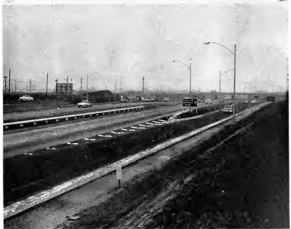
UPPER—Giant scissors cut a ribbon and open to traffic the most recently completed section of the Eastshore Freeway. LOWER—The Jackson Street separation shortly after the freeway was opened to traffic.
