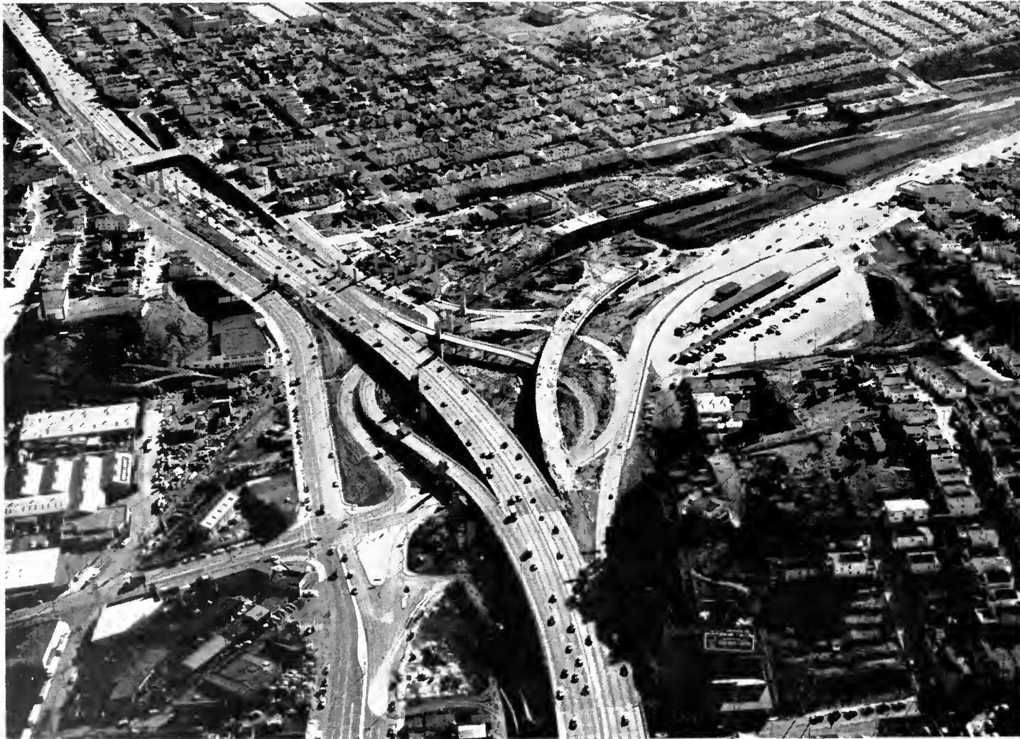
When completed this interchange on the James Lick Memorial Freeway (Boysshore) in San Francisco will connect with the first unit of the Southern Freeway under construction in the right middleground.
