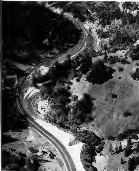
CK COVER —Looking northerly along the new section of freeway on U.S. 101 (The Redwood Highway), in Rattlesnake Creek Canyon, about 12 miles north of Laytonville. (See Report From District I, page 31.)
