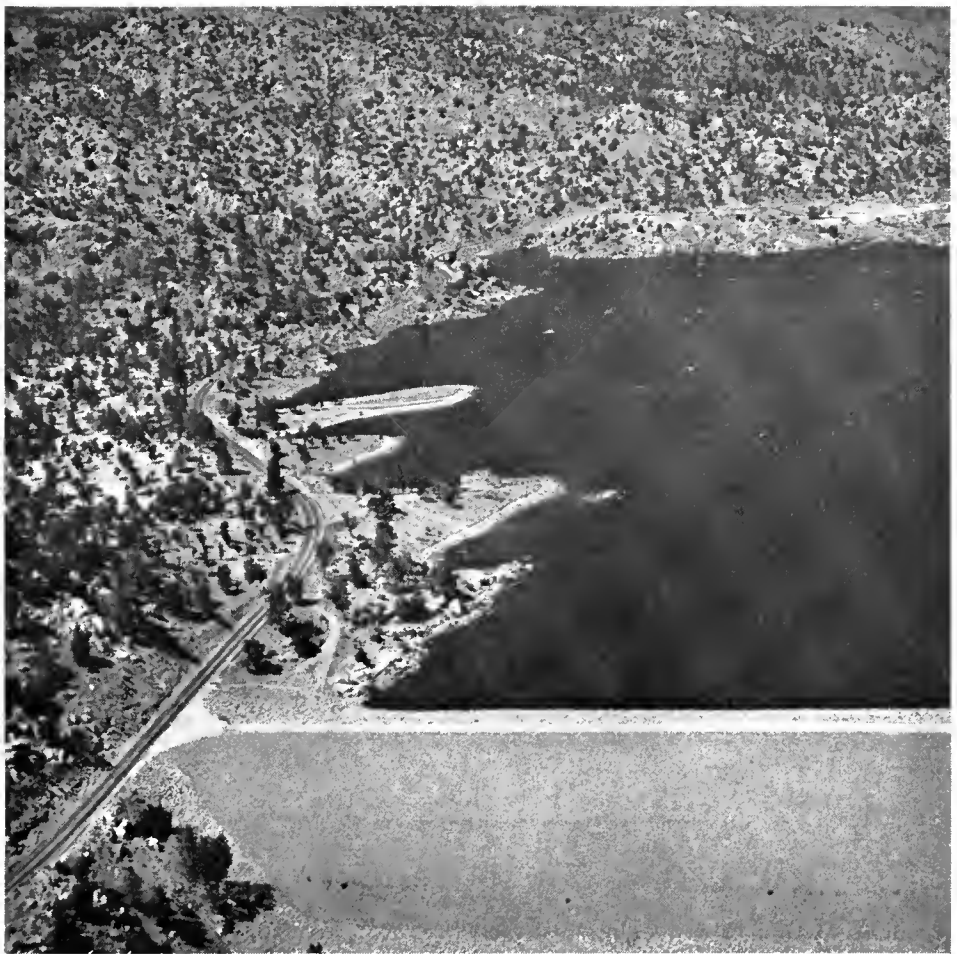
Looking north along Sign Route 178 toward Kernville from the west end of the main dam at Lake Isabella in Kern County
