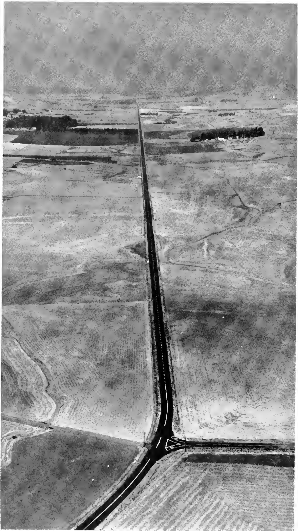
This newly constructed county road between San Luis Obispo and Baywood Park on the coast serves the commuting traffic between these two communities as well as the farms and ranches along the route. Although the highway visible in the picture is absolutely straight, it curves in the distance and heads through the hills to the left.
