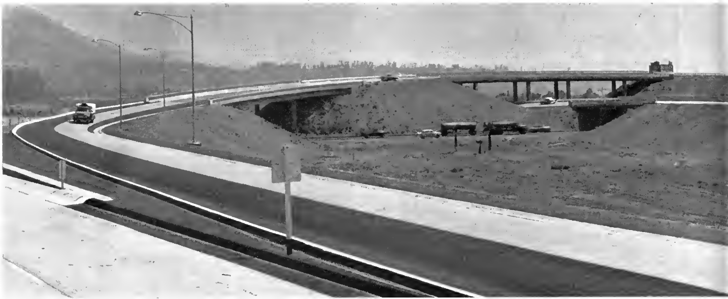
The three-level Colton interchange connects US 70-99 with US 91-395. Lowest level is US 70-99 westbound toward Los Angeles.
