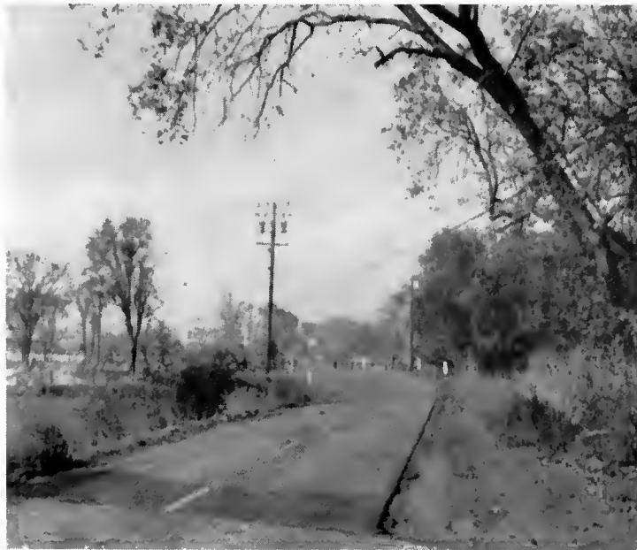
Before and after construction views of the alignment at one of the bridges on Silverado Trail, Federal-Aid Secondary Route 607. The new alignment provides large radius curves with smaller interior angles and greater sight distances.
