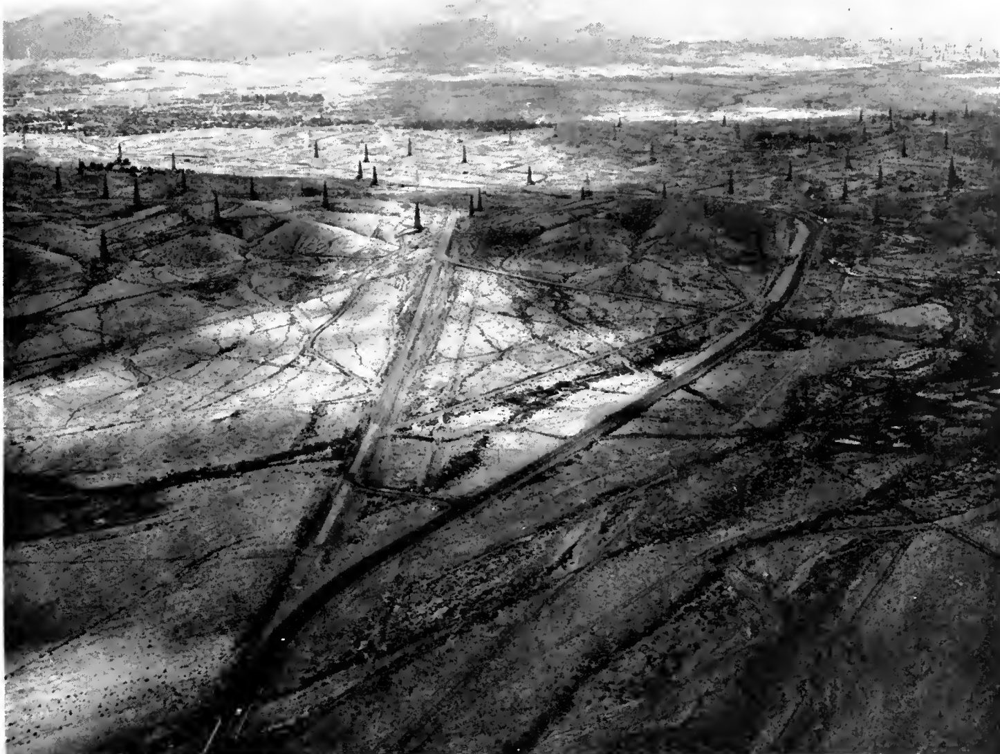
US 399 in Kern County has been relocated around Hill 36. Note the old highway leading directly across the hill (center). Fard City and Taft can be seen in the left background.
