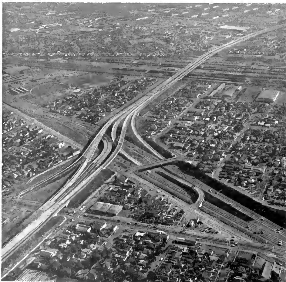
This aerial photograph, taken just east of Los Angeles Civic Center, shows recent, current and coming freeway construction in one view. Traffic on the Santa Ana Freeway moves along smoothly under the bridges which carry the Long Beach Freeway. The section of the Long Beach Freeway extending upward (south) from the interchange was recently opened to traffic, while construction is scheduled to start in 1958 on the northward extension for which preparation is evident at bottom left.
