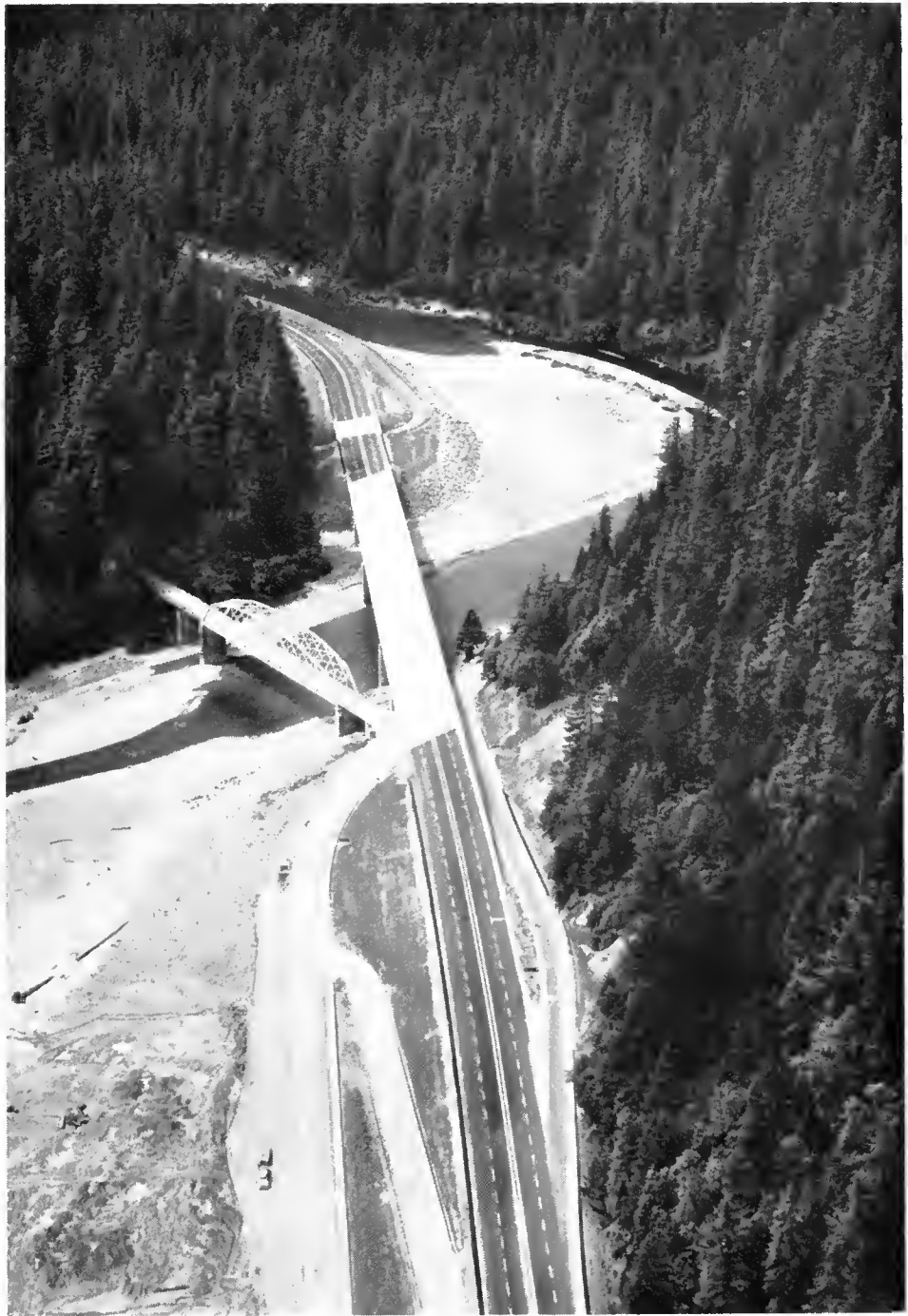
A view southward showing the new George M. Leatherwood Memorial Bridge on the recently completed first unit of the Redwood Parks Freeway (US 101) at Dyerville in Humboldt County. The old highway bridge can be seen to the left of the new one. (See photo on page 25.)
