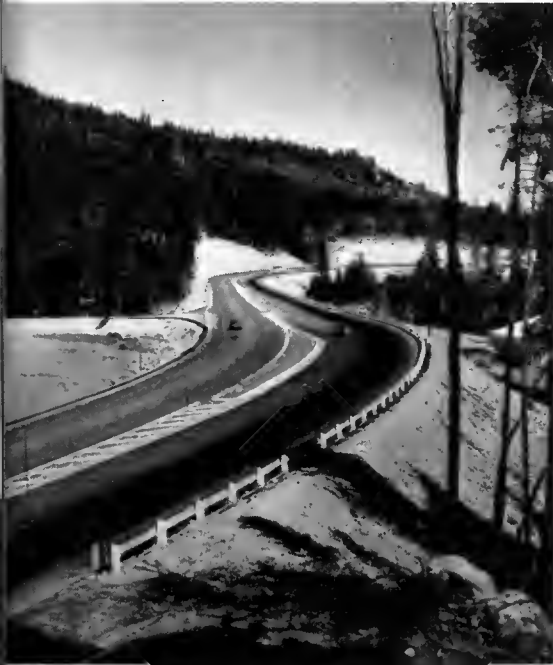
WIN COVER —Recently completed expressway construction on U.S. 99 north of Shasta Lake. The channelized intersection will eventually be replaced with an interchange when this section is developed to a full freeway under the Interstate Program. The large snow markers have been placed for the winter season to guide the snowplow operators. (See Report From District II, page 12.)
