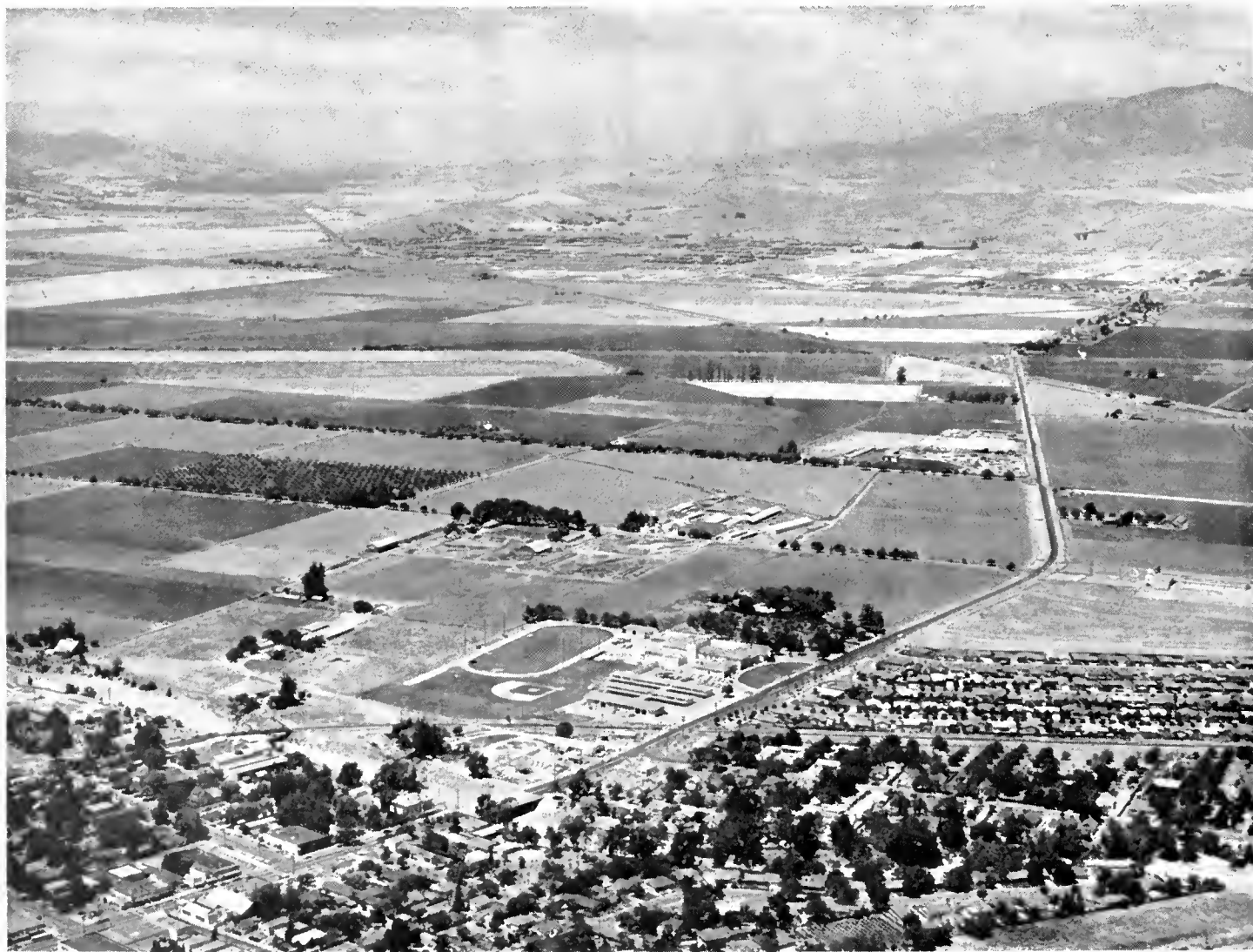
This view northward from Pleasanton shows the reconstructed portion of Santa Rita Road (FAS Route 1019). The new bridge can be seen in the left center foreground.
