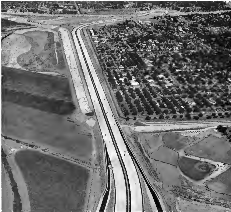
When work is finished on several current and budgeted projects, this recently completed portion of the Ventura Freeway in the San Fernando Valley will be part of 90 miles of continuous full freeway on US Highway 101 from Calobasas, through Los Angeles, to the San Diego County line south of San Clemente.
