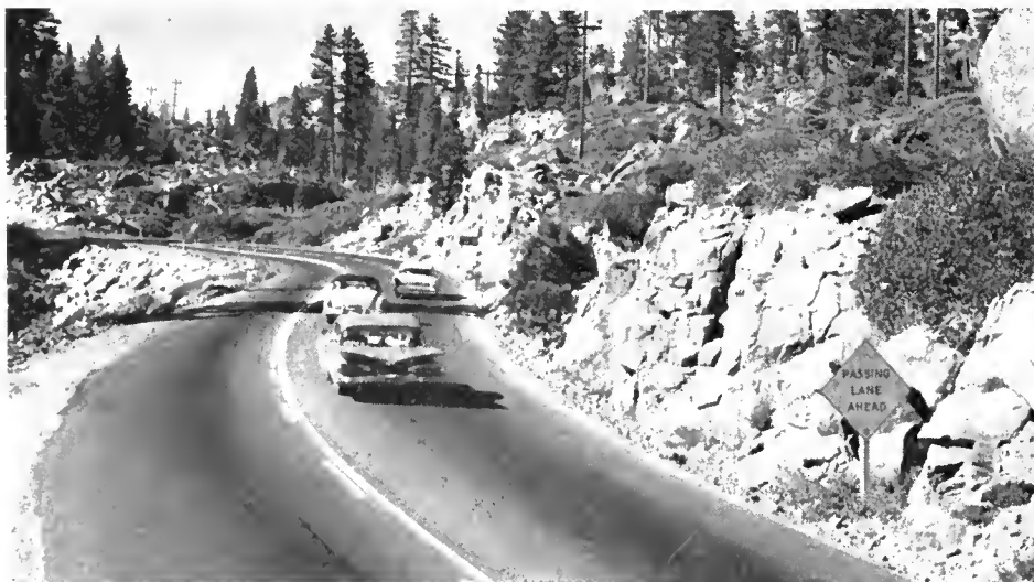
Old road over summit is still only two lanes, but many passing lanes have been provided on up-grades.
