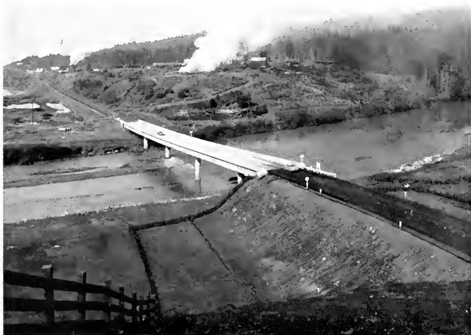
PHOTOS ABOVE AND RIGHT—Two views of the new reinforced concrete box girder bridge across the Gualala River on Sign Route 1.
