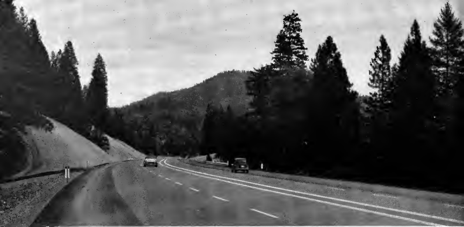
This new section of expressway was recently completed on U. S. 99 in the Sacramento River Canyon in Shasta County. The view is northward toward Pollard Flats.
