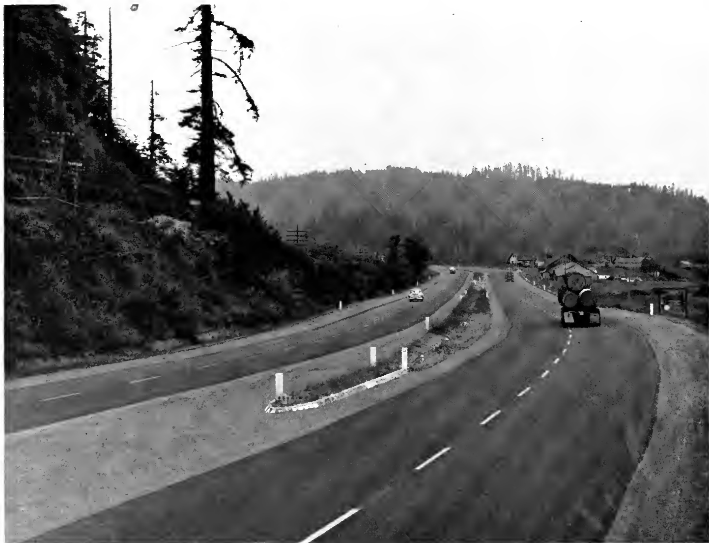
This expressway section on US 101 is between Robinson Ferry Bridge and Alton. It was the first long section of four-lane, divided roadway to be constructed in District I.
