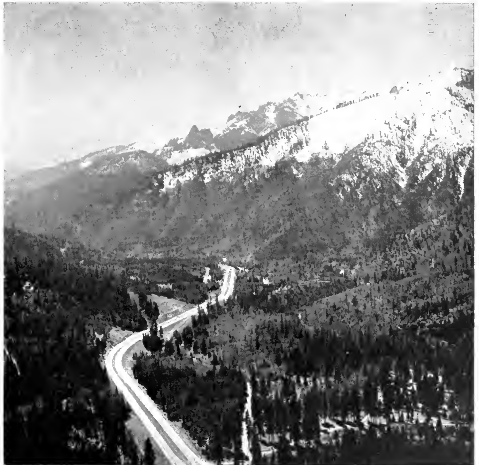
A section of new expressway on US 99 in Siskiyou County. Castle Crags are in the background.
