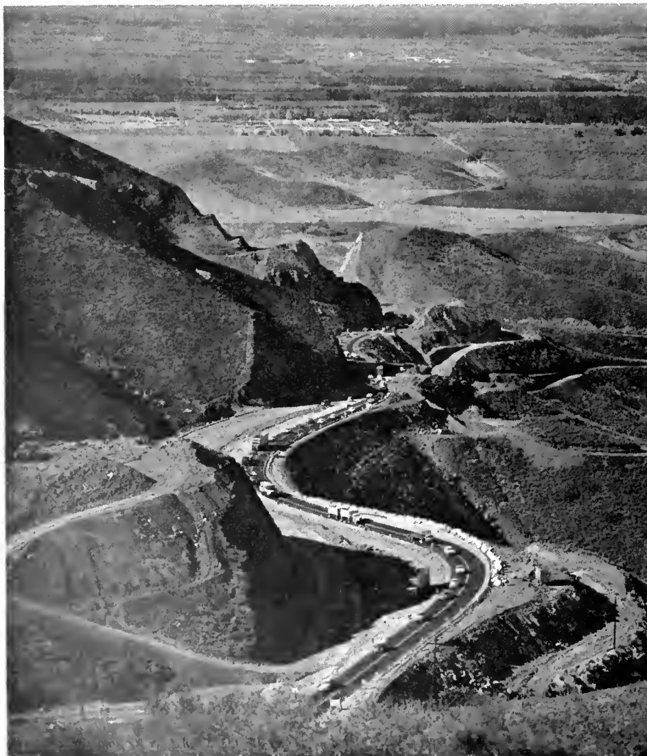
Looking west from the top of Conejo Grade showing construction in progress on the Ventura Freeway. Traffic through the construction area is being handled on a temporary detour.
