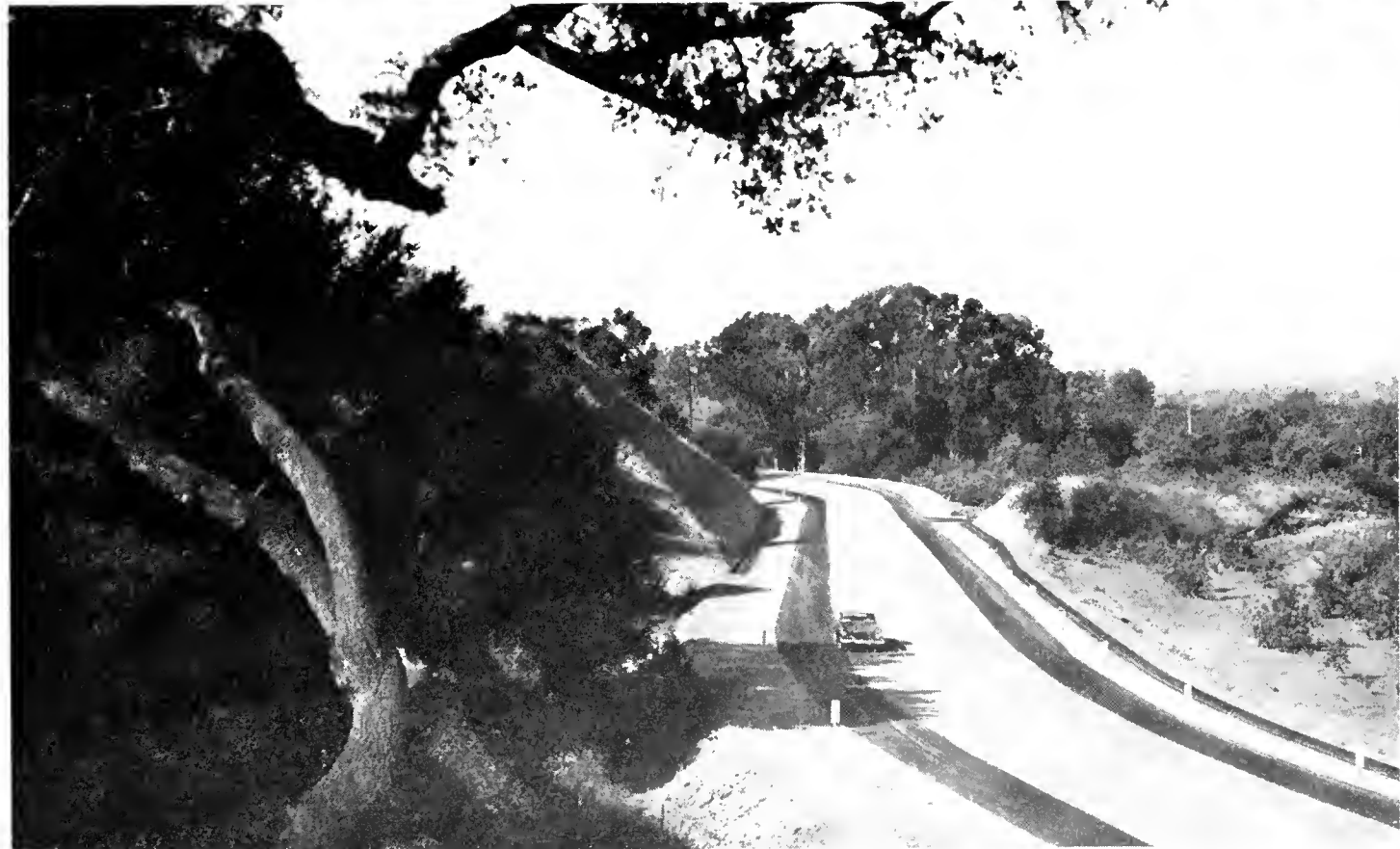
UPPER LEFT—A reconstructed section of Sign Route 41 in northern San Luis Obispo County. UPPER RIGHT—An aerial of the new section of US 101 freeway west of Santa Barbara near Elwood. LOWER—An improved section of Turnpike Road north of US 101 near Santa Barbara.
