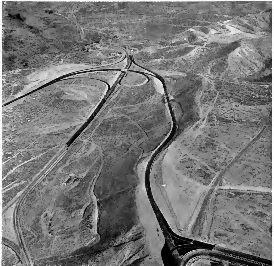
Federal aid secondary county road projects are planned by the county and in most instances constructed with county supervision following review and approval by the Division of Highways. One large-scale 1957 FAS project was this improvement and interchange on the Alfred Harrell Highway near Bakersfield, Kern County.
