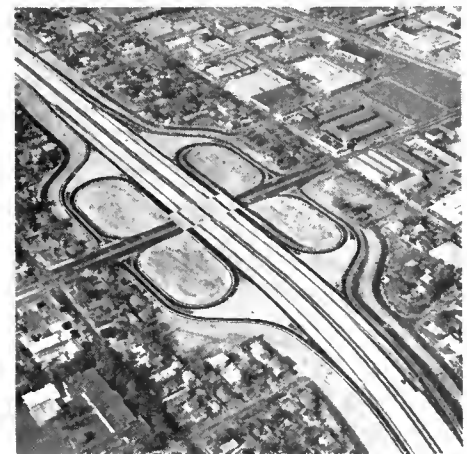
Looking north showing cloverleaf interchange for Golden State Freeway and Western Avenue in Glendale
