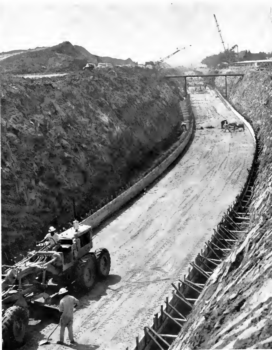
This photo shows the form work in place for the bottom slab of the Burbank-Western Storm Drain Channel.
