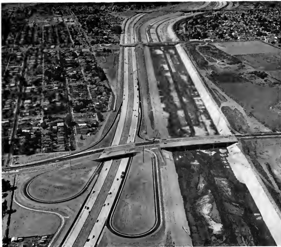
An aerial of the Olive Street Interchange on the Long Beach Freeway. The view is northward.
