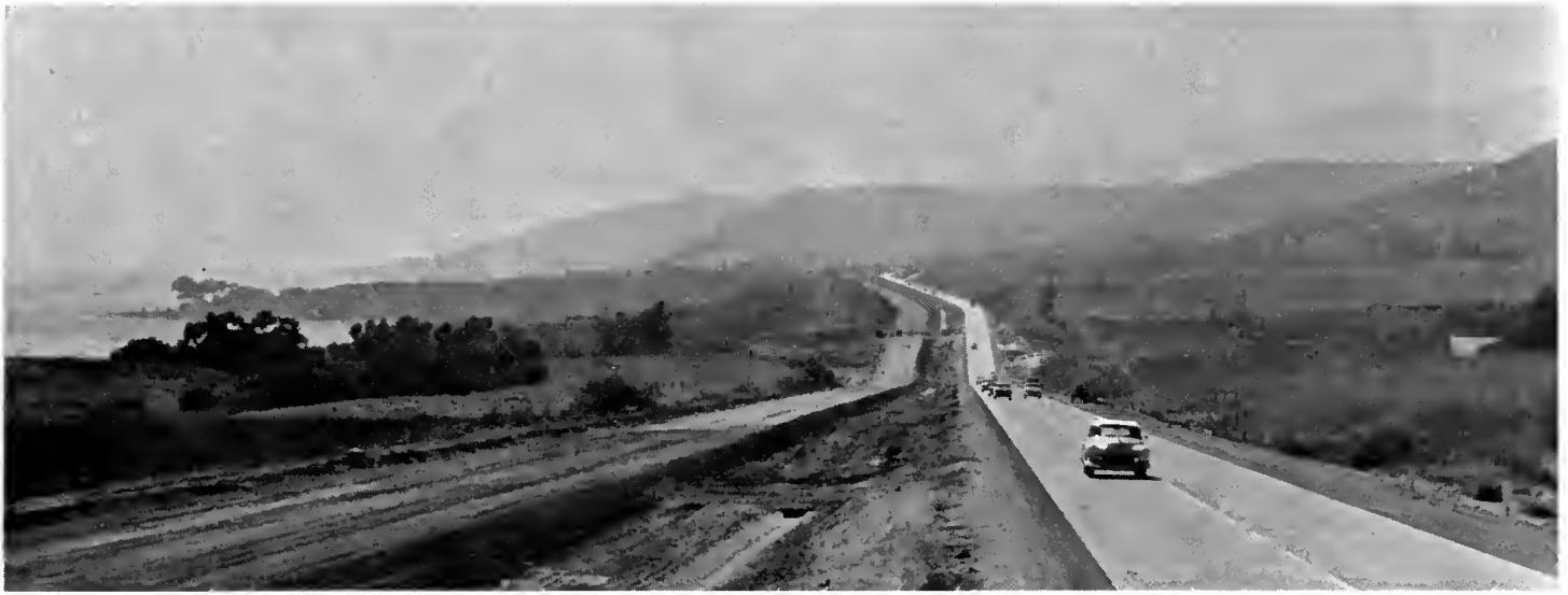
This expressway under construction south of Santa Barbara is another link in the chain of improved sections on US 101. In this photo, the new lanes have been completed and are being used by traffic while the old roadway to the left is being reconstructed to expressway standards.
