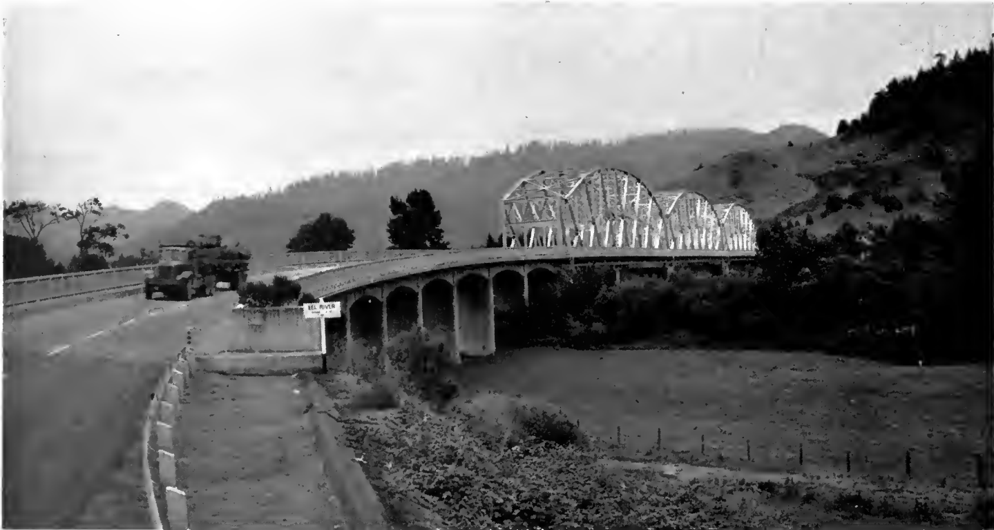
This existing bridge spanning the South Fork of the Eel River at Dyerville will become part of a future interchange. The proposed new structure is rising from the gravel bar right of the limits of this picture to cross the existing road near the left extremity of this picture. US 101 disappears into the Redwoods at the site of the Founder's Tree, tallest tree in the world. The tree cannot be detected because its neighbors are only a few feet short of the record 364 feet.
