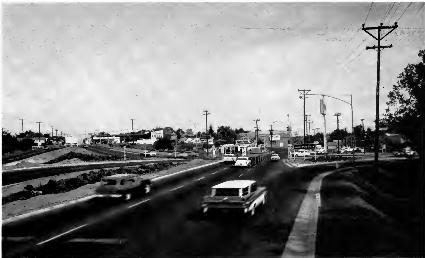
This traffic channelization at the junction of U.S. 99 and State Sign Route 44 in Redding is part of the new one-way street system through the city.
