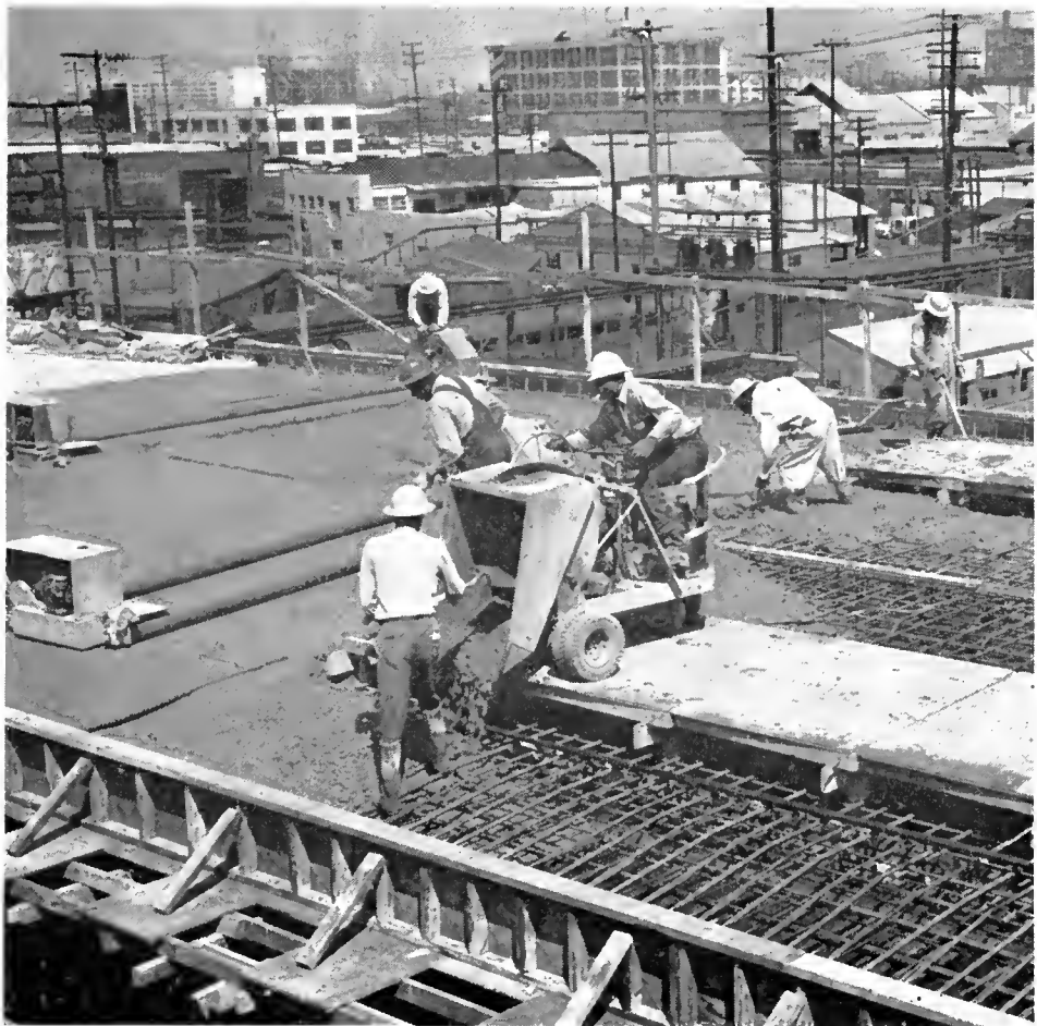
This crew is pouring concrete for the deck of the westbound distributor roadway over the Santa Fe Railway yard.
