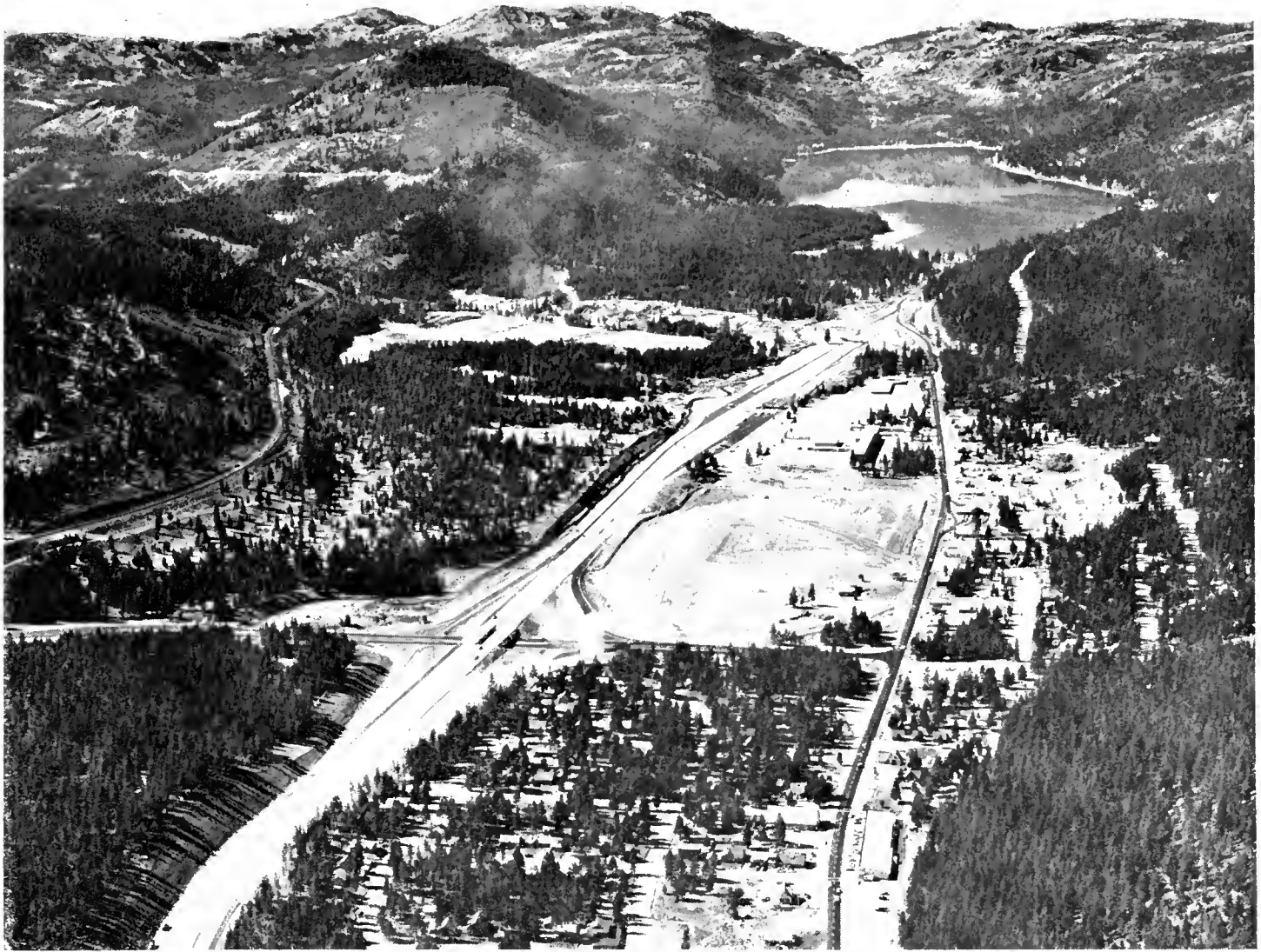
Aerial view of western outskirts of Truckee and US 40-State Sign Route 89 intersection which is turnoff for Squaw Valley. Donner Pass is lowest notch above Danner Lake in background. New alignment will cross summit farther to right. Site of new plant inspection station is just above right center.
