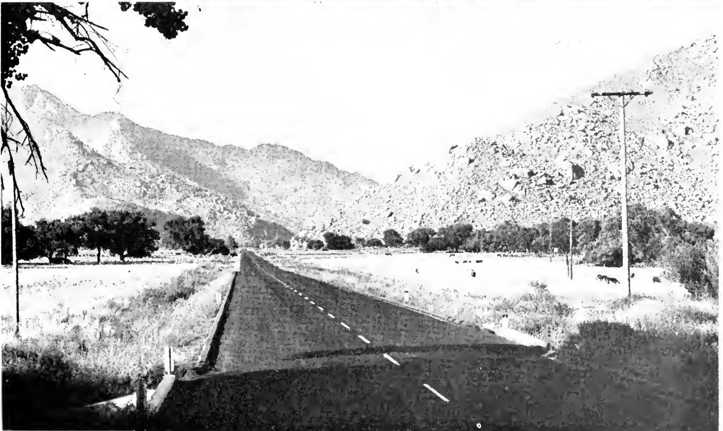
UPPER--The recently improved junction of US 466, on the left, and US 6 at the north edge of Mojave. LOWER--A view eastward of the Walker Pass Road (Sign Route 178) near Weldon. The old highway curved along the base of the hills to the left.
