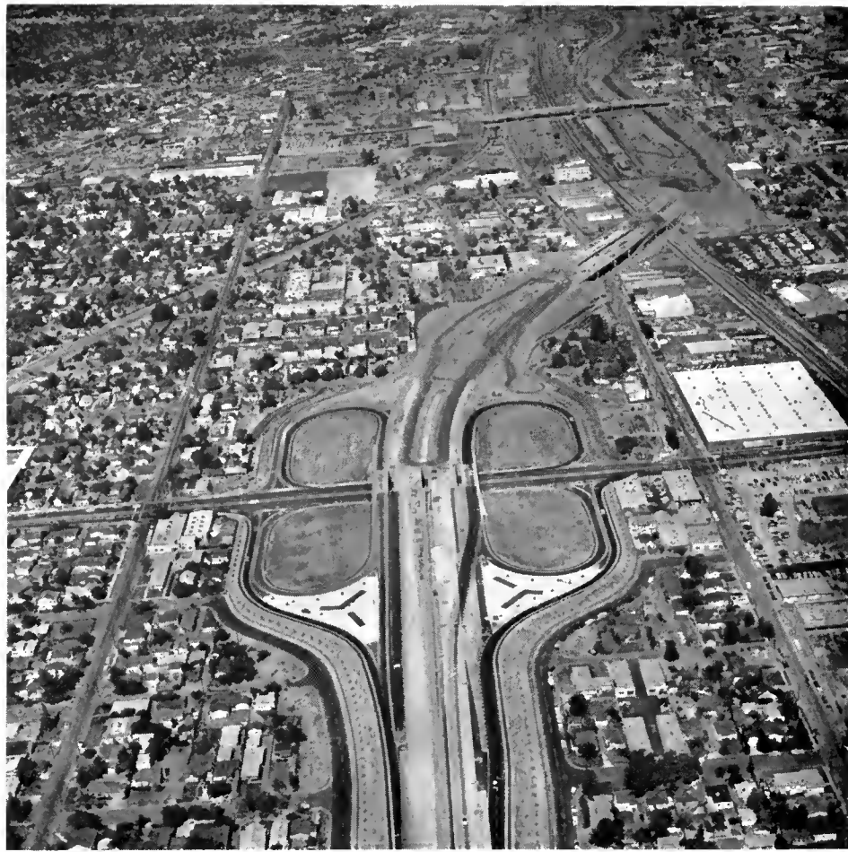
Looking north along a section of the Golden State Freeway showing construction through the City of Burbank. The cloverleaf in the foreground is the Alameda Avenue interchange.
