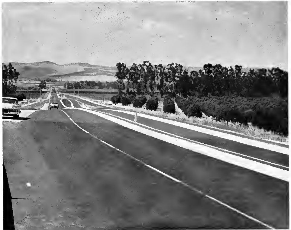
Looking west along Laguna Canyon Road showing a considerable portion of the two miles of new roadway.
