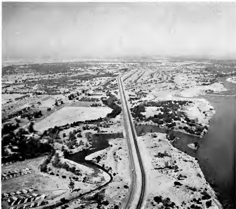
This view eastward shows the four-lane interim improvement on US 50 between Sacramento and Alder Creek. Nimbus Dam and Reservoir is to the right.
