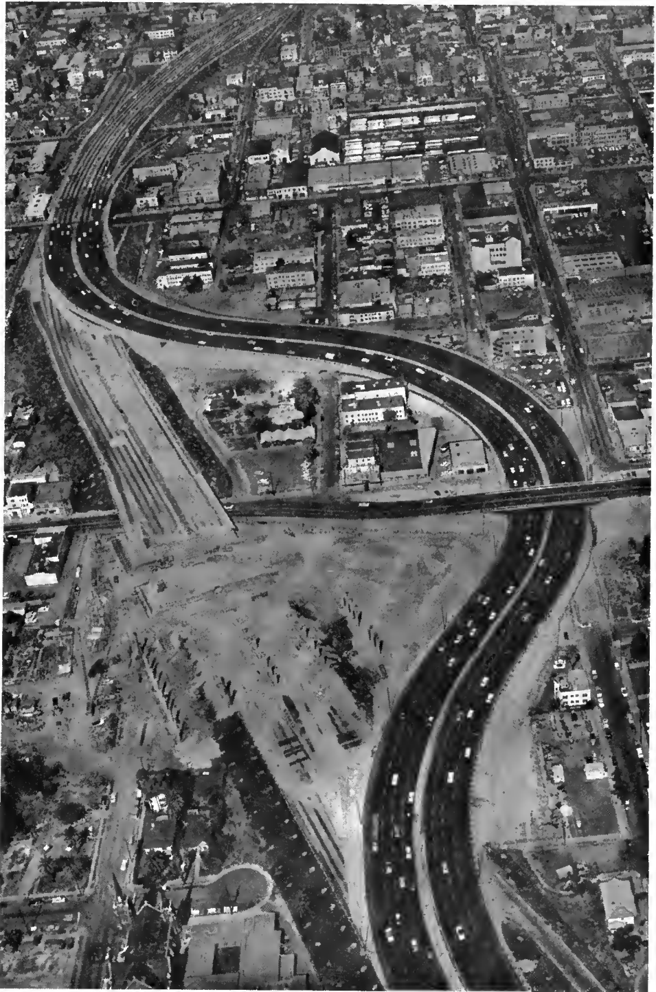
This view northward shows the Harbor Freeway detour around construction of the Santa Monica Freeway separation. Venice Boulevard (left to right) passes under the construction zone and over the detour.
