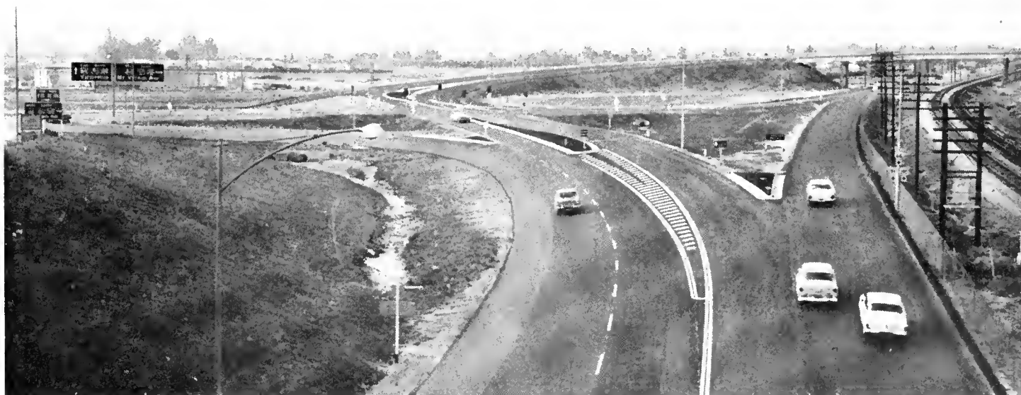
UPPER—A view of the Victorville-Borstow Freeway and some of the rolling desert country through which it passes. LOWER—This interchange connects Highland Avenue (Sign Route 30) with US 66-91-395 in the City of San Bernardino.
