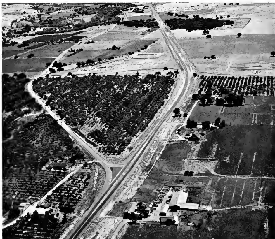
An aerial view eastward on Sign Route 120 in Stanislaus County showing relocation of the highway at Jones Curve, east of Oakdale. The old highway is to the left.
