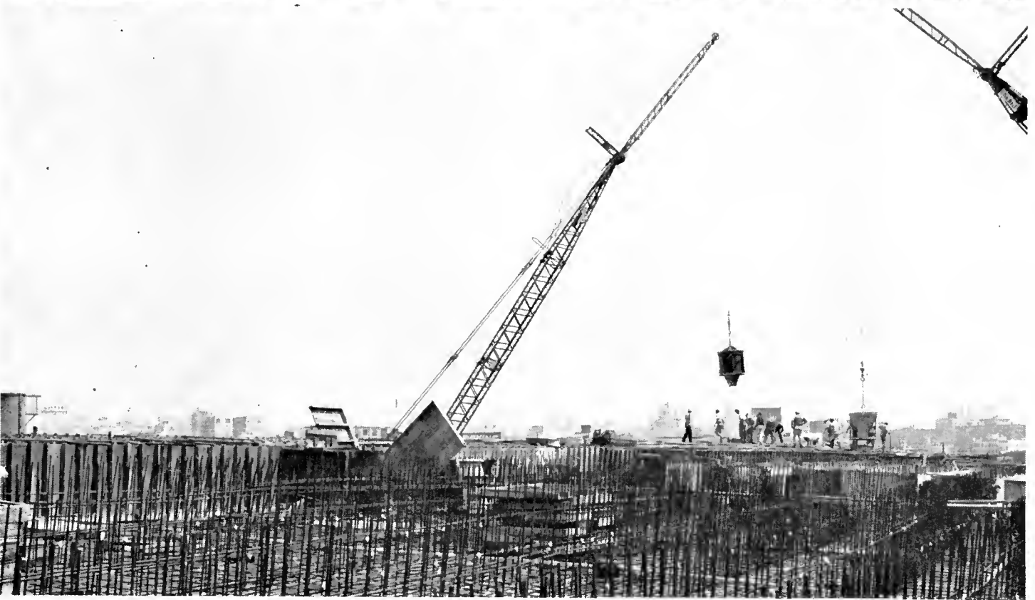
UPPER—Workers pour concrete on the third level of the new Santa Monica Freeway Separation. LOWER—Hundreds of reinforcing steel bars serve as a foreground to concrete pouring operations beyond.
