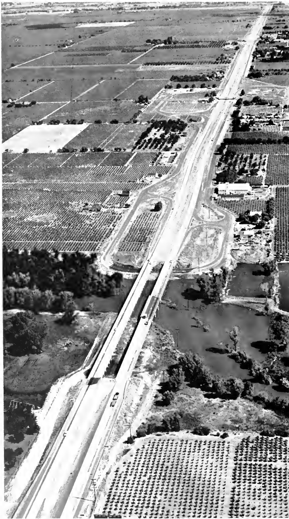
An aerial view of US 99 in Son Joaquin County showing the twin spans across the Mokelumne River with frontage road passing under the north end of the bridges
