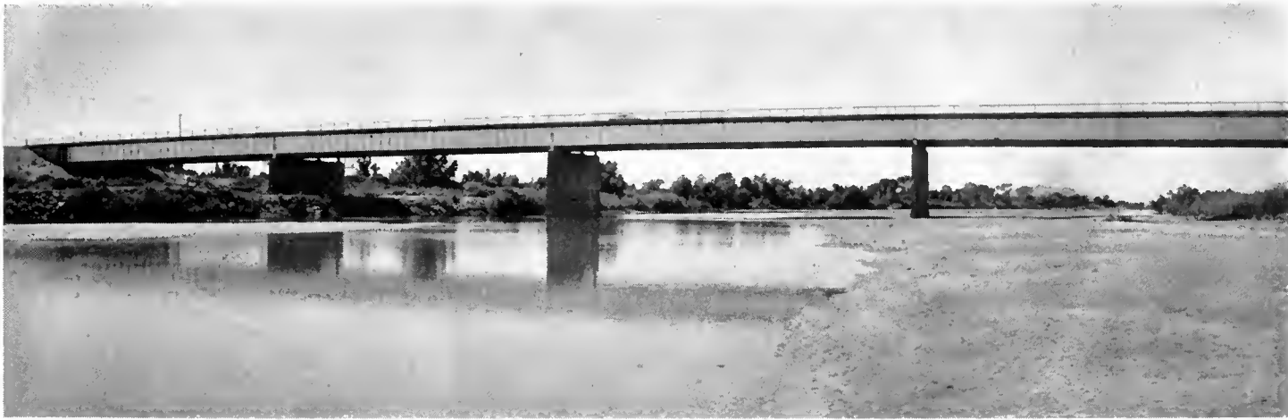
This bridge carries US 80 across the Colorado River between Winterhaven in Imperial County and Yuma, Arizona
