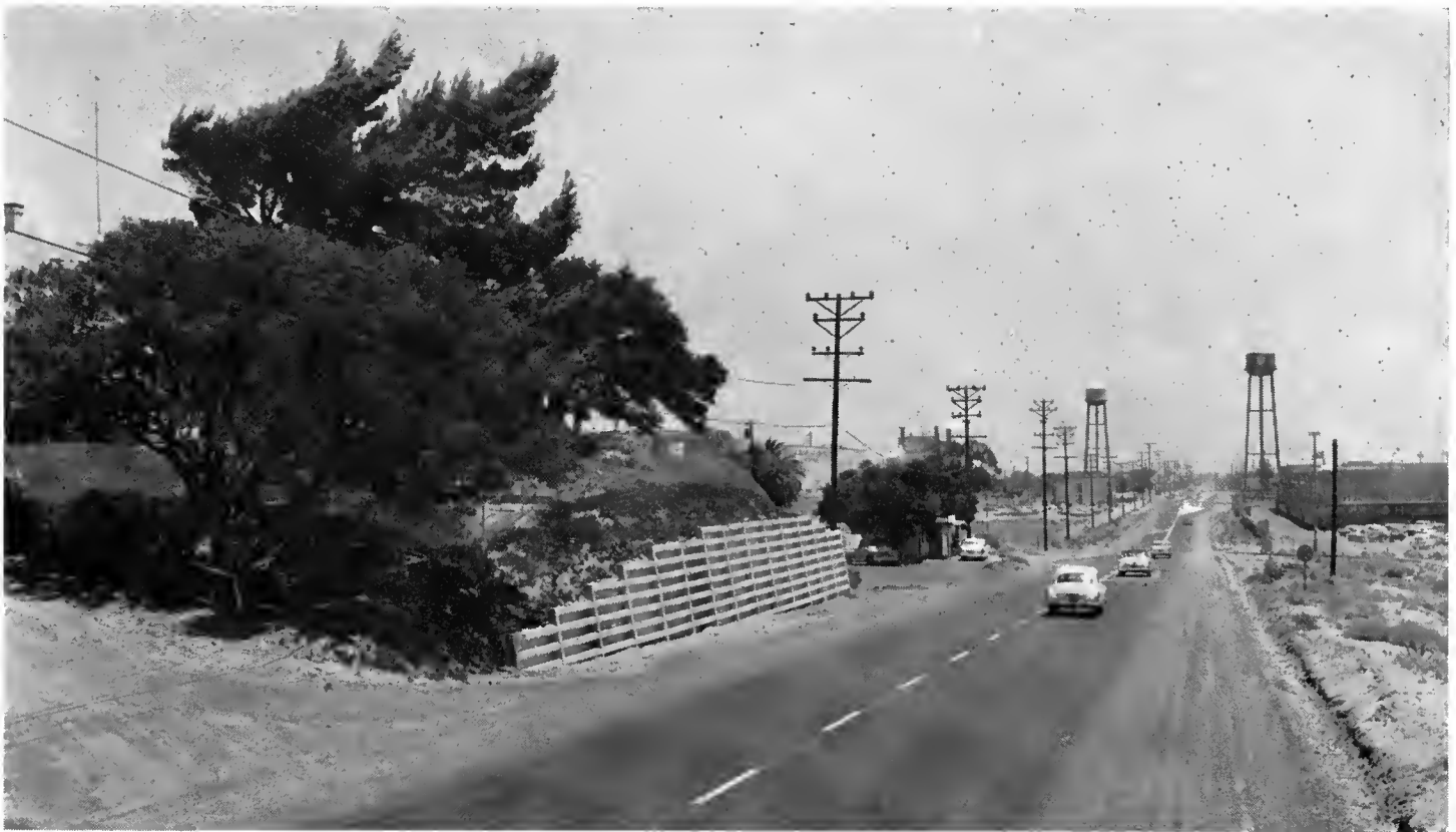
This is a portion of Wilbur Avenue, an industrial highway east of Antioch, recently improved by Contra Costa County under its road bond and federal-aid secondary program.
