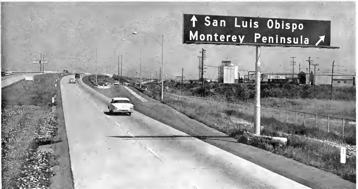
The Salinas Bypass on US 101 in Monterey County. As the directional sign indicates, the interchange ahead connects US 101 with State Route 117 to the Monterey Peninsula.
