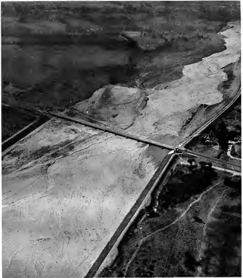
An aerial of the recently constructed channel for the Santa Ana River and the Crestmore Bridge located northwest of the City of Riverside
