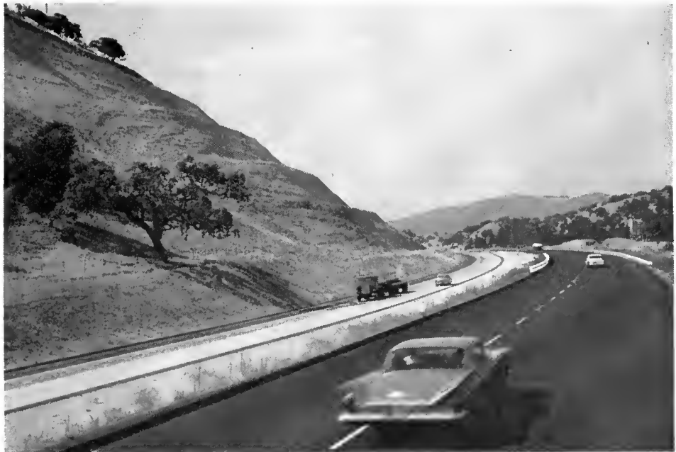
A section of new US 101 freeway between the northern outskirts of Buellton and the Sign Route 150 intersection.
