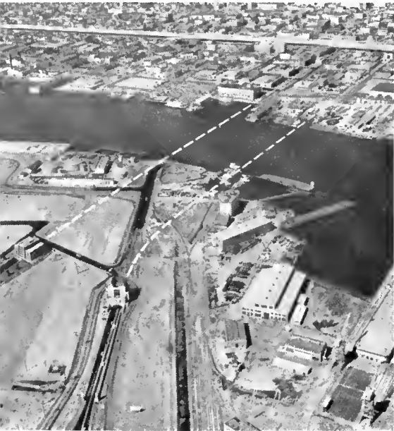
Location of the existing Posey Tube in the photo above is shown by the dotted white line on the right; the dotted line on the left indicates the location of the future Webster Street tunnel.
