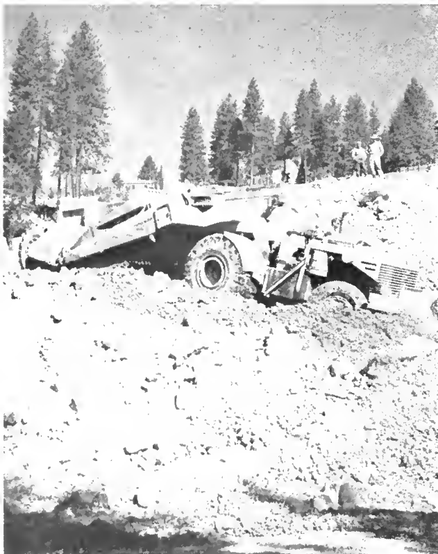
Self-propelled scrapers and bulldozers cutting stabilization trenches near Alta.
