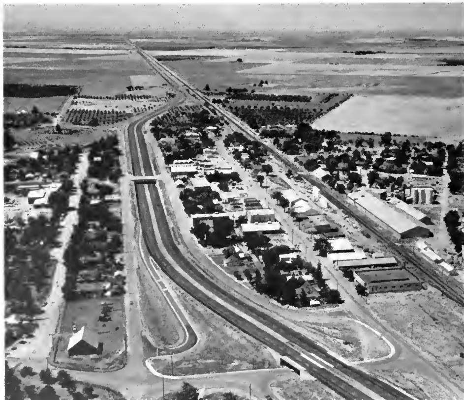
An aerial view of the freeway through the Town of Arbutle on US 99W. The separation structure in the center of the picture is the Hall Street Overcrossing.
