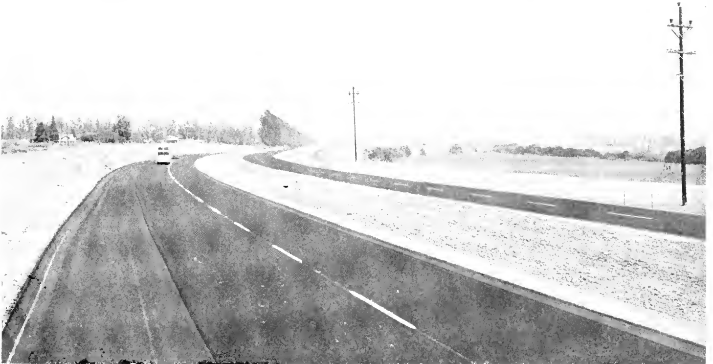
UPPER—Completion of this new expressway between Greenfield and King City on US 101 in Monterey County has eliminated the congestion caused in the past by heavy local agricultural truck traffic. LOWER—Another scene on the new expressway between Greenfield and King City. The roadway follows the Salinas River (right).
