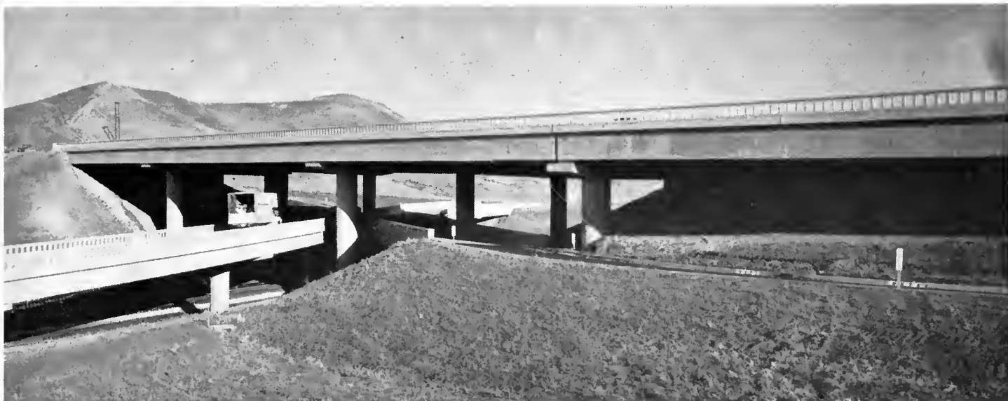
The three-level interchange near Hercules where two freeways meet. Top level is US 40; bottom level is the Arnold Industrial Freeway; middle level is for on ramps to US 40.
