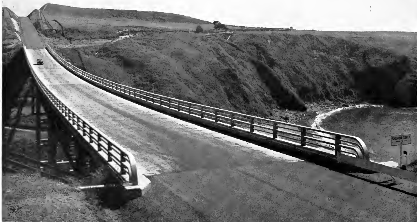
Old bridges on Sign Route 1 on the Mendocino coast have been replaced by modern structures such as this one across Salmon Creek
