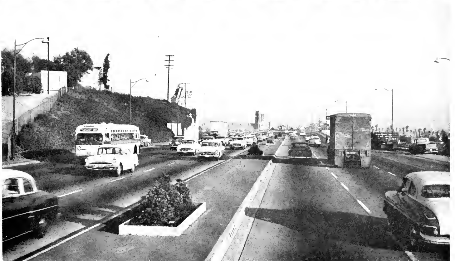
UPPER—The effectiveness of various median designs was evaluated in a recent Division of Highways safety study. Medians with barriers, such as this one on the James Lick Freeway in San Francisco, were among those classified as nontraversable. LOWER—This type of curbed center strip on the Hollywood Freeway in Los Angeles was one of the deterring median designs included in a recent Division of Highways freeway safety study.
