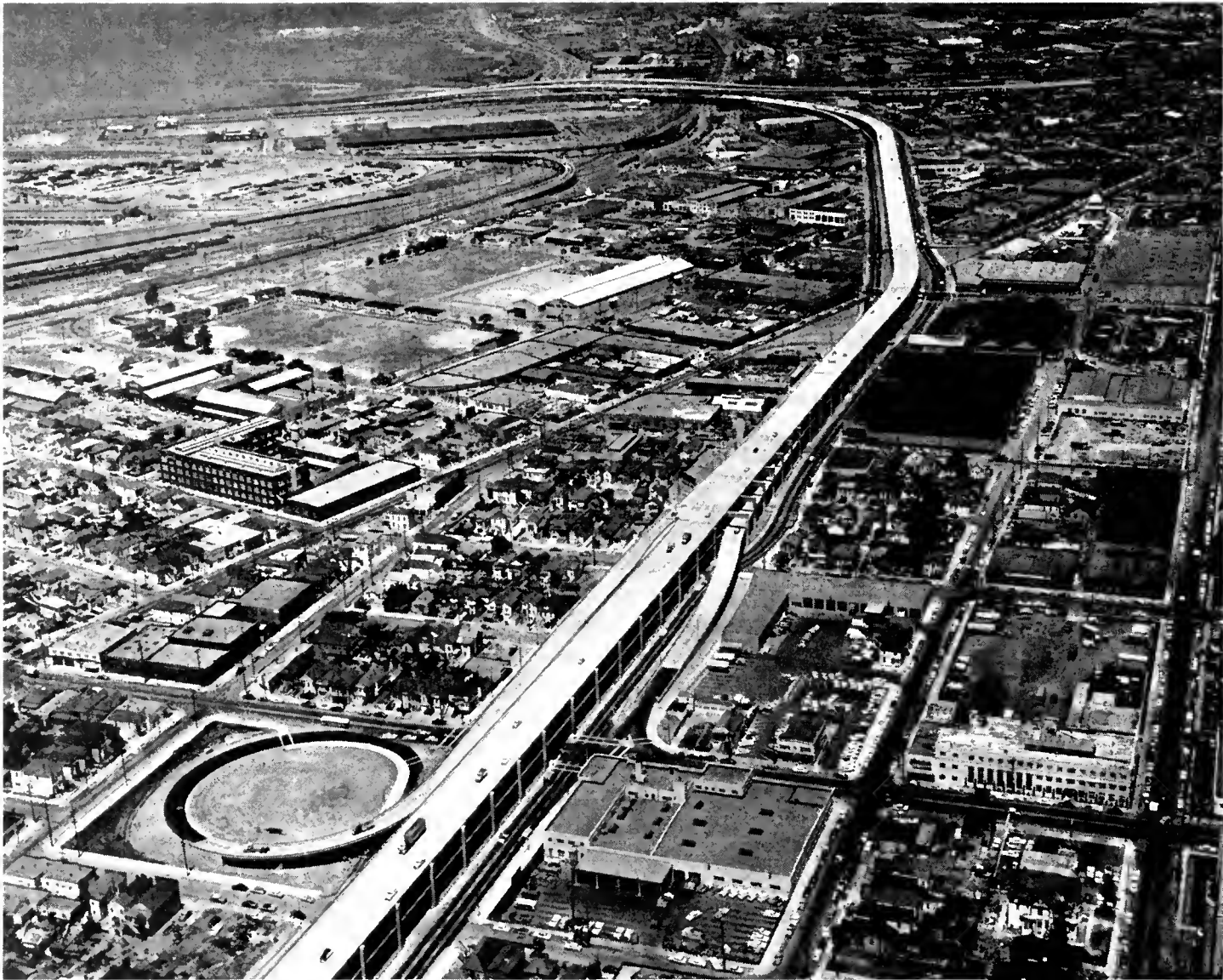
The double-deck Cypress Street structure on the Eastshore Freeway in Oakland. The southbound off-ramp to 14th Street is at the lower left.
