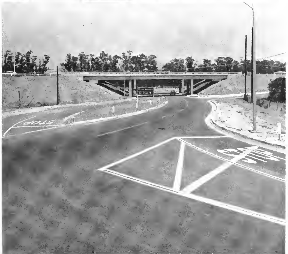
UPPER—A view southeast from Jeffrey Road toward the Town of Irvine along the newly completed section of the Santa Ana Freeway. LOWER—The Culver Road undercrossing the new freeway. Culver Road connects with the county highway leading to the main entrance of the El Tara Marine Air Station.
