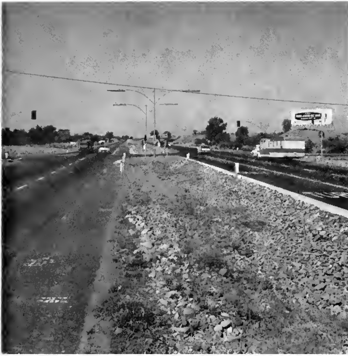
Improvement of intersections is an important part of the district construction program. Typical of these are (left) the Nimbus Intersection, an interim improvement east of Sacramento on US 50 which will eventually be replaced by a full freeway interchange and (right) the Latrobe Road intersection, also an US 50, where part of a hill was removed near the highway to give better sight distance to motorists.
