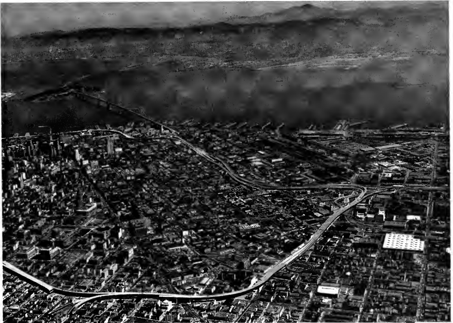
A new 1.4-mile section of the Central Freeway in San Francisco between South Van Ness Avenue and Turk Street, including an overcrossing of Market Street (foreground), opened April 22d. The Embarcadero Freeway and San Francisco-Oakland Bay Bridge may be seen in the background.
