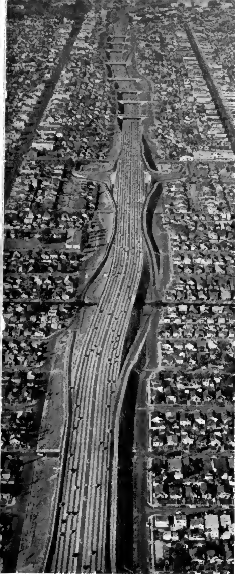
Aerial photo looking north along a completed section of the Harbor Freeway from above Manchester Avenue
