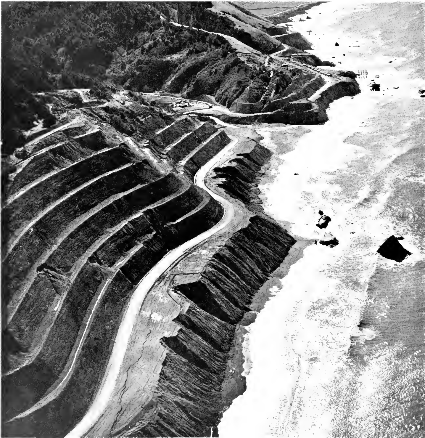
This aerial view of State Sign Route 1 in Mendocino County shows the giant cuts made in the Juon Creek Bluffs as part of the reconstruction of the highway by the county under the Federal-aid Secondary Highway Program
