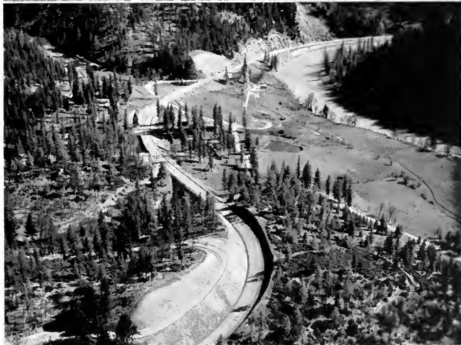
UPPER—Adin Summit on US 299 in Modoc County. Note the damage to the sign which has evidently served as a rifle target for vandals. LOWER—New construction on US 299 in Trinity County with the Trinity River on the right and the old highway on the left.
