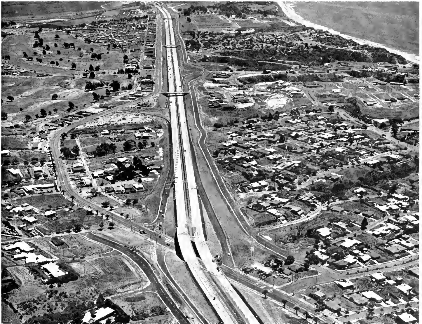
Looking south along the new freeway through San Clemente. The north connection with present US 101, which passes under the freeway, can be seen in the foreground.
