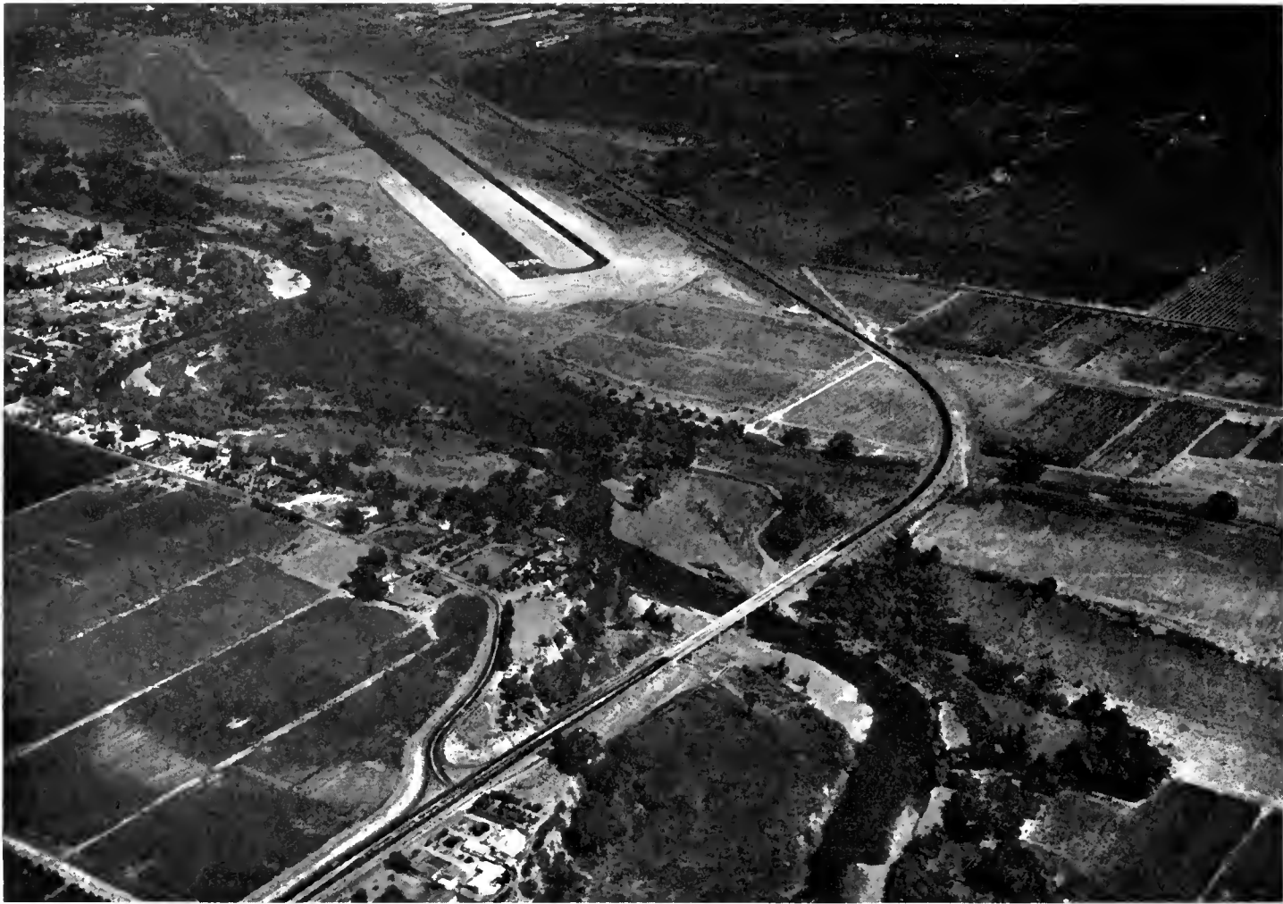
A view of East Modesto Road (FAS Route 1226) looking in the opposite direction of the photo on the previous page showing the bridge across the Stonislaus River and the City of Modesto in the distance
