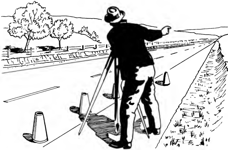
Members of survey parties working on any portion of a highway wear a red shirt, pancha, vest or coat. These may be luminous or standard cloth.
