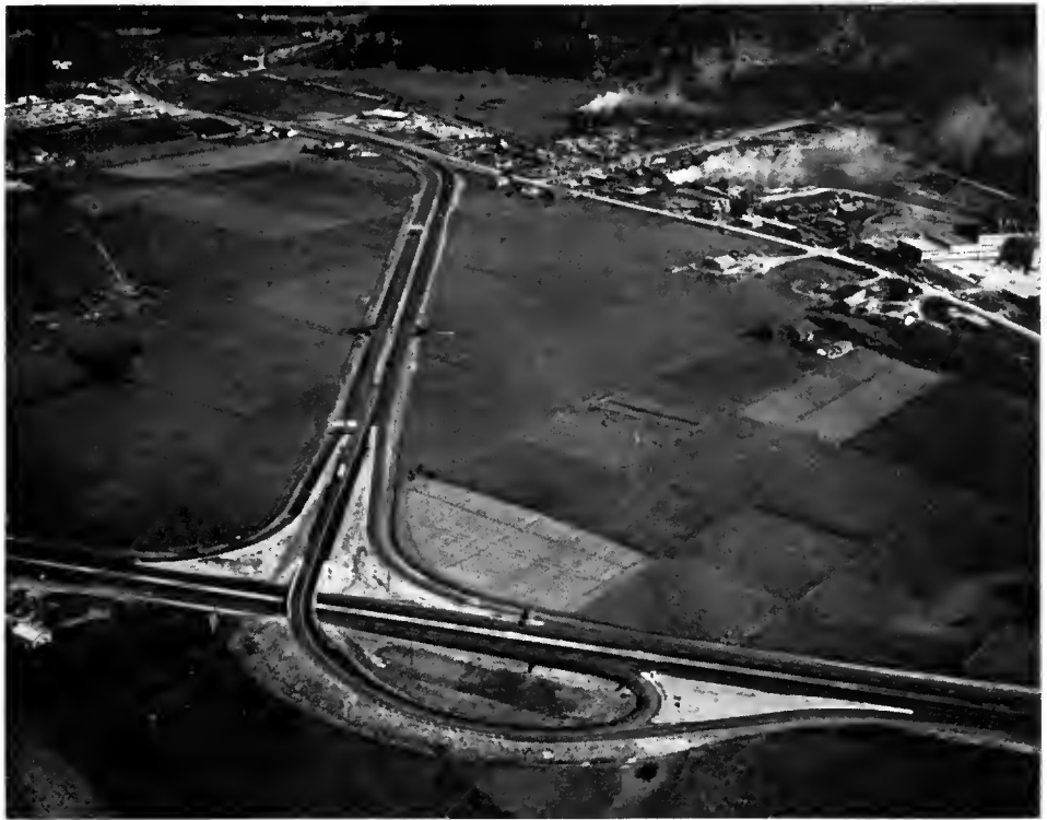
Reconstruction of US 101 north of Arcata resulted in a new trumpet-type interchange connecting US 101 and US 299. This aerial is looking eastward along US 299.
