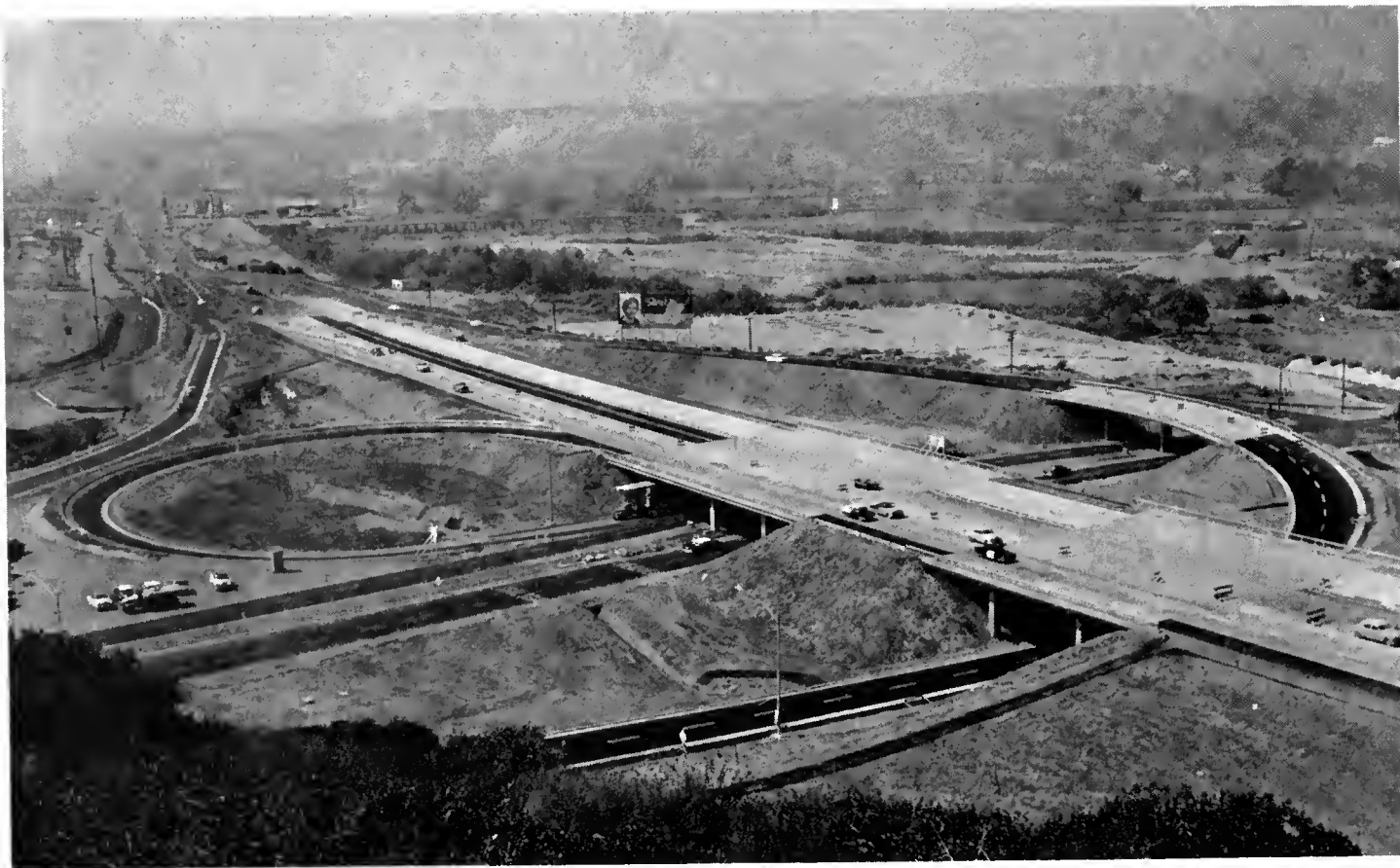
This pattern of bridges and ramps is the new US 80-Fairmont Avenue traffic interchange just east of San Diego
