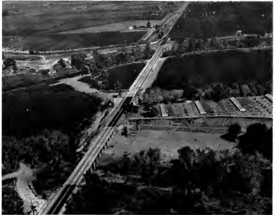
A northerly view of County F. A. S. and Flood Relief Project on F. A. S. Route 903 between Modesta and Escalan (in the distance). The old flood-damaged bridge and trestle occupied the diagonal bare area on the left.
