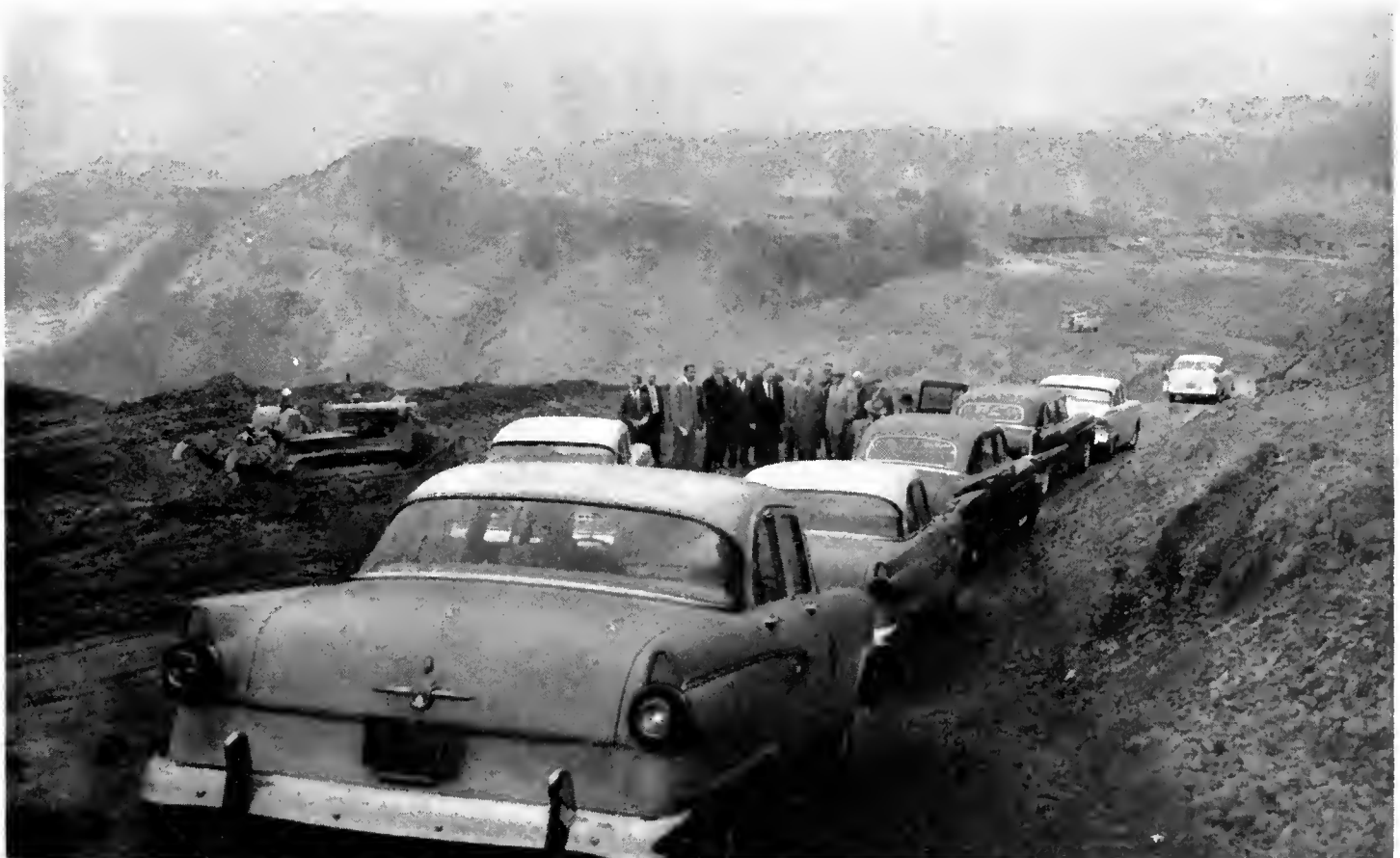
Governor's party halts on contractor's haul road to inspect work. The road is normally traveled by heavy equipment used in construction of the Ventura Freeway-San Diego Freeway interchange.
