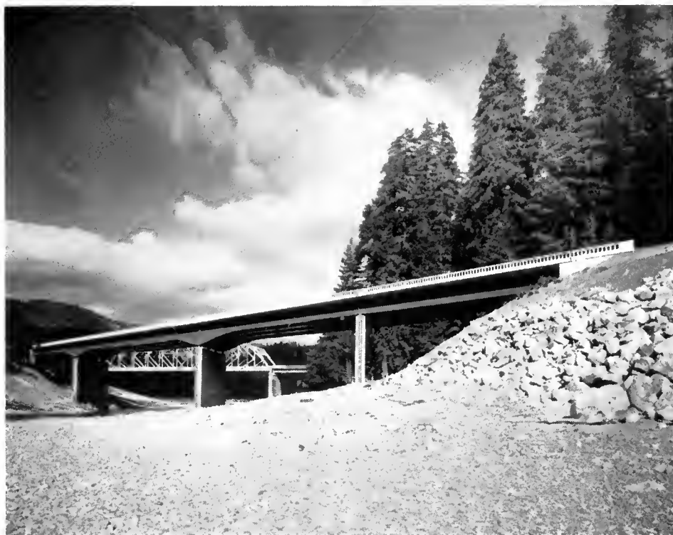
Winner of the first honorable mention award in the Class II Division for Bridges with spans less than 400 feet long and costing more than $500,000, was this structure across the South Fork of the Eel River on US 101 near Dyerville in Humboldt County. (Aerial view on page 33.)
