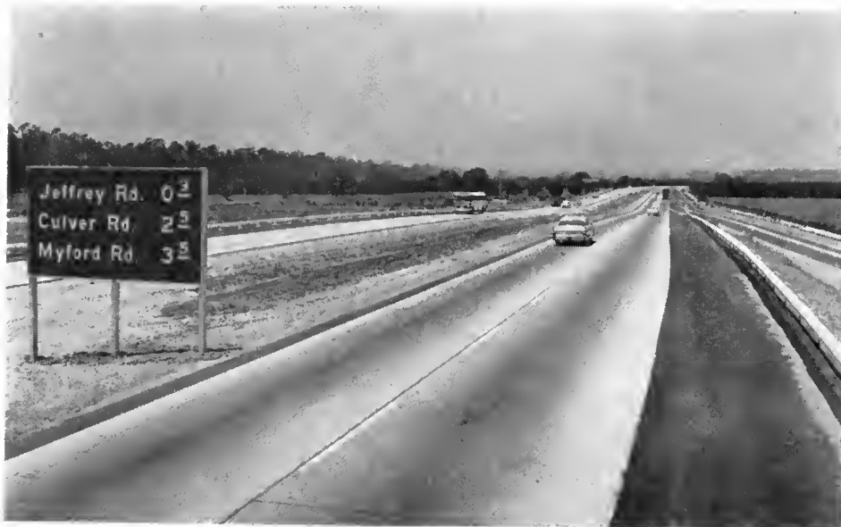
Signing along the new freeway. Motorists are alerted to forthcoming separation structures where they may want to leave the freeway.
