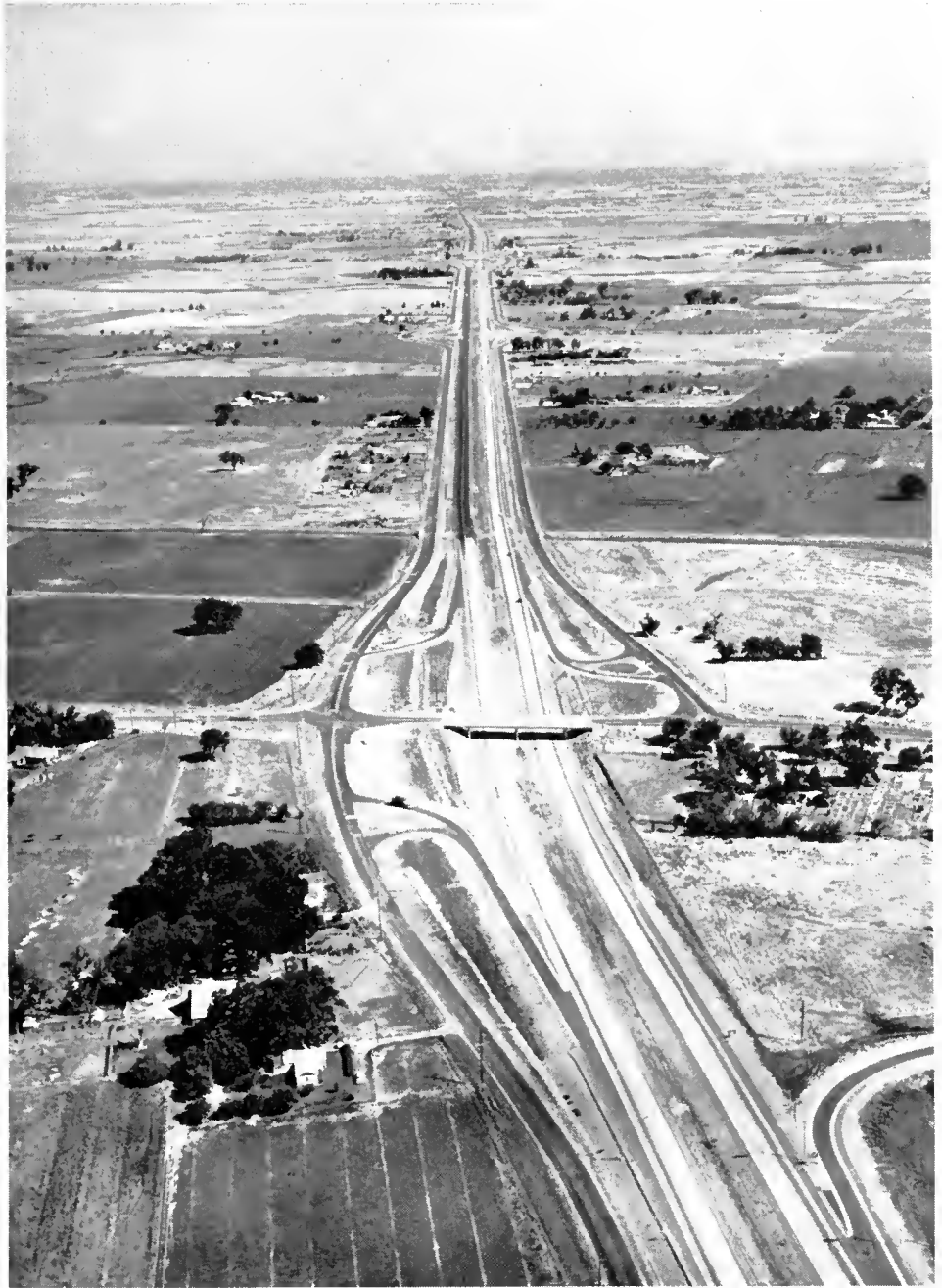
This section of freeway on US 99-50 south of Sacramento will be completed this summer. The Elk Grove Road Interchange is in the foreground; the City of Sacramento on the horizon.
