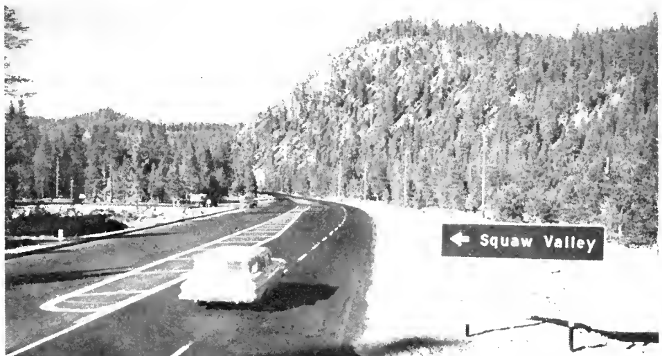
Recently rebuilt State Sign Route 89, looking northward at channelized intersection for Squaw Valley turnoff.
