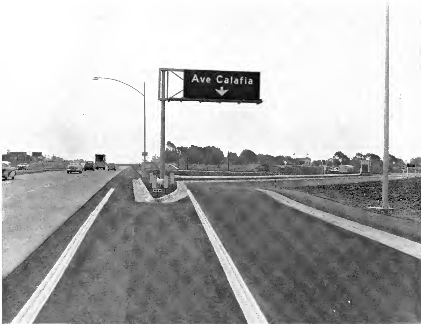
Pictured here is a cantilever type sign structure. This type of sign reaches maximum proportions of 10 feet by 30 feet.
