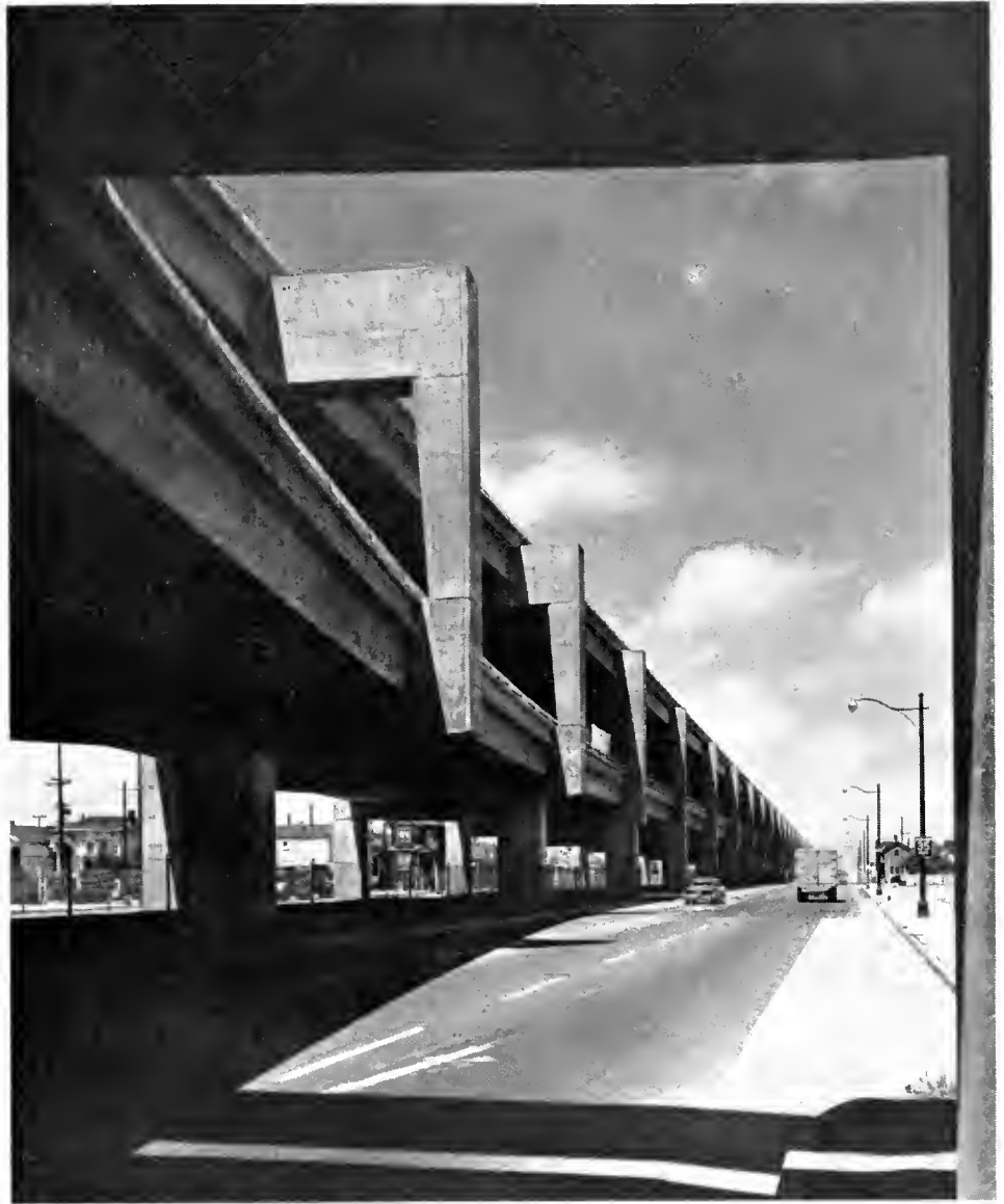
The double-deck Cypress Street traffic viaduct on the Eastshore Freeway through Oakland. Note the local service roads on each side.
