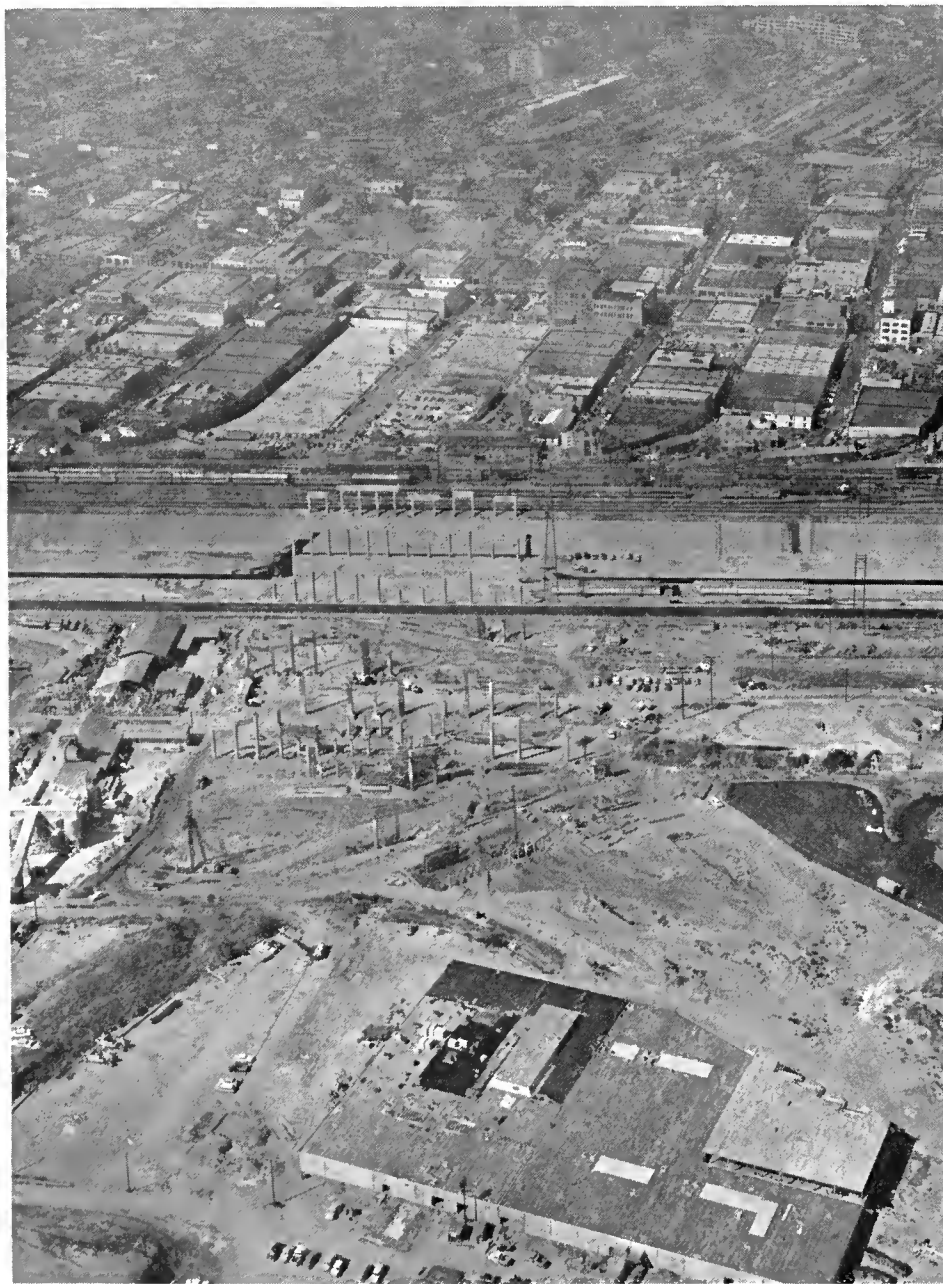
This view of the construction area was taken just after the erection of the reinforced concrete columns which will support the six parallel bridges over the river.
