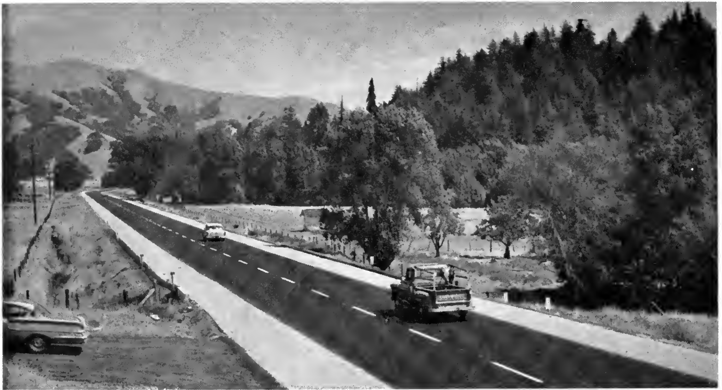
New alignment of Marin County's Sir Francis Drake Boulevard between Lagunitas School and 2.7 miles easterly recently completed under the Federal-aid Secondary Highway Program
