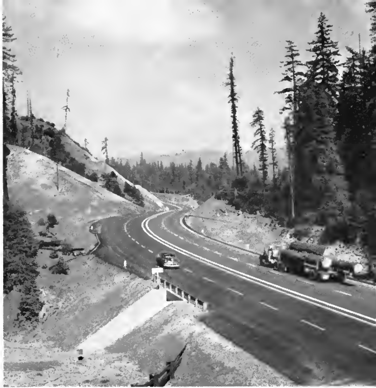
A portion of the completed first unit of the Redwood Parks Freeway on U. S. Highway 101 north of Dyerville at High Rock Road Undercrossing.
