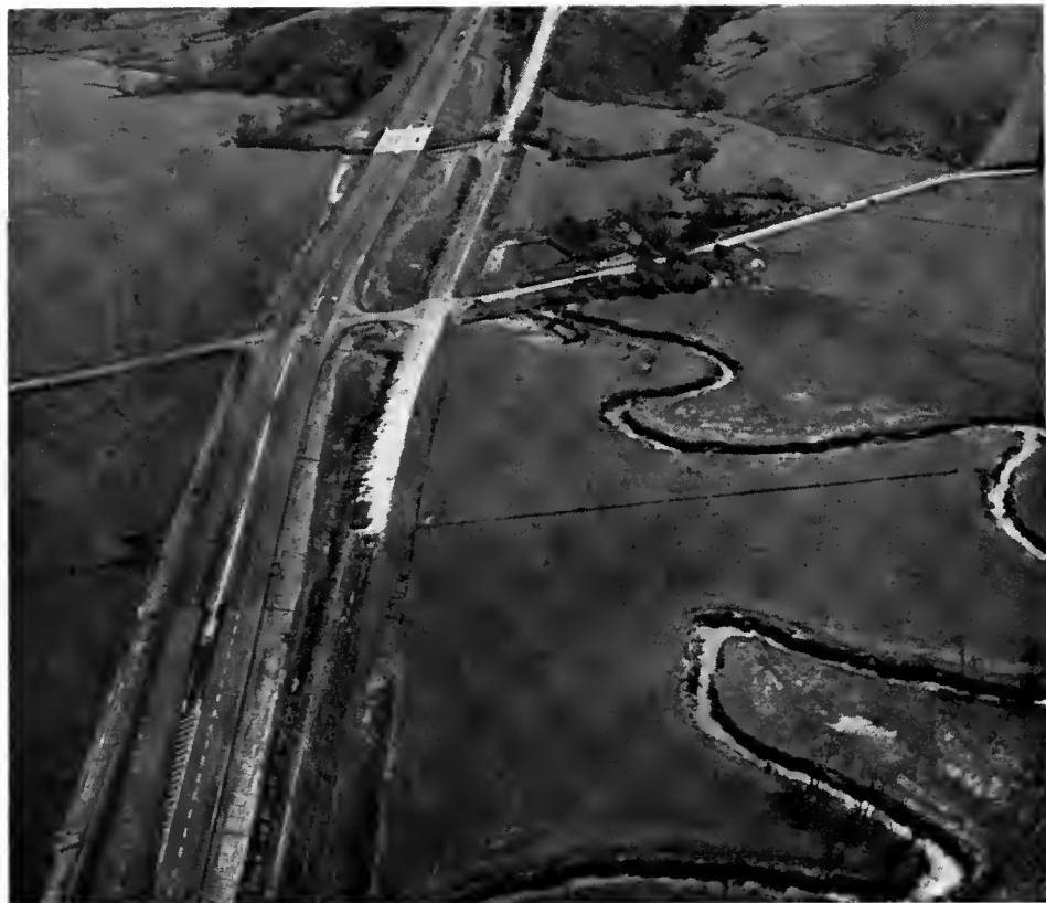
An aerial view taken at the north end of the Loleta Bypass. The road extending southward to the right of the new freeway is the old highway.
