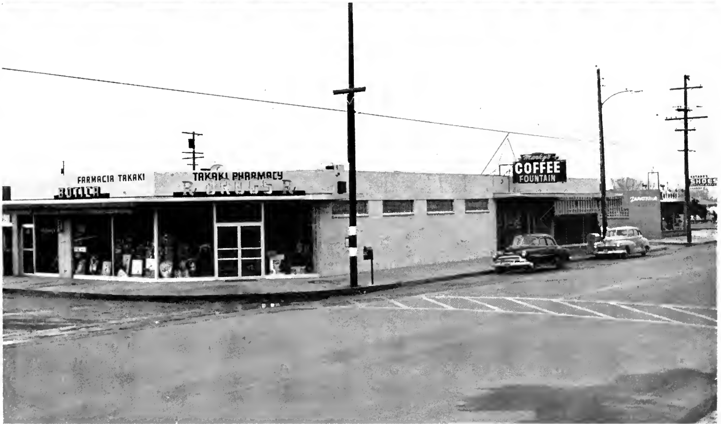
Representative of the significant commercial building activity which has taken place in West Delono since freeway construction was started in 1954 are the new supermarkets (upper) and the new block of stores (lower) located on opposite corners of an intersection near the freeway.
