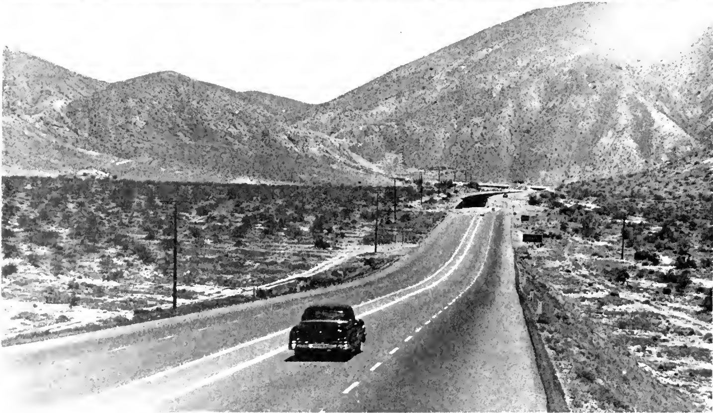
UPPER Looking west along Pole Line Road near the Nevada state line. This route connects US 395, which follows the base of the Sierra Nevada seen in the distance, with the Naval Depot at Hawthorne. LOWER This recently completed portion of US 6 north of Mojave is typical of the divided, four-lane pavements used for new expressways in District IX. Visible ahead is a continuation of this section now under construction through Red Rock Canyon.
