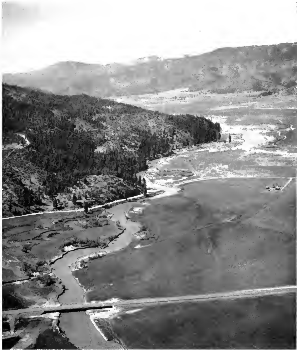
The new highway and bridge on State Route 82 north of Fort Jones in Siskiyou County. The bridge on the old route across the Scott River (center) was washed out during the winter floods of 1955-56.
