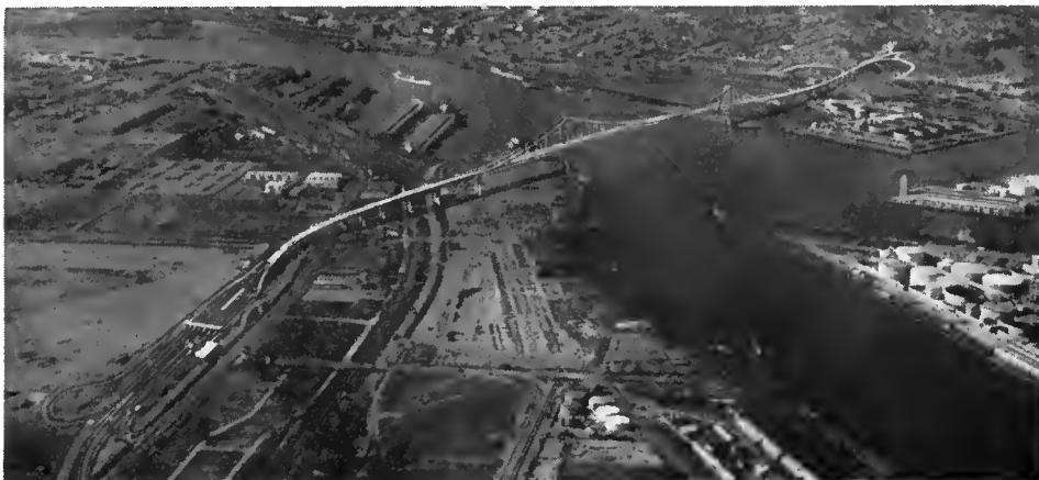
Artists of the Division of Highways have prepared this drawing to show how the new Terminal Island Bridge will appear after it is completed. It will form part of a link connecting the Long Beach and Harbor Freeways.
