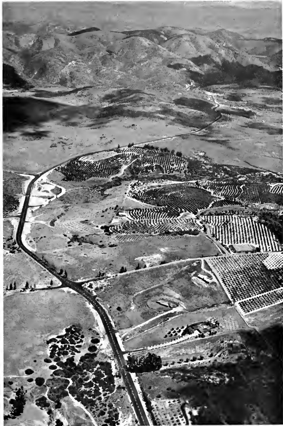
Improvement of the Del Dios Highway (shown here) was a co-operative federal-state-San Diego County project. This aerial view looking northeastward was taken near the west end of the project and shows the Rancho Santa Fe area in the foreground and the Lake Hodges Dam in the background.
