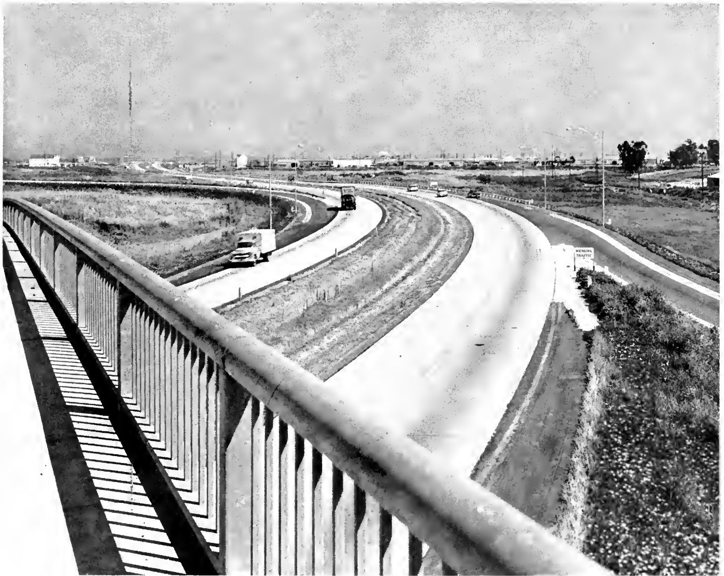
A view southward of the Salinas Bypass from the John Street overcrossing showing industrial development in the zoned area to the right
