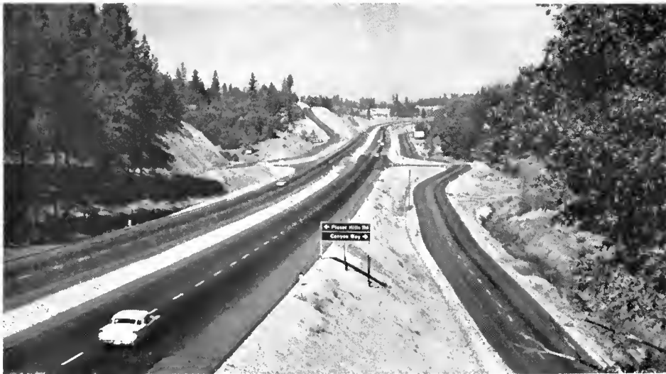
Section of expressway in vicinity of Auburn.
