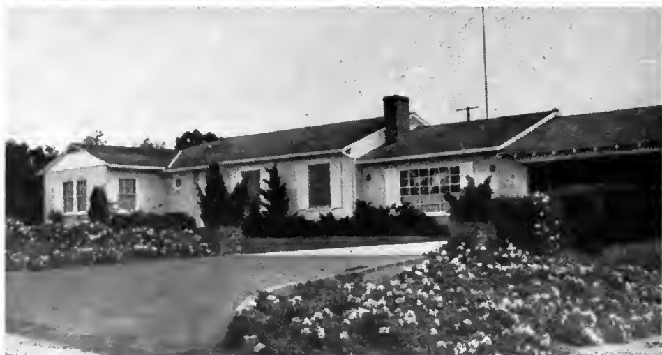
UPPER—This modern residence, purchased by the State in 1950, supported an assessed value of $2,170. Its market value at the time of acquisition was $19,750. LOWER—The same residence after sale at public auction and relocation upon another site. Assessed value 1953, $4,610. Note characteristic "upgrading" changes completed even on this relatively modern improvement, i.e., the family room addition where the garage was formerly located.
