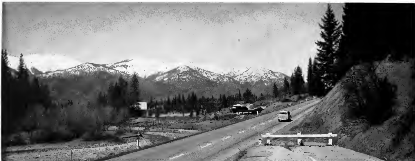
An improved section of US 299 east of Weaverville in Trinity County. A section of the old highway can be seen in the right foreground.
