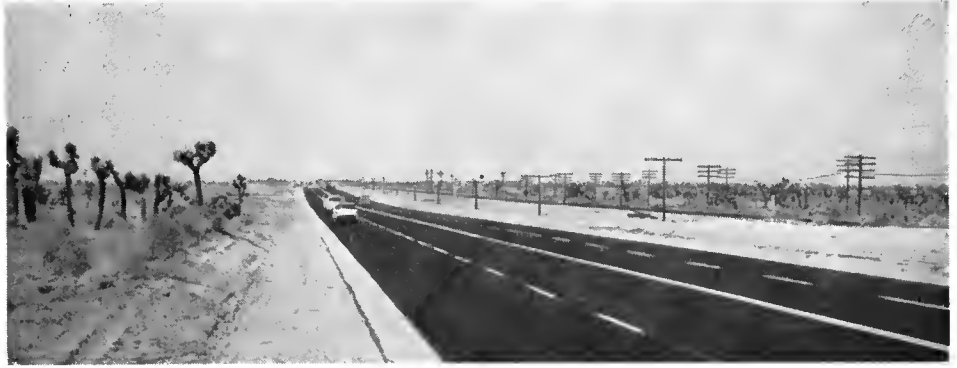
An eight-mile section of the US 6 in Los Angeles County was opened to traffic on April 15th. Reconstruction of this section of US 6, which is also known as the Sierra Highway, extends from Avenue R in Palmdale to Avenue I in Lancaster and involved four-laning the highway at a cost of $600,000. Work on the project was started last September.
