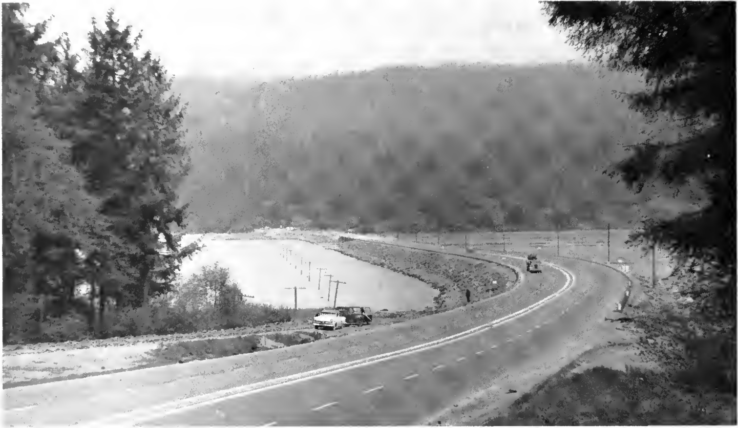
A recently completed freeway section on US 101 between Patricks Point and Big Lagaan in Humboldt County. This northward view shows the embankment across Big Lagaan which replaced the former timber trestle.
