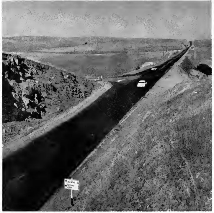
Improvement of intersections is an important part of the district construction program. Typical of these are (left) the Nimbus Intersection, an interim improvement east of Sacramento on US 50 which will eventually be replaced by a full freeway interchange and (right) the Latrobe Road intersection, also an US 50, where part of a hill was removed near the highway to give better sight distance to motorists.
