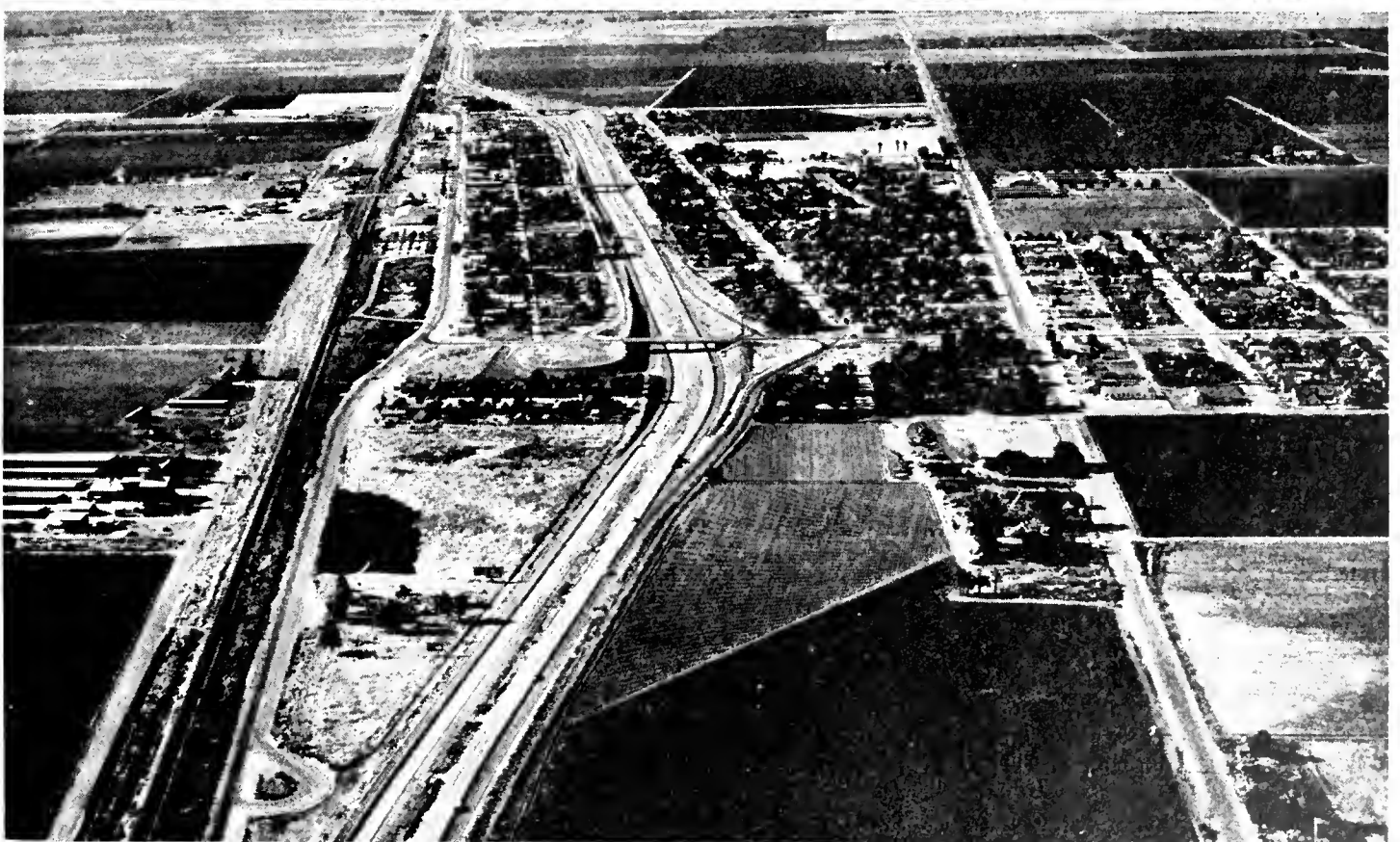
UPPER - Overcrossings carry local traffic over the new US 99 freeway bypass of Delano. LOWER - The business section of Earlimart is bypassed by the freeway on US 99. The old highway follows the railroad to the left. The view is northward.
