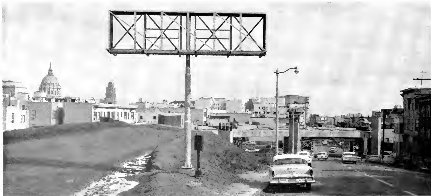
Central Freeway (U. S. 101) in San Francisco showing ramps under construction
