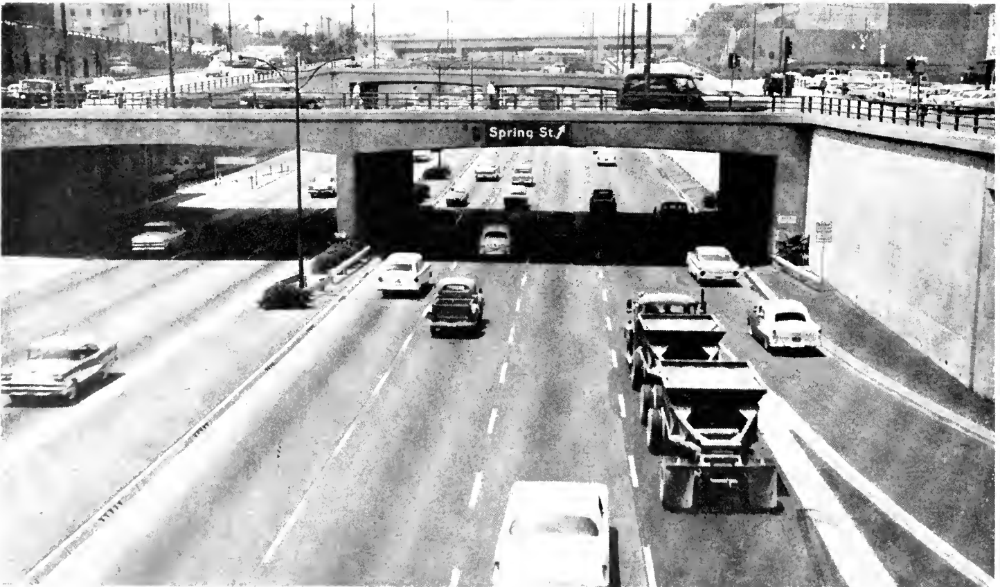
UPPER This eastward view of the Santa Ana Freeway, taken from Los Angeles Street, shows the odd lane for westbound traffic (extreme right). LOWER— A westward view of the Santa Ana Freeway of the Los Angeles Street on-ramp showing the odd traffic lane occupied by the truck and trailer (right foreground).
