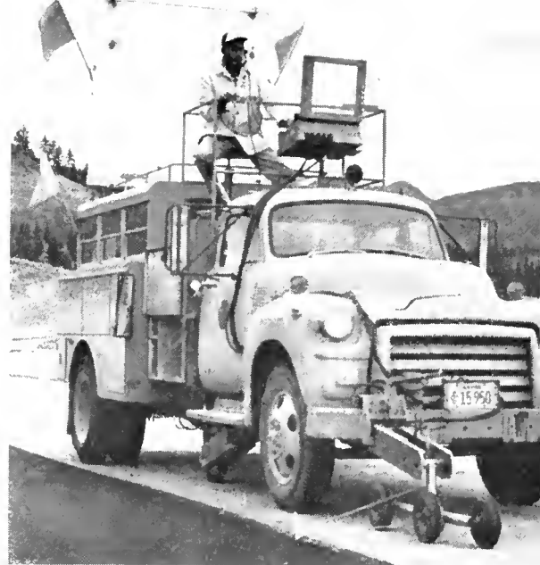
Truck-mounted profilograph checking smoothness of paving on completed section near Boca.
