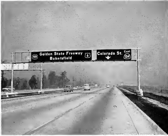
Constant improvements are being made in the design and placement of directional signs on freeways to make it easier for motorists to find their destinations. At left is an overhead illuminated sign bridge typical of those now used extensively on freeways. At right is a sign showing distances to the next three turnoffs. Standard plans and specifications for freeway sign structures have been developed and are included in major freeway construction contracts.
