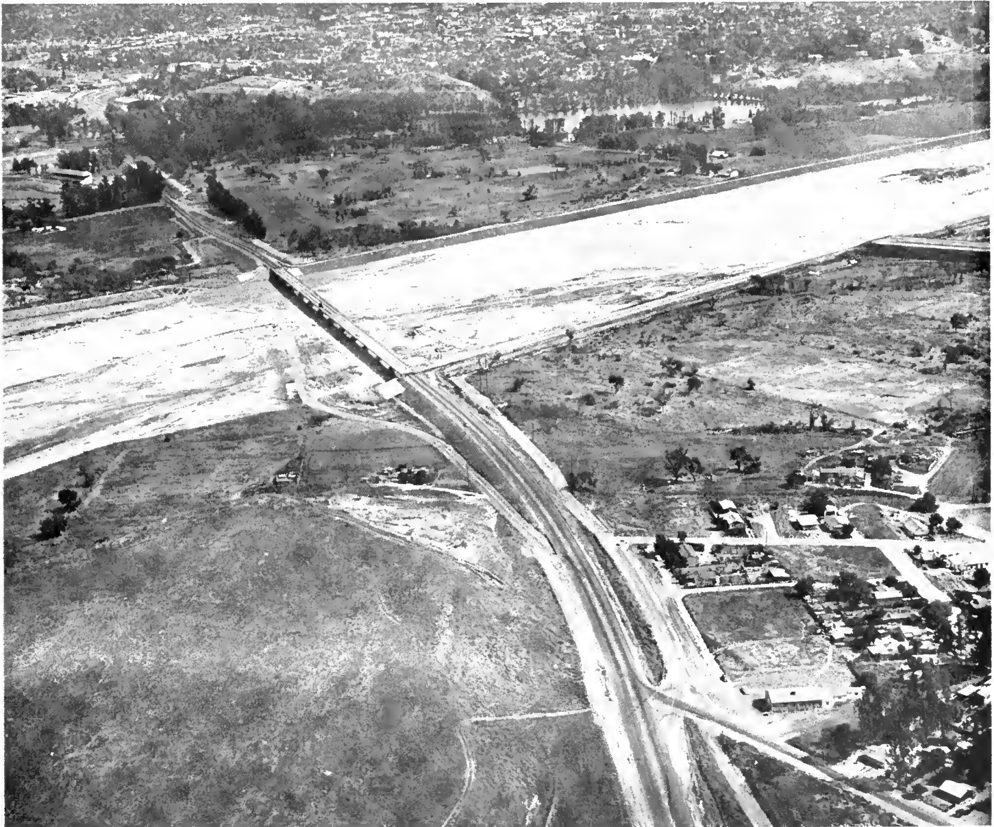
An aerial view of the new Crestmore Road and Bridge with the City of Riverside in the distance. The bridge was lengthened by Riverside County under the Federal-aid Secondary program. The river is the Santa Ana.
