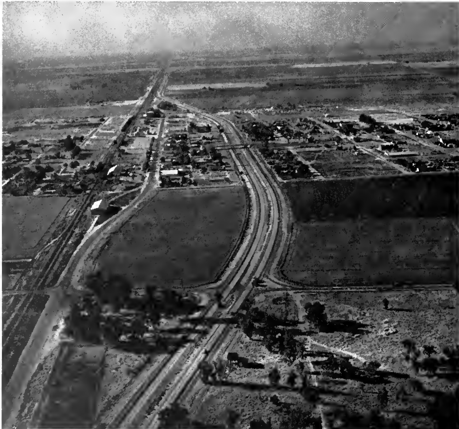
This expressway on US 99 bypasses the business section of Tipton. The structure over the expressway at the center of the picture is the Sixth Street Overcrossing. The view is to the north.
