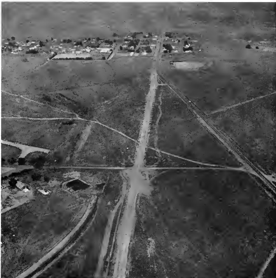
The north end of the Sign Route 41 relocation project joins the existing highway at Kettleman City.
