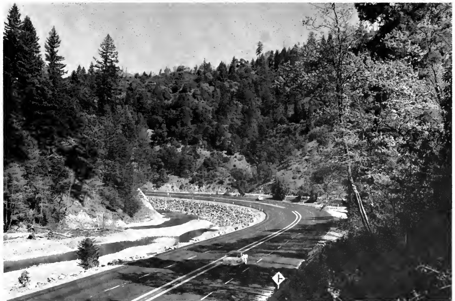
A new section of freeway on US 101 about 10 miles north of Willits in Long Valley Creek Canyon in Mendocino County.
