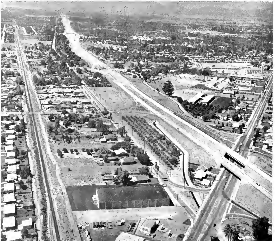
Looking northward toward Cajon Pass from the Highland Avenue (Sign Route 30) separation showing construction of the new US 66-91-395 freeway. LOWER—At present, the southern terminus of the Riverside Freeway is at Arlington Avenue in Riverside; however, construction is under way for another five and one-half miles south.
