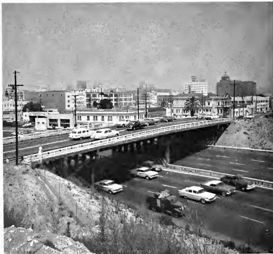
UPPER—Venice Boulevard passes under the construction area (foreground). The north end of the Harbor Freeway detour is in the middleground. LOWER—A temporary bridge carries Venice Boulevard traffic over the Harbor Freeway detour.
