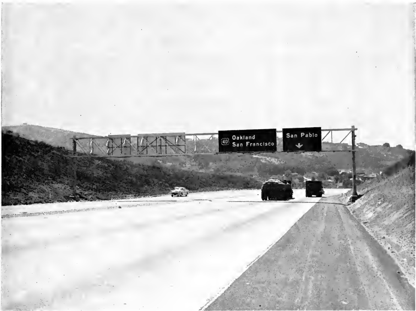
This is a sign bridge. In this type the Standard Plans cover structures up to 10 feet high by 130-foot span. Although walkways and safety railing are on this structure, they are hardly perceptible to the motorist.
