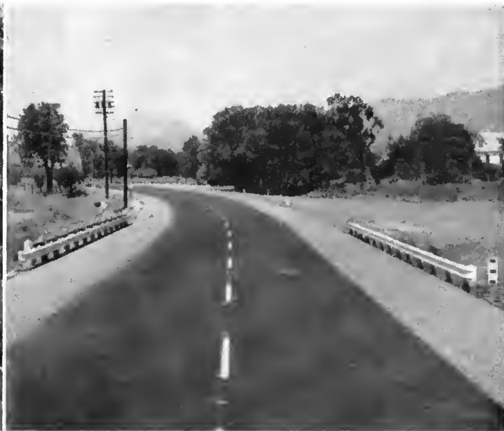
Before and after construction views of the alignment at one of the bridges on Silverado Trail, Federal-Aid Secondary Route 607. The new alignment provides large radius curves with smaller interior angles and greater sight distances.
