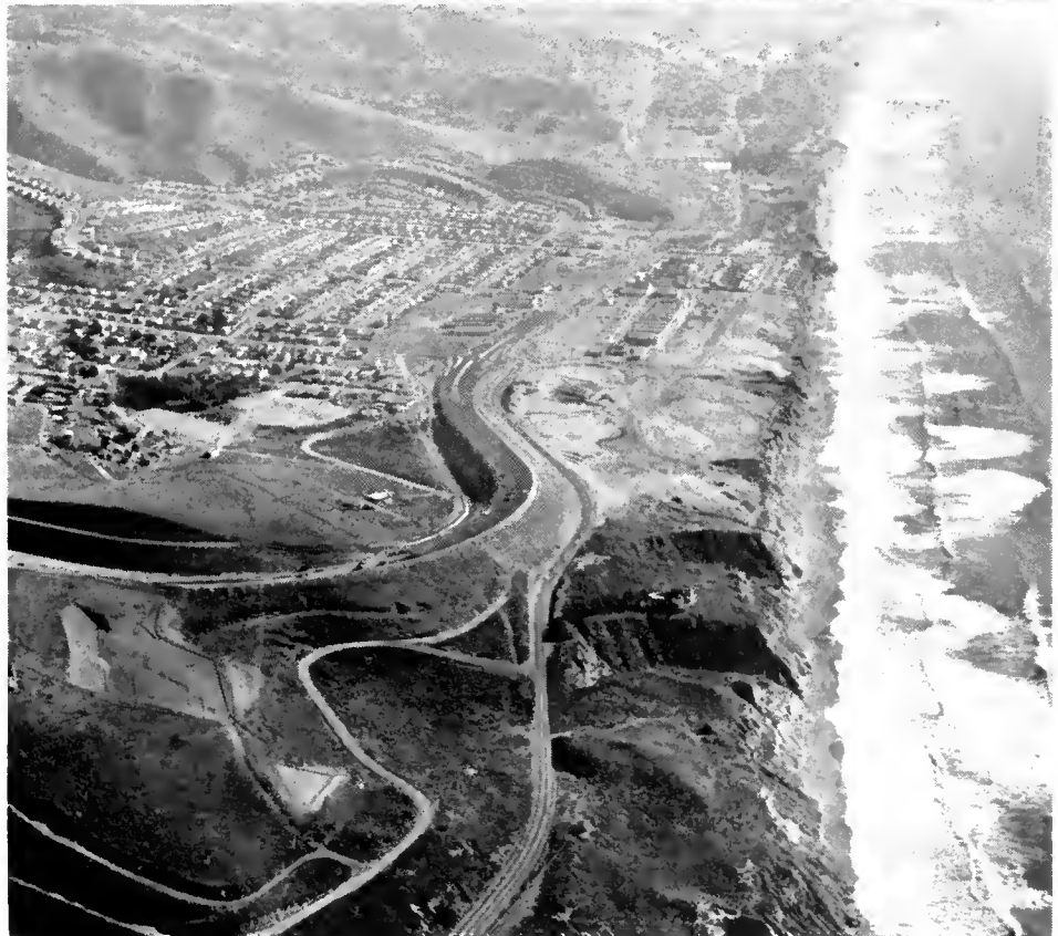
UPPER—An aerial view of the south end of the new freeway. The old road parallels the new freeway on the left before taking out around the Tharnton Bluffs in the distance. LOWER—Looking south over part of the Tharnton Bluffs showing the old highway (middle foreground) and the new freeway curving up the slope to the left.
