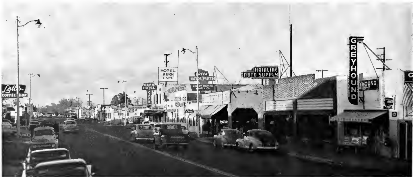
Representative section of High Street, the former state highway, looking north.
