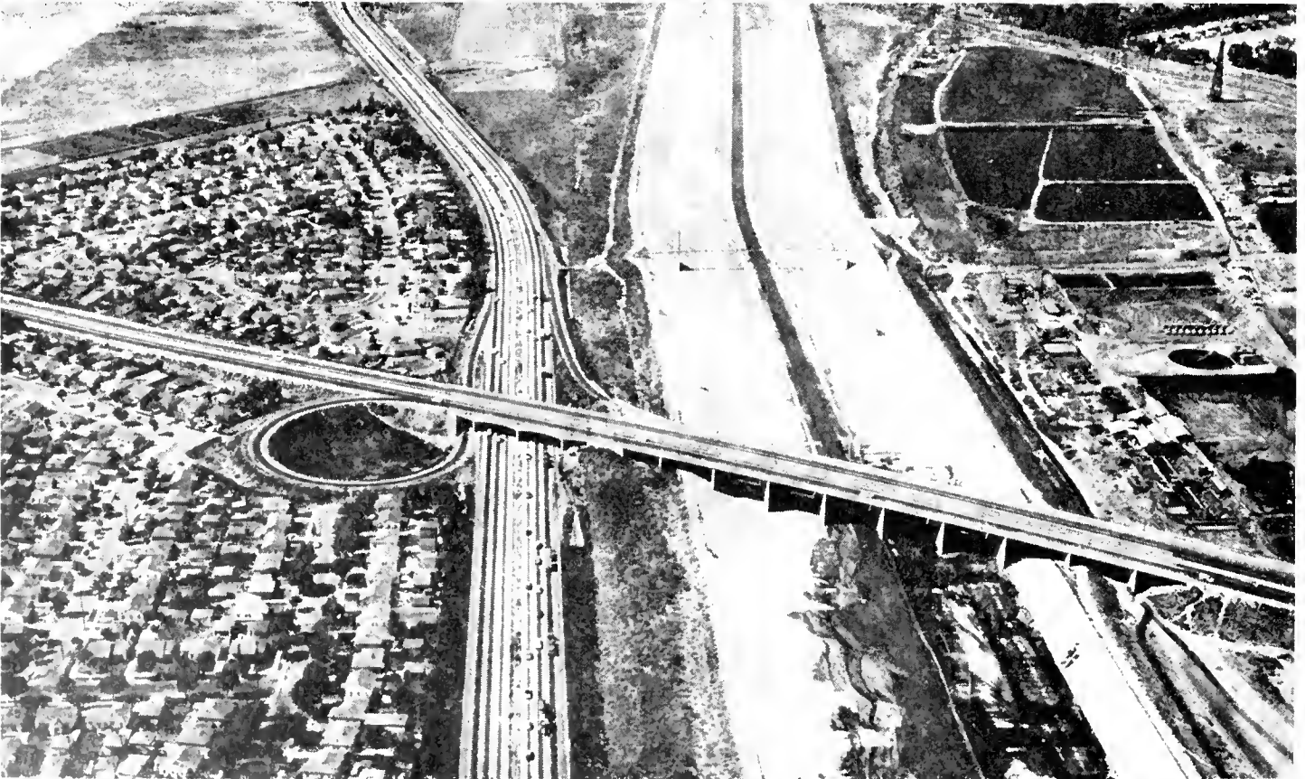
UPPER: An aerial view of the Firestone Boulevard Cloverleaf and the Los Angeles River Channel along the Long Beach Freeway. The channel joining the river from the right is the Rio Hondo. LOWER: The Belhart Street Overcrossing built by Los Angeles County.
