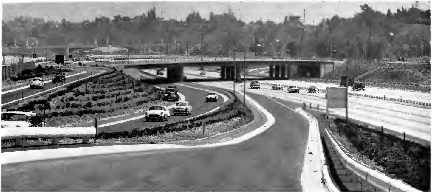
This overcrossing takes Las Feliz Boulevard traffic across the Golden State Freeway.
