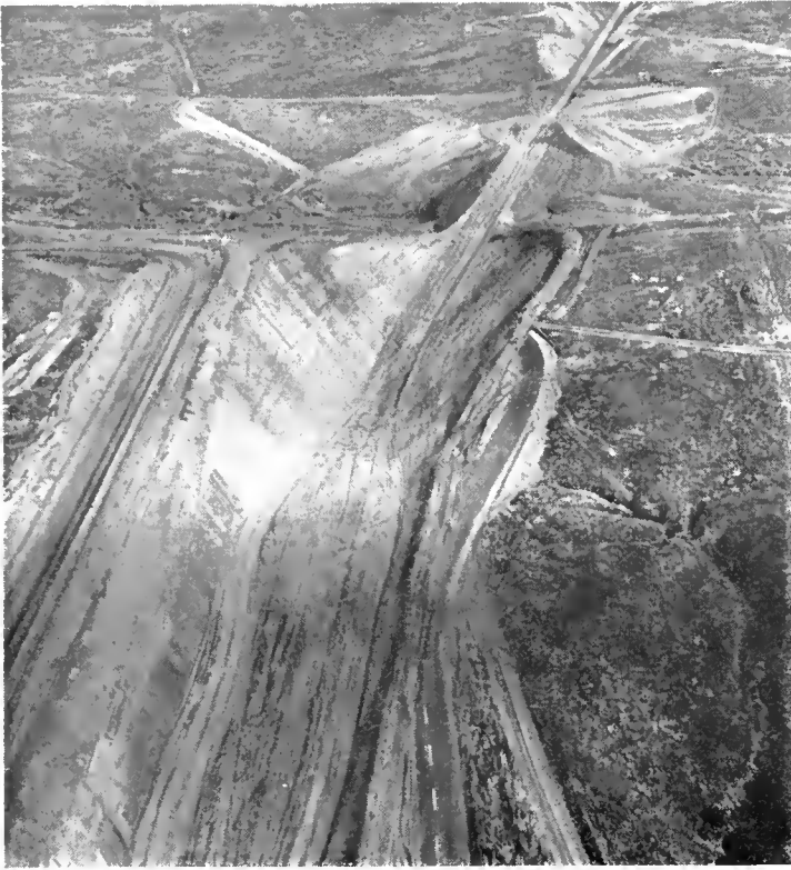
LEFT—The deepest cut (65 feet) and the highest fill (70 feet) are shown in the aerial with the detour on the left. RIGHT—This view southward from the middle of the job shows the relocated private road connections taking shape.
