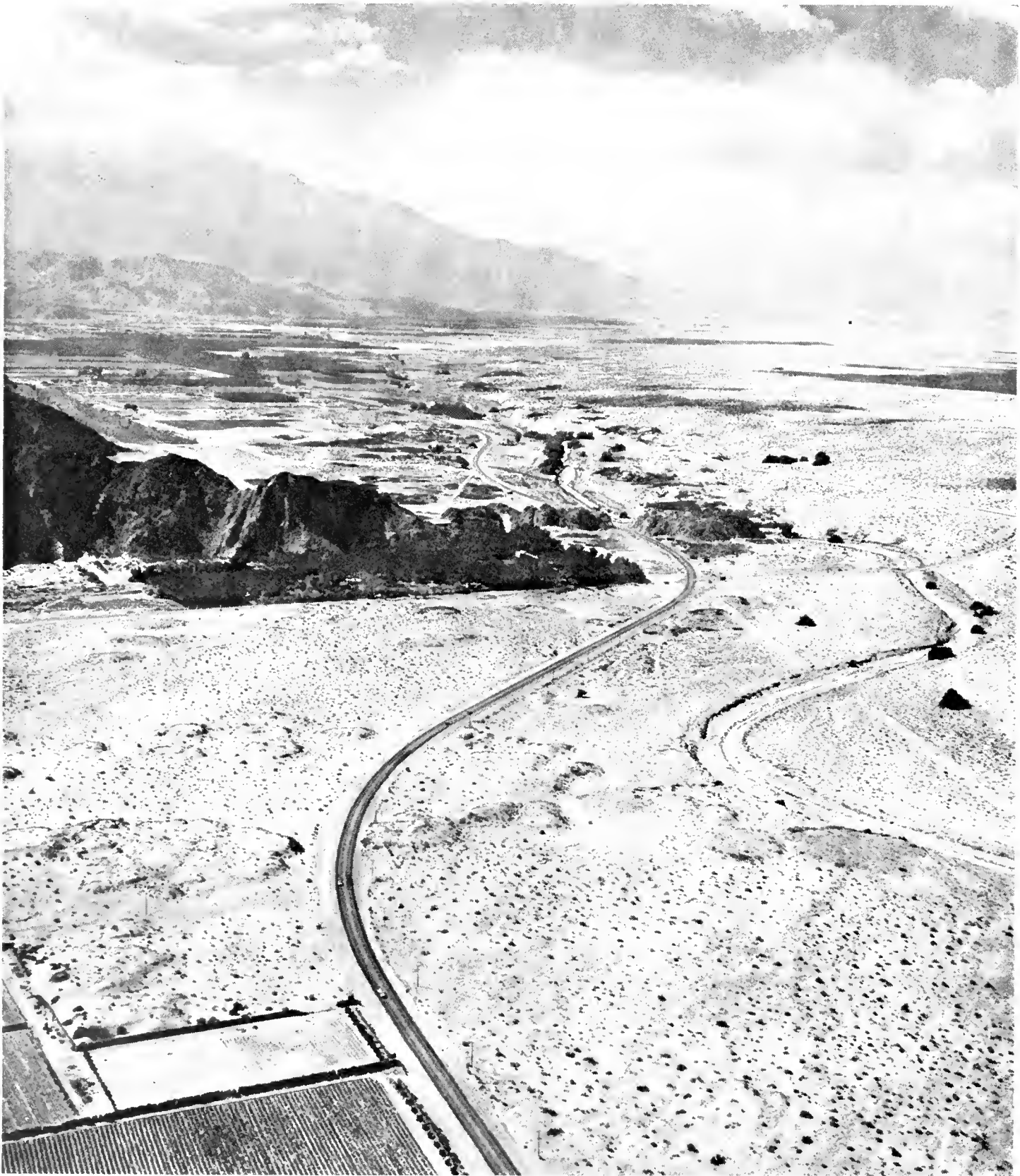
State Sign Route 111 winds its way through the desert country west of Indio in central Riverside County. Note the neatly demarked crop and orchard areas in the left fore-, middle- and background of the photo.
