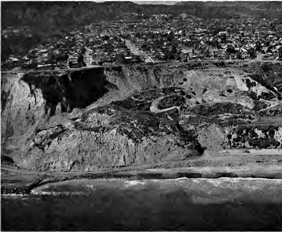
This huge landslide along the Pacific Palisades closed US Highway 101 Alternate near Santa Monica and took the life of a Division of Highways maintenance superintendent. A temporary detour was constructed to reopen the highway, and at the end of the year work was being pushed on rerouting the highway around the slide.
