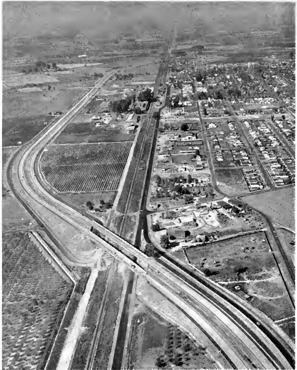
An aerial view looking northwest along the new US 99 Bypass at Atwater. In the foreground is the East Atwater overhead and the Broadway frontage road. The dark road in the center of the picture extending from foreground to background and paralleling the railroad tracks is old US 99.
