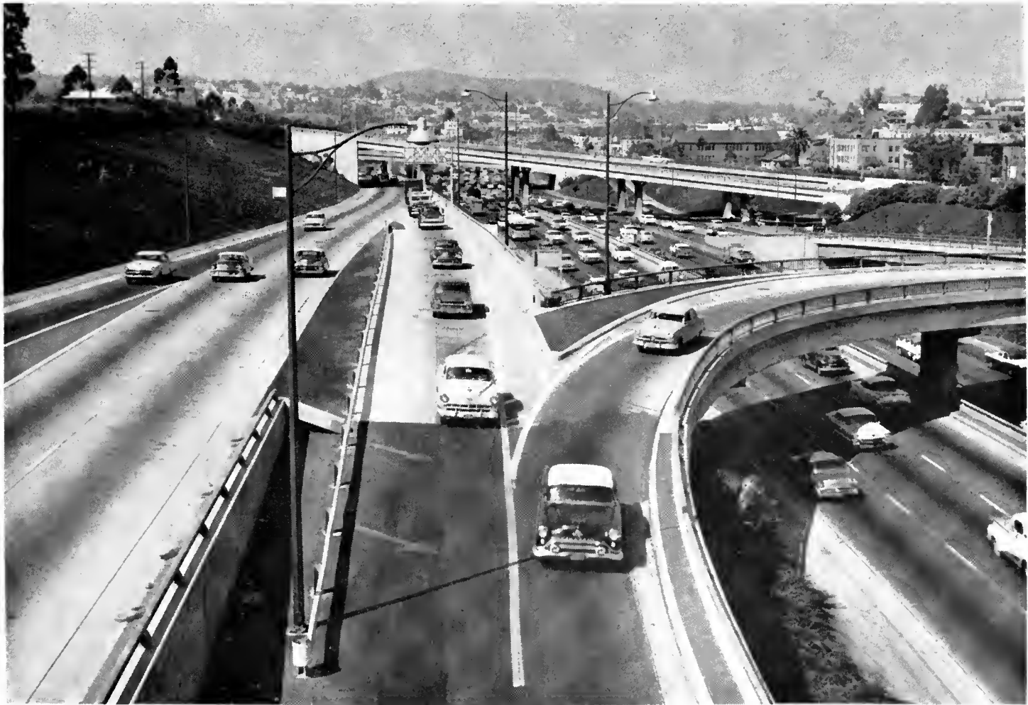
The Harbor Freeway, looking northward, showing the new slip ramp which handles traffic from the distributor road (left) to the curved Fifth Street southbound inlet (right).
