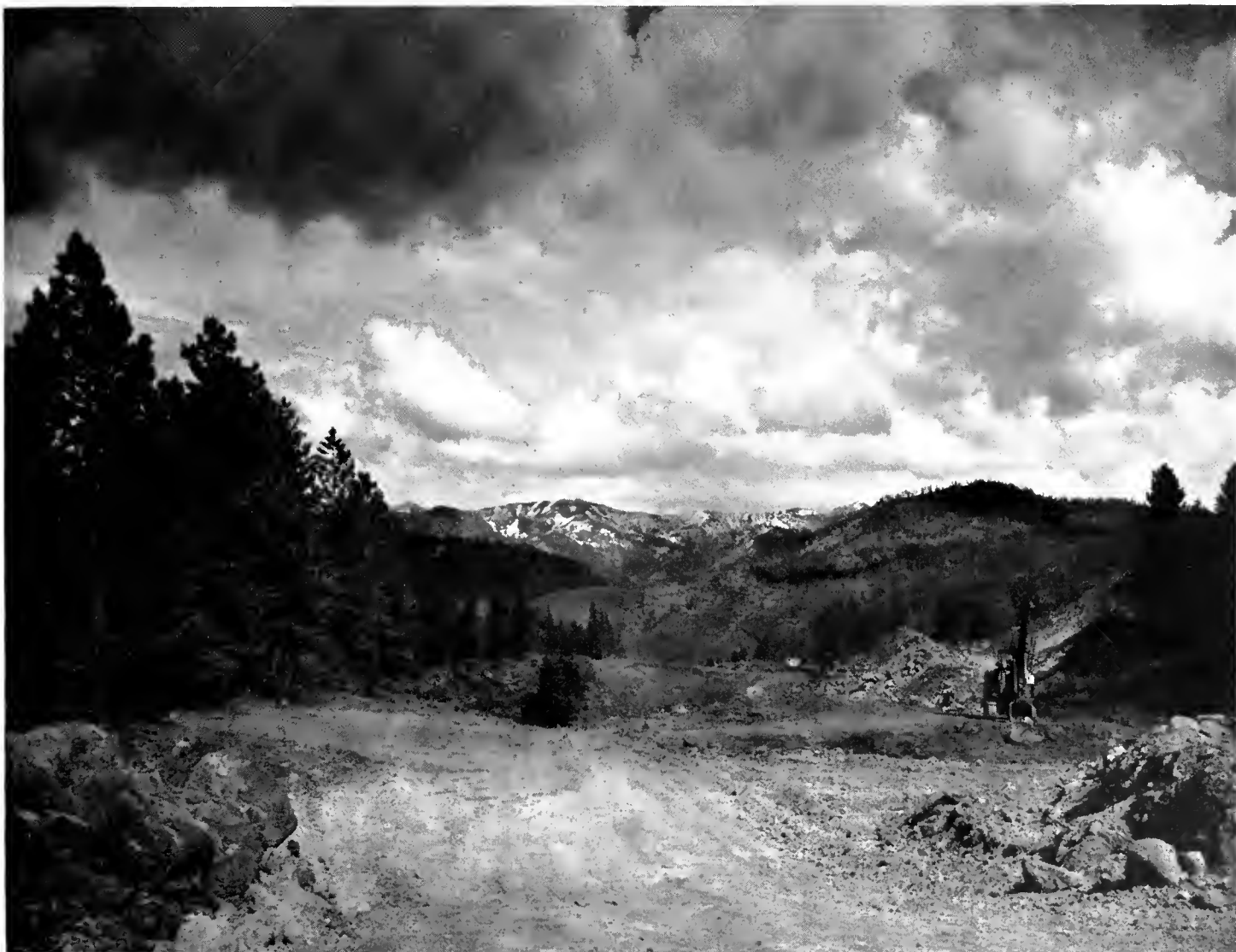
Freeway construction on US 40 near Floriston in Sierra County. The section from Floriston to the Nevada state line will be completed this summer.
