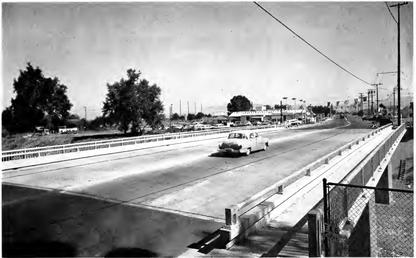
The new bridge at Pleasanton has adequate roadway width as can be seen in this photo. Space for sidewalks is also provided on each side.
