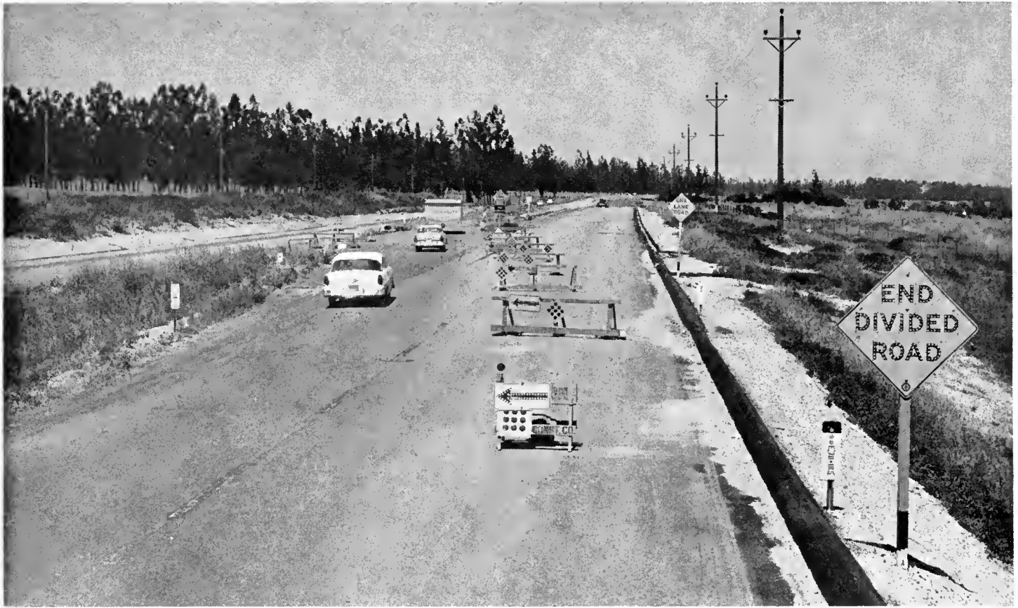
The detour at the beginning of the freeway project between King City and Greenfield during construction. Effective barricades such as this get traffic moving over the detour without delays. Some 9,000 vehicles a day use this section of US 101.
