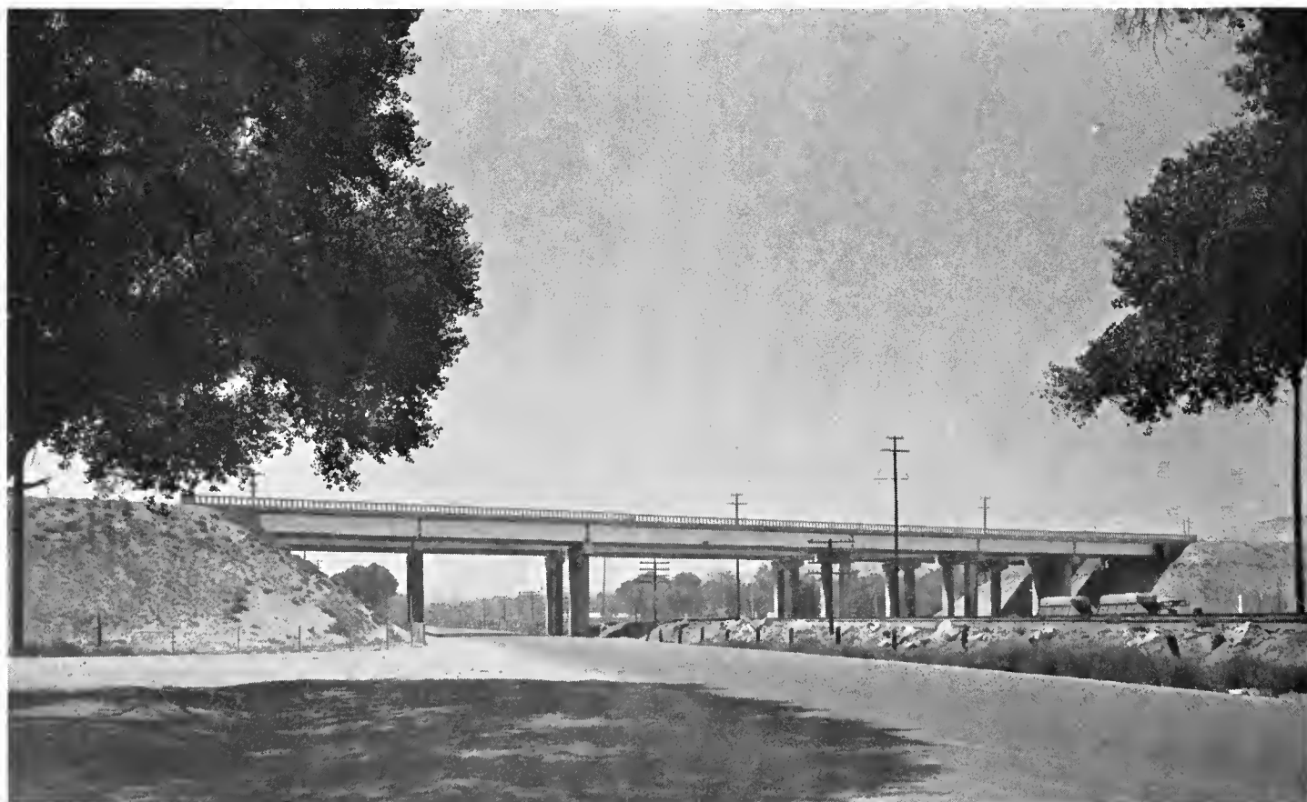
The Victorville Overhead carries the new freeway over the old highway and railroad tracks
