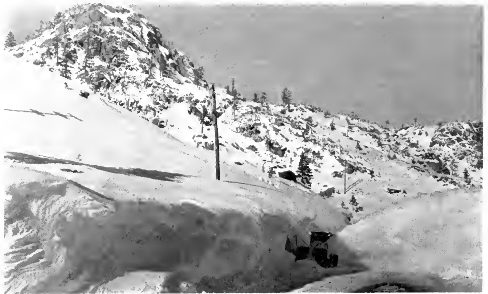
Snow removal in the passes of the Sierr Nevada Mountains is a difficult job handled each winter by the division's maintenance men. Here a rotary plow chews into a high snow bank on US Highway 40 near Donner Summit and deposits the snow on the far side.
