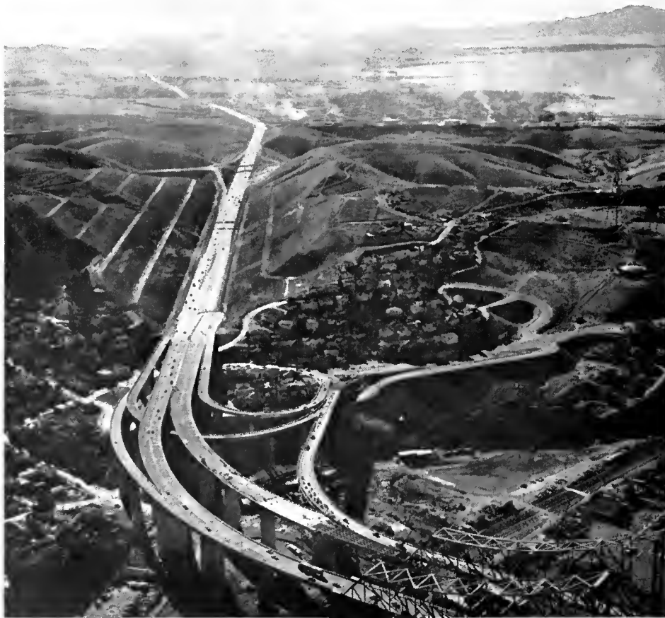
Motorists on the new US Highway 40 freeway approaches to the Carquinez Bridges in Contra Costa County travel through a manmade canyon believed to be the largest cut in the history of road building. The "Big Cut" is a quarter-mile wide at the top and up to 350 feet deep.
