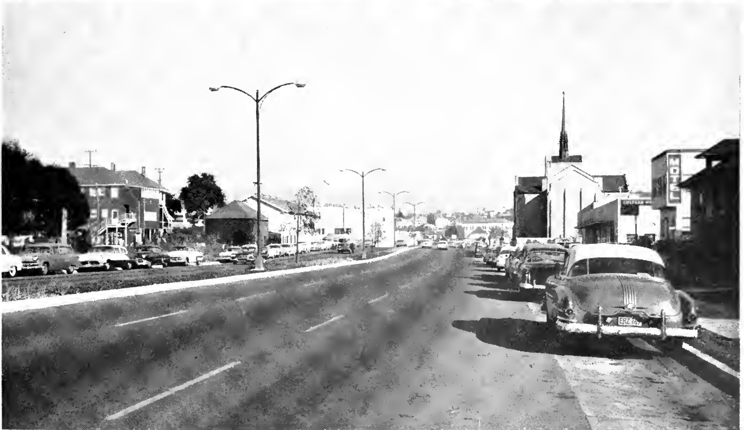
UPPER—This photo taken in 1953 looking eastward along 27th Street shows the end of the street, private homes and the U. S. Government housing that was removed to make way for the roadway. LOWER—This photo was taken from approximately the same location as the one above after the new divided roadway was completed in 1958. For a point of reference note the church spire in the right background of both pictures.
