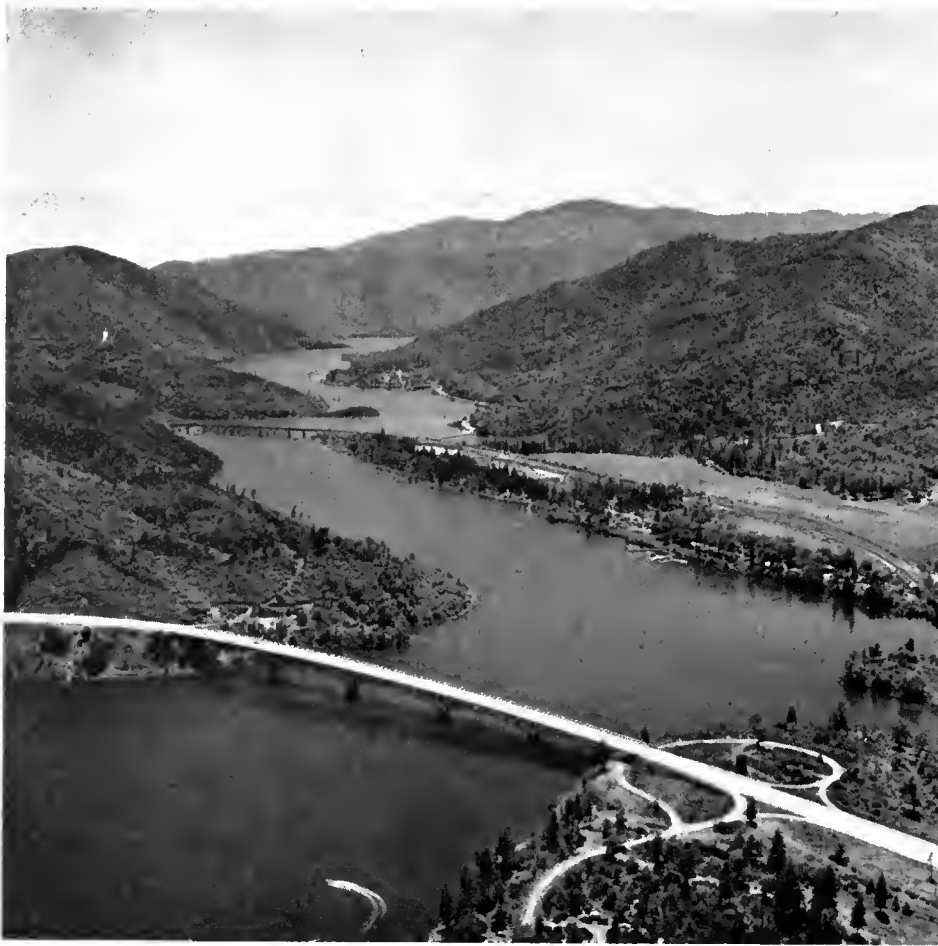
The Antler Bridge on US 99 spans the Sacramento River arm of Shasta Lake. The Southern Pacific Railroad Bridge is in the background. The connection to the U. S. Forest Service Antler Campground is in the lower right.
