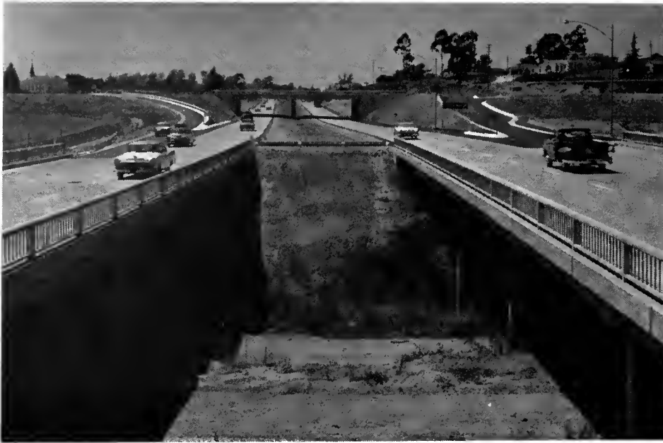
These twin bridges carry the US 101 freeway across Arroyo Grande Creek in San Luis Obispo County.
