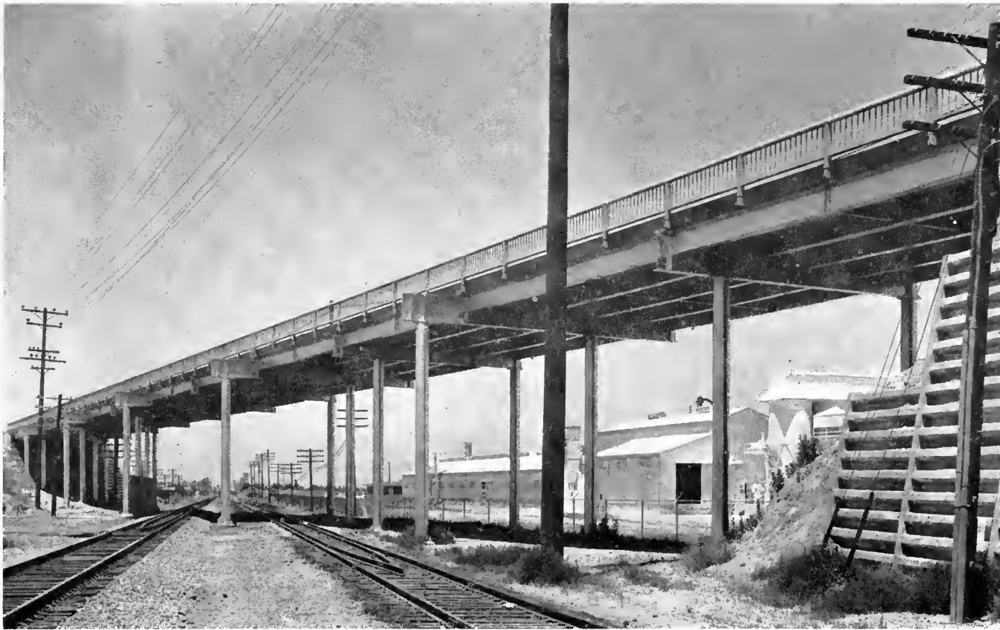
The new overcrossing which carries Wilbur Avenue traffic over the Santa Fe Railroad Tracks east of Antioch. Note the method of aligning the columns to make them parallel to the tracks by staggering their positions in relation to the highway structure.
