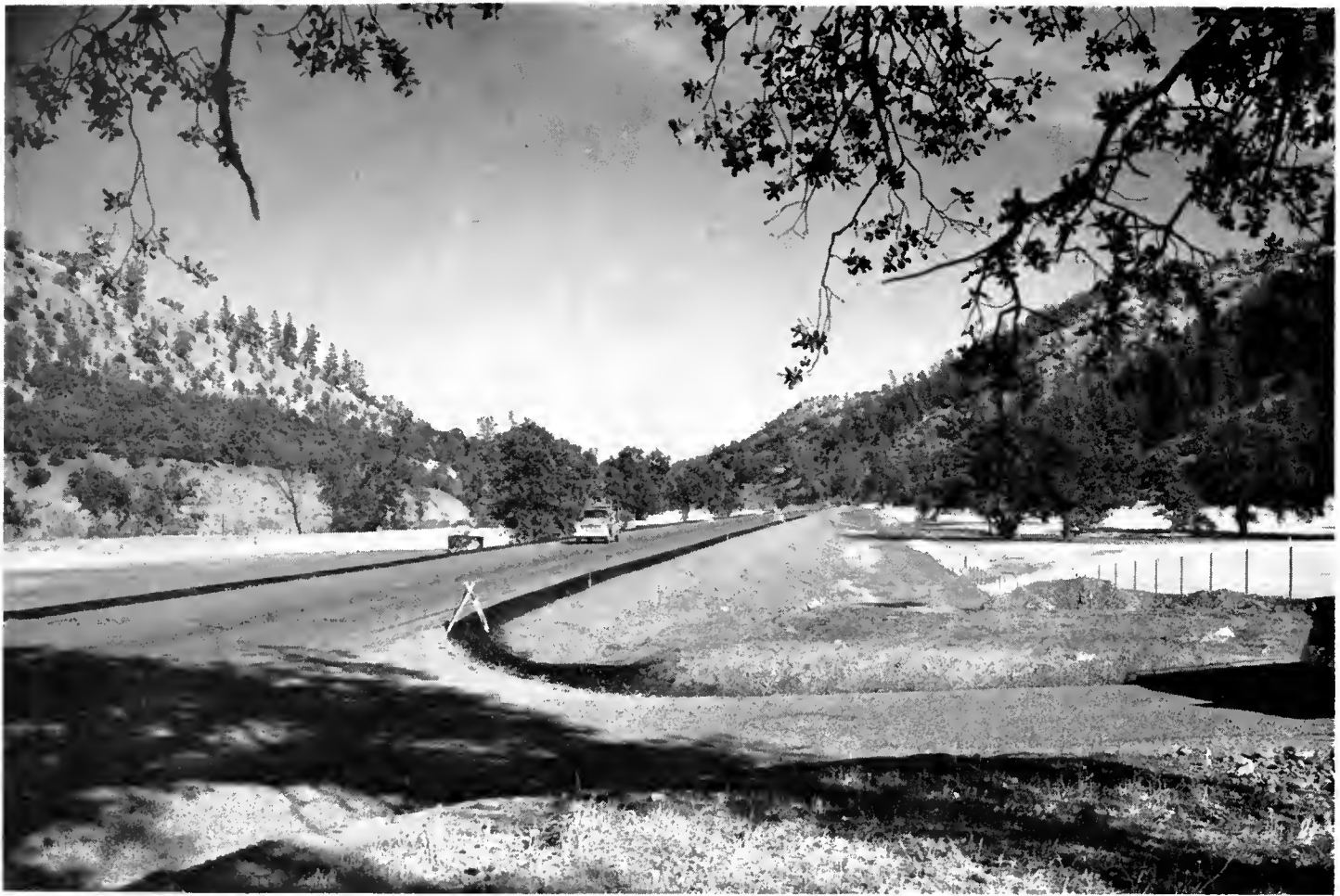
A new section of two-lane highway on State Sign Route 36 in Tehama County 31 miles west of Red Bluff.
