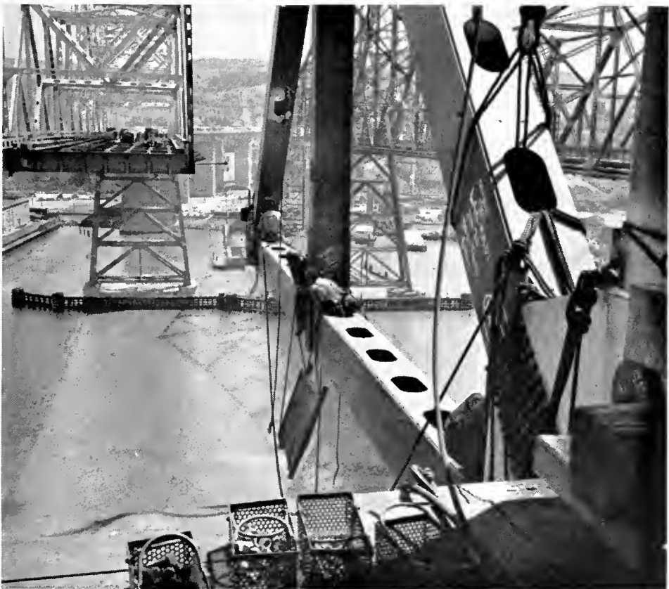
UPPER—For erection of the south anchor arm, steel was brought to the site by water from the Richmond assembly yard on barges. It was lifted into place by a 146-ton tower derrick mounted on two barges and assisted by stiff leg skid travelers. Most of the steel members were erected by cantilevering out; however, near each of the end towers eight panels of the suspended span were temporarily used as falsework, a portion of which can be seen in the lower left hand corner of the picture. LOWER—The bridge grows piece by piece to join with the other half of the cantilever span 145 feet above the waters below.
