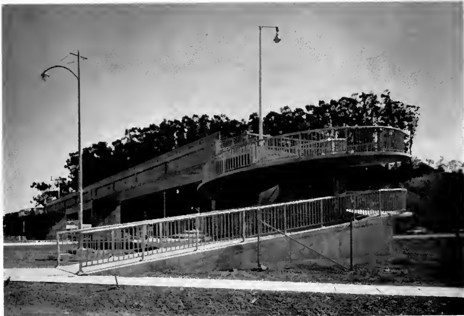
This pedestrian overcrossing near the Richardson Bay Bridge on US 101 in Marin County is typical of such structures being built across freeways throughout the State.
