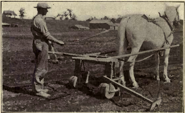
FIG. 9—MACHINE FOR MARKING DISTANCES TO PLANT
