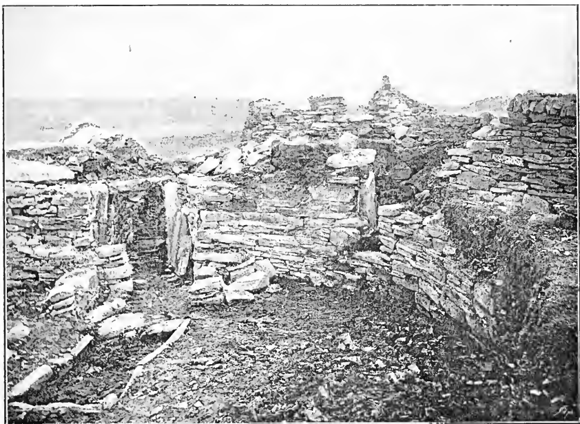
View showing main entrance and entrance to south chamber, as fully excavated.
