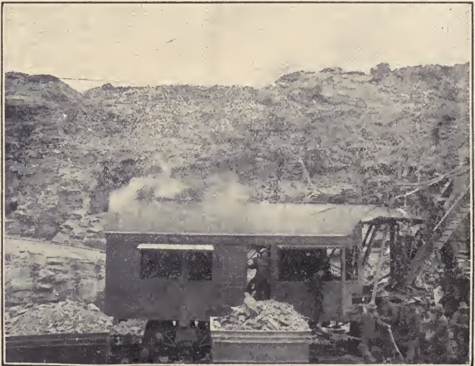
FIG. 78.—Steam-shovel in cement-rock quarry.
