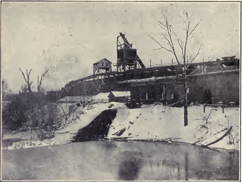
FIG. 42.—Kilns and kiln-housing, Speed plant, Speeds, Ind.
