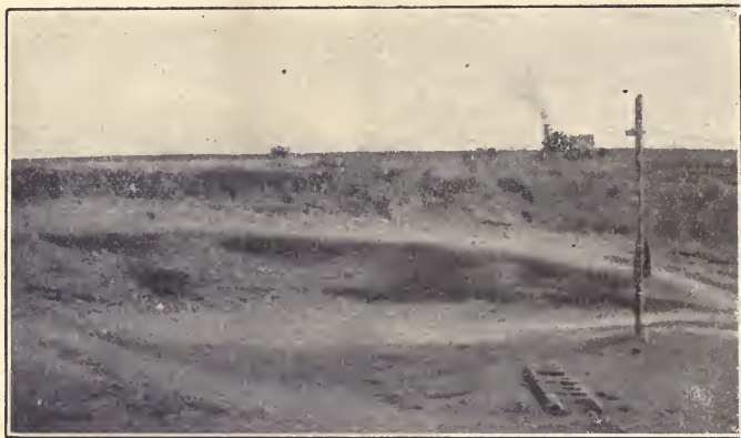
FIG. 71.—Stripping a flat, shallow bed.
