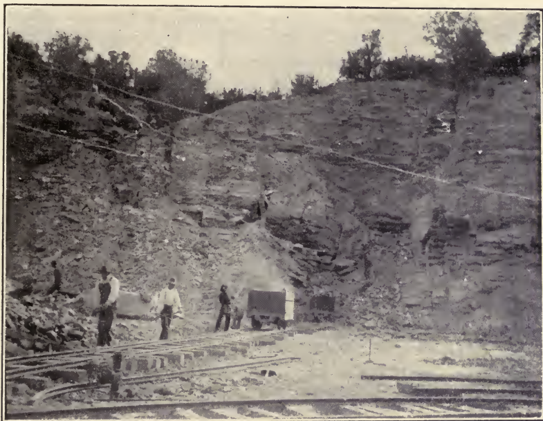
FIG. 68.—Open cut in cement rock.
