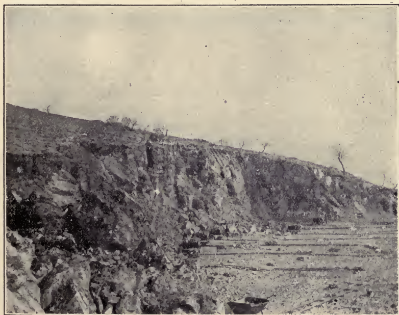
FIG. 73.—Temporary tracks laid to face.
