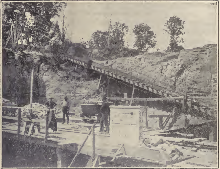
FIG. 77.—Hoisting from quarry worked in levels.
