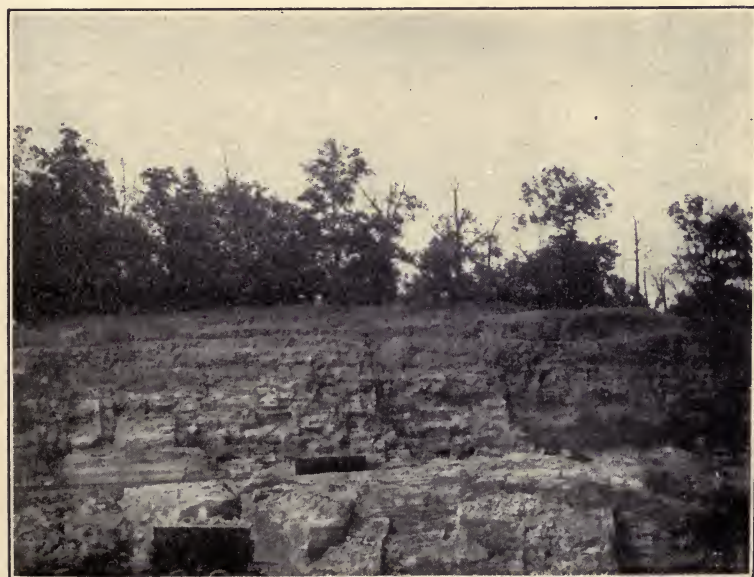
FIG. 76.—Shale-pit worked in two levels.
