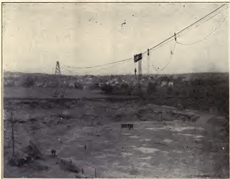
FIG. 74.—Cableway in cement-rock quarry.
