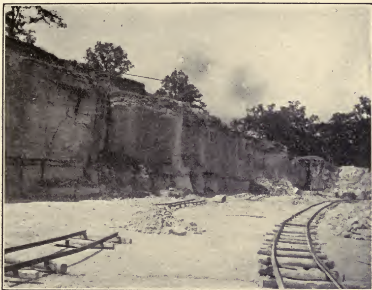
FIG. 66.—Working heavy horizontal bed of limestone.
