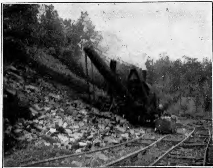
FIG. 79.—Steam-shovel handling limestone.
