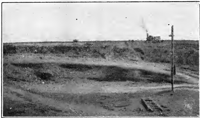
FIG. 71.—Stripping a flat, shallow bed.
