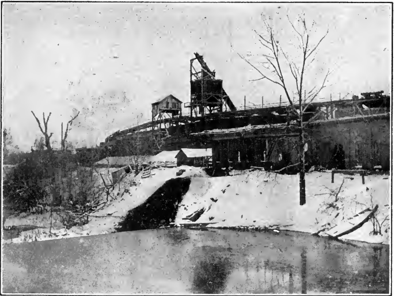
FIG. 42.—Kilns and kiln-housing, Speed plant, Speeds, Ind.
