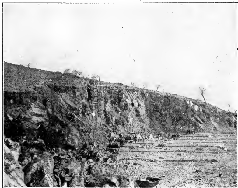
FIG. 73.—Temporary tracks laid to face.
