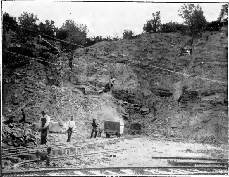
FIG. 68.—Open cut in cement rock.
