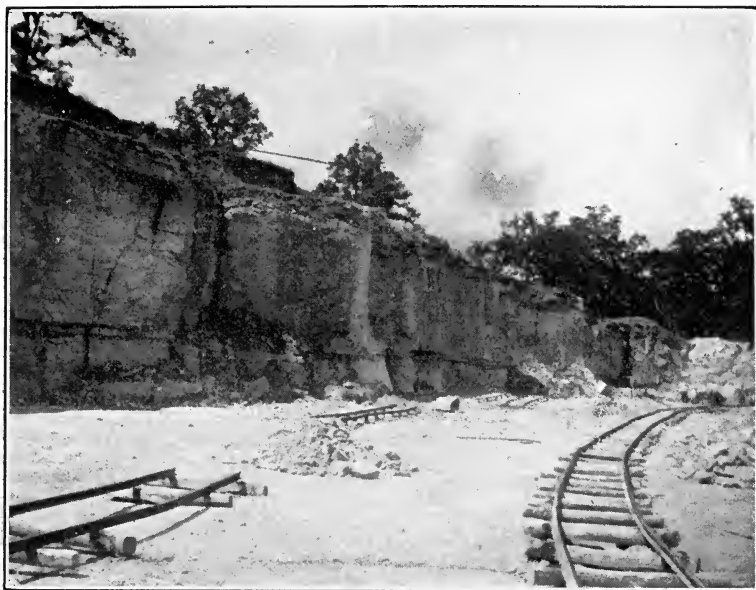
FIG. 66.—Working heavy horizontal bed of limestone.
