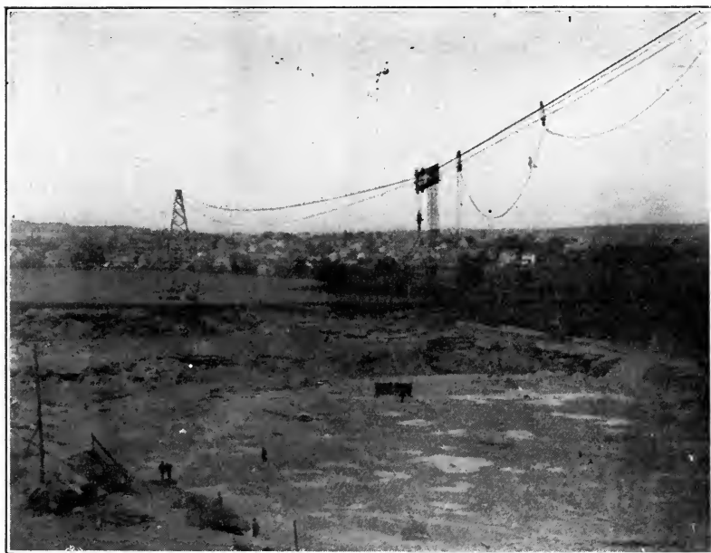
FIG. 74.—Cableway in cement-rock quarry.
