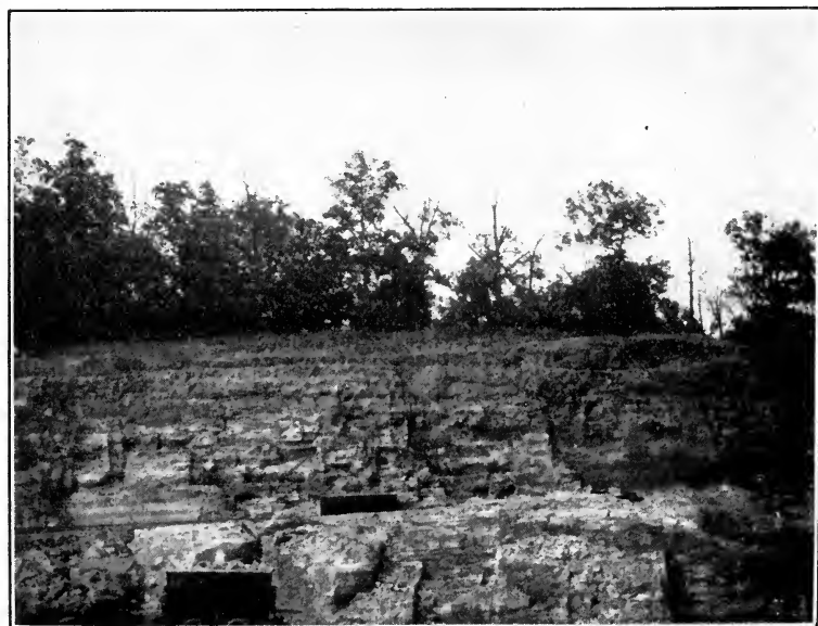
FIG. 76.—Shale-pit worked in two levels.
