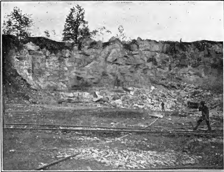
FIG. 65.—Working thick limestone-bed.
