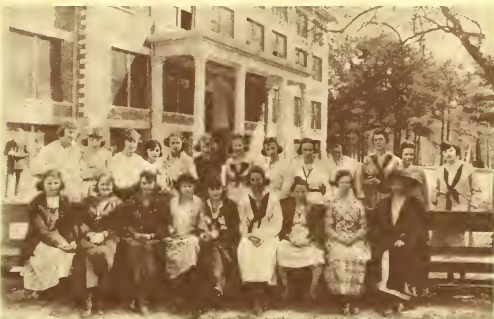
The Centenary ladies of 1920 pose before Jackson Hall.
