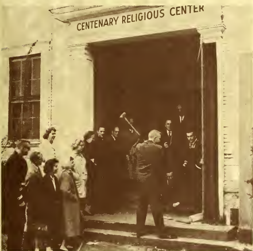
Destruction precedes construction, and appears to be more fun.
