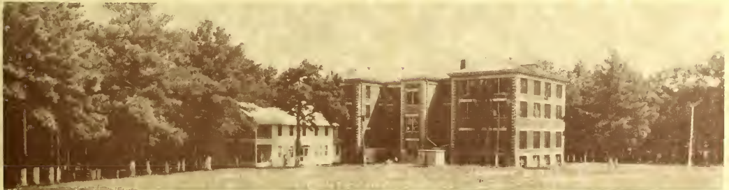
Moving the dining hall and kitchen to a wooden building made available much needed space for classes and dormitory rooms in the rapidly deteriorating Jackson Hall.
