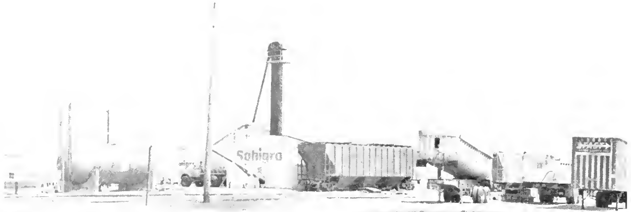
THE SOHIGRO PLANT – 1975
