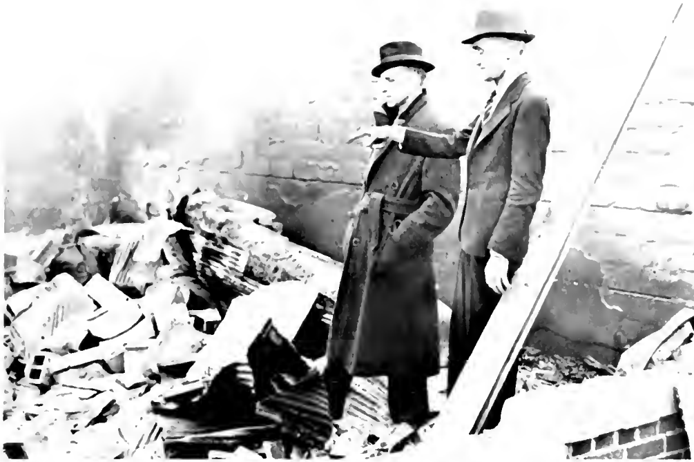
WOOLDRIDGE AND SIDDENS INSPECTING THE REMAINS OF THE DRUG STORE THE MORNING AFTER THE FIRE
