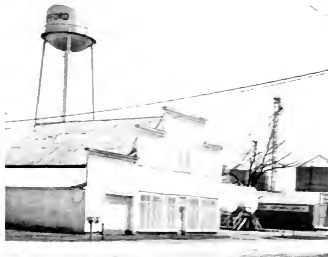
The BUSBOOM WAREHOUSE & Oil Tanks — 1975
