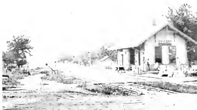
THE DEPOT, LOOKING WEST FROM MAIN STREET The small white building at the left is believed to be the first depot for the narrow-gauge railroad.
