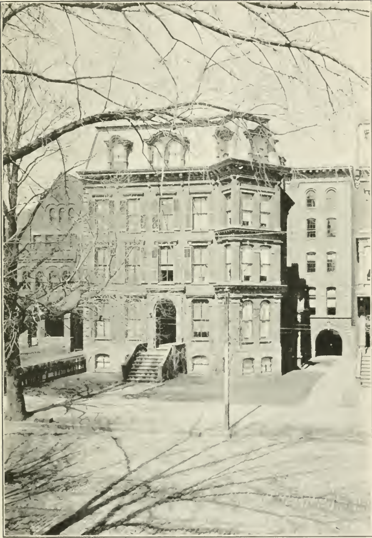
THE PRESENT BUILDINGS
