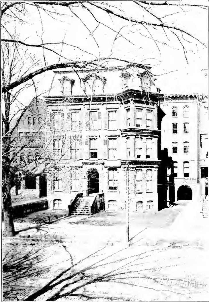
THE PRESENT BUILDINGS
