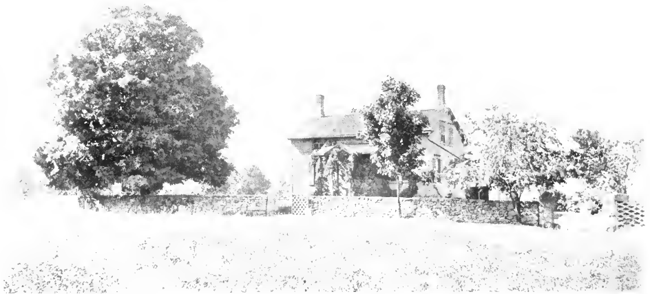
THE OLD JOHN BROWN HOME BEFORE BEING REMODELED
