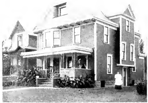
RESIDENCE OF ELMER A. GAULT, AKRON
