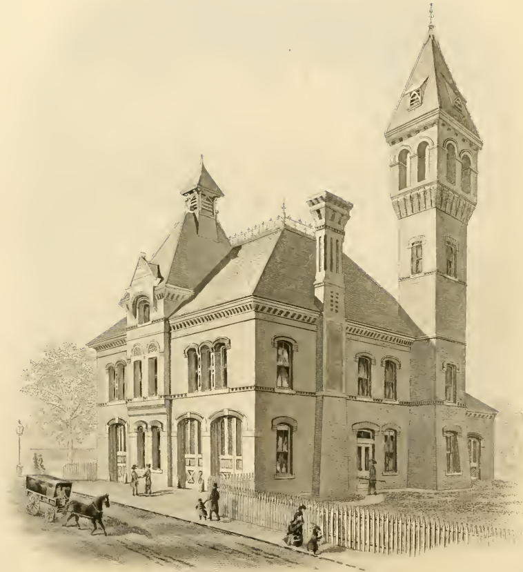
Engine House EIGHT FID WAY
