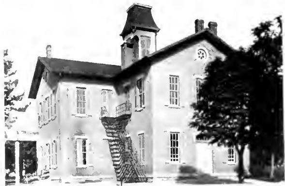
SCHOOL HOUSE, WEST MILTON
