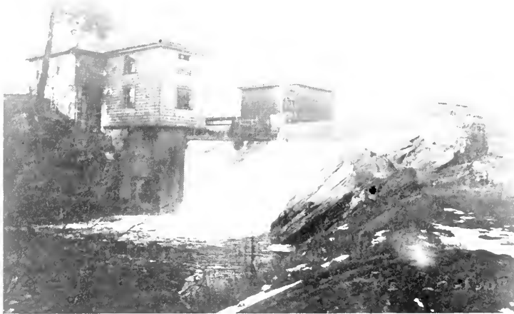
Shenipsit Dam and High Service Pumping Plant.
