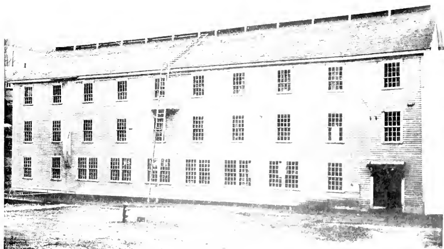
OLD ROCK FACTORY, WHICH WAS FIRST WOOLLEN FACTORY OF ANY SIZE BUILT IN ROCKVILLE, STILL STANDING.
