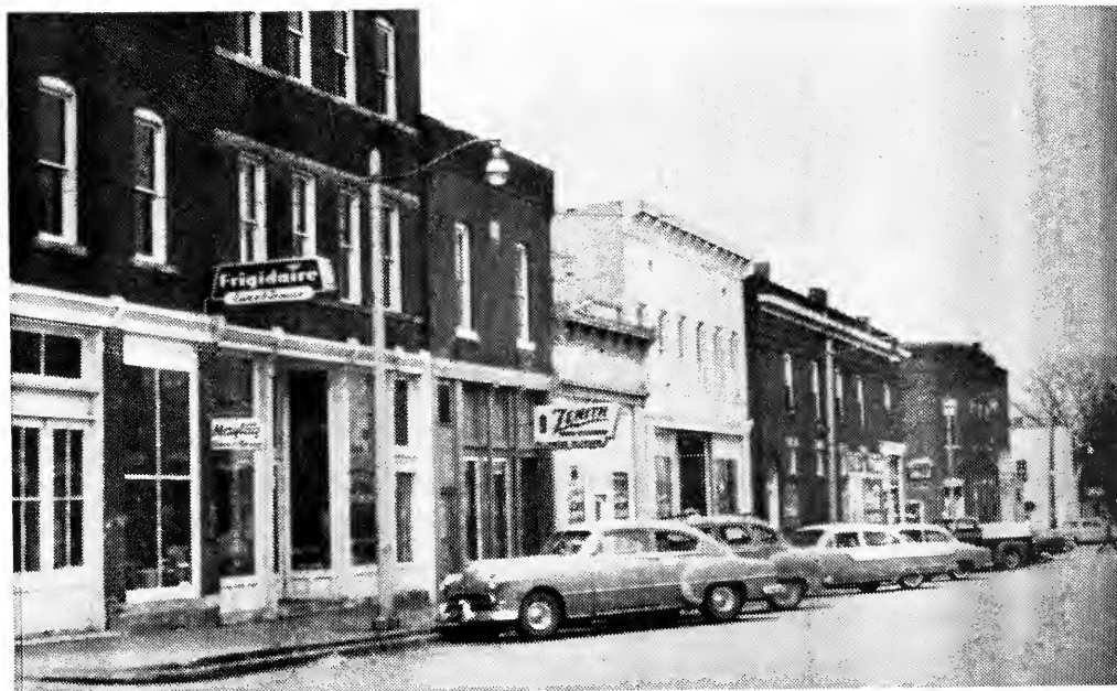
LOOKING WEST ON EAST ATTICA STREET
