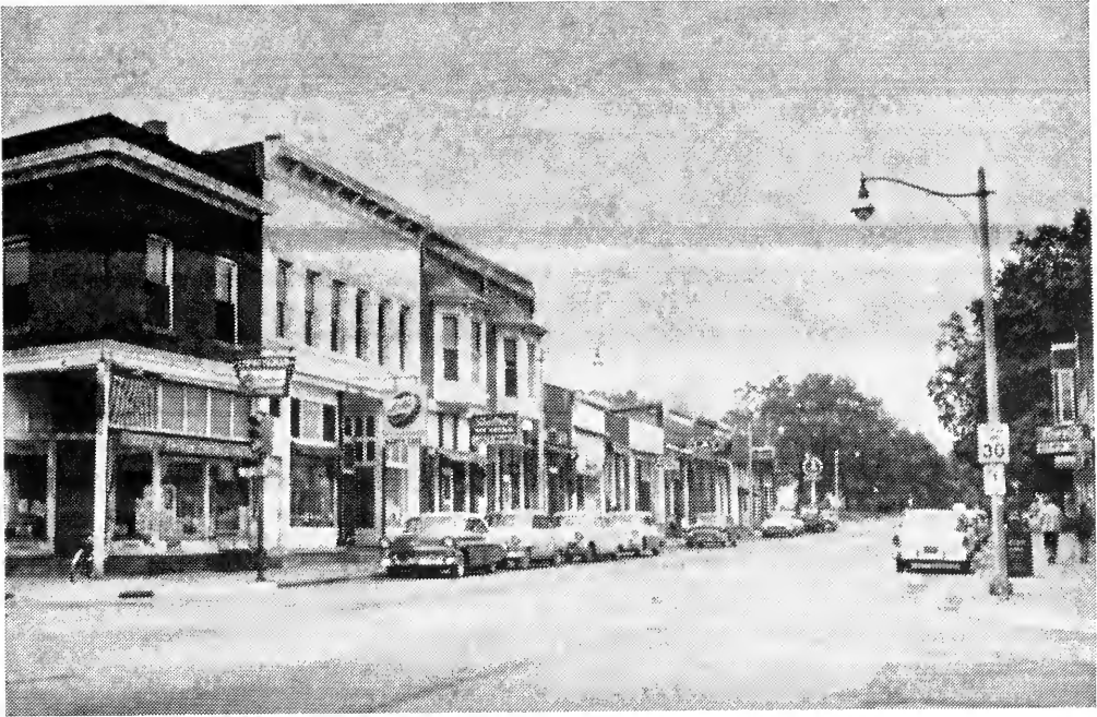
LOOKING SOUTH ON CHICAGO STREET.
