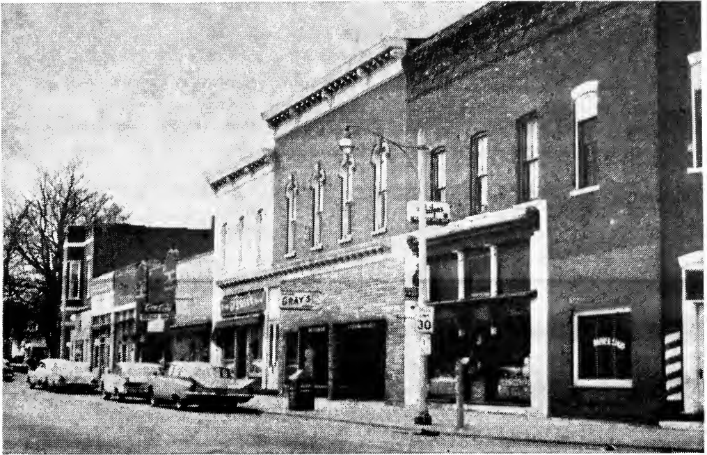
LOOKING SOUTH ON CHICAGO STREET
