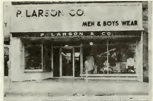
NEW FRONT INSTALLED AT PAXTON IN 1958!
