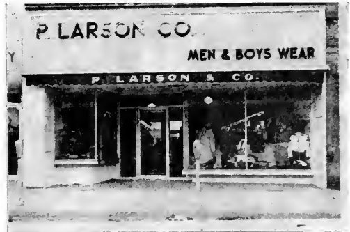
NEW FRONT INSTALLED AT PAXTON IN 1958!
