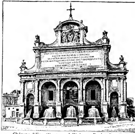
Château d'Eau (Fontana dell'Acqua Paola), Rome. (From "Baudenkmalern in Rom," pub. by Wasmuth, Berlin.)
