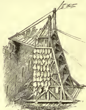
Belfry used in the assault of a medieval fortress. (From Viollet-le-Duc's "Dictionnaire de l'Architecture.")
