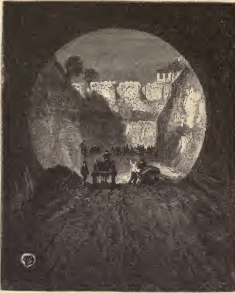
CUTTING ON UNION RAILROAD, SEEN FROM TUNNEL.
