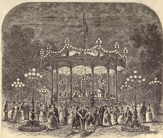
MABILLE. THE CENTRAL PAVILION.
