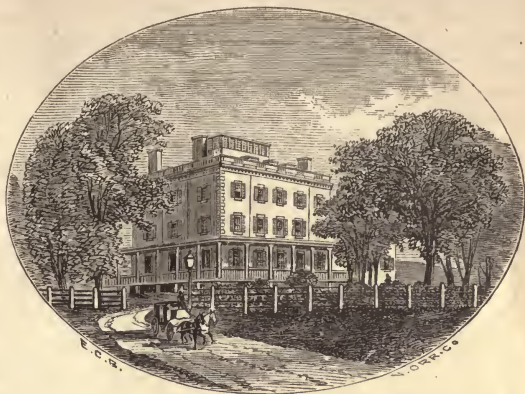
THE WEST POINT HOTEL (FORMERLY ROE'S)
