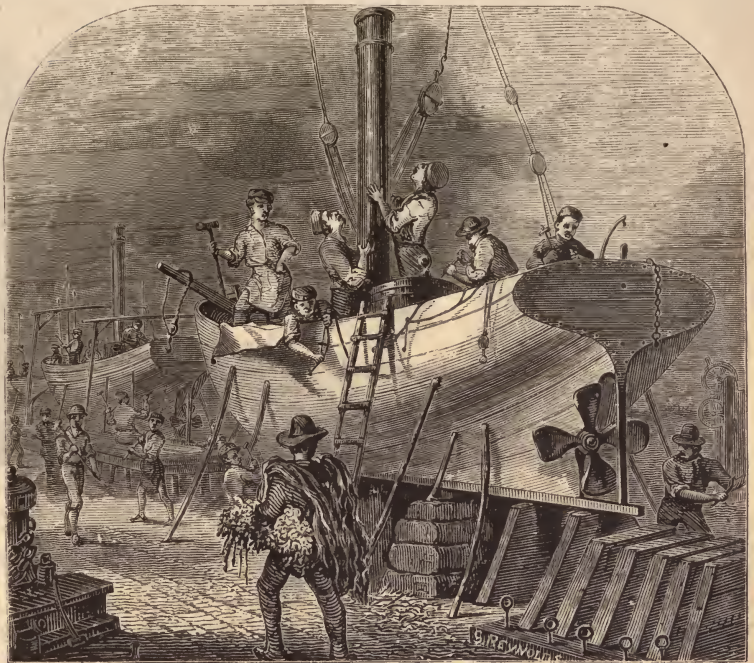
BUILDING STEAM YAWLS AT THE NAVY YARD.
