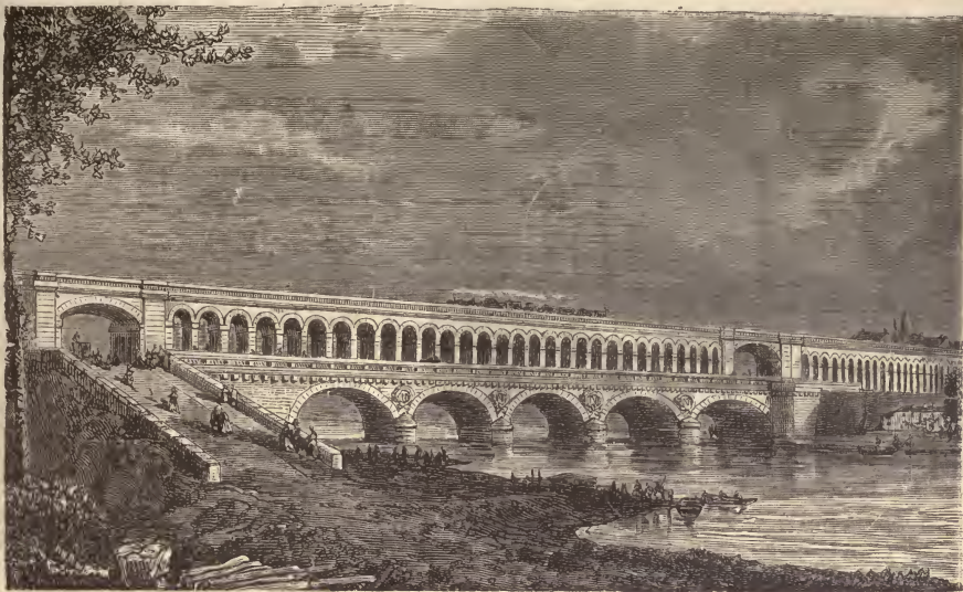
THE CIRCULAR RAILWAY VIADUCT.
