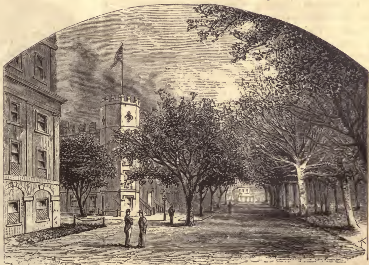
ROAD IN FRONT OF CADET BARRACKS.
