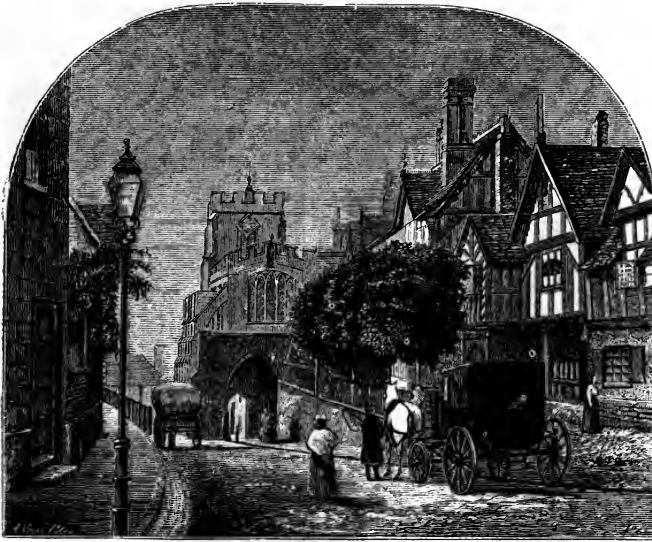
ST. JAMES'S HOSPITAL, HIGH STREET.
