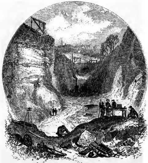
CLAY-CUTTING, UNION RAILROAD, BALTIMORE.
