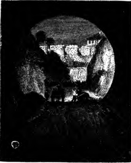
CUTTING ON UNION RAILROAD, SEEN FROM TUNNEL.
