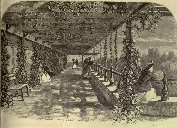
VINERY NEAR CASINO, OVERLOOKING THE MALL.
