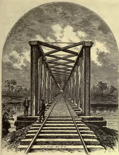
BRIDGE ACROSS ARKANSAS RIVER—M., K. AND T. RAILWAY.
