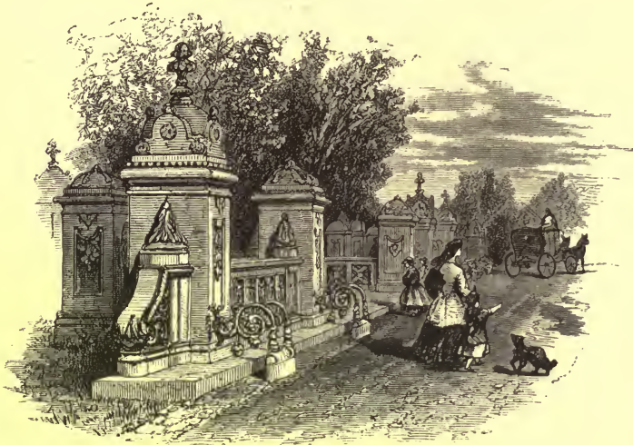
STONE SCREEN DIVIDING PLAZA FROM CARRIAGE-ROAD.
