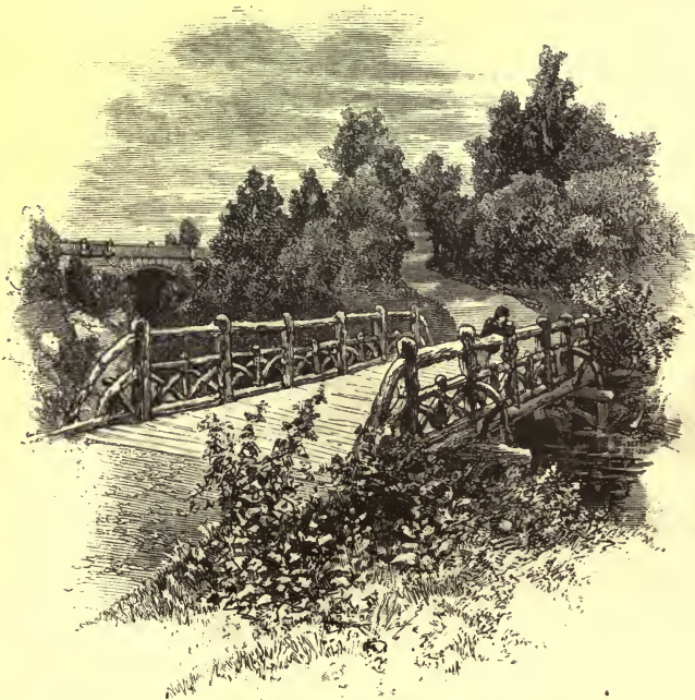
RUSTIC BRIDGE NEAR BALCONY BRIDGE, LOOKING EAST.
