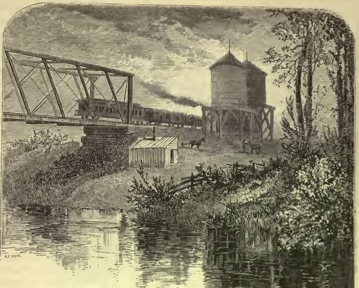
DEEP WATER TANKS.
