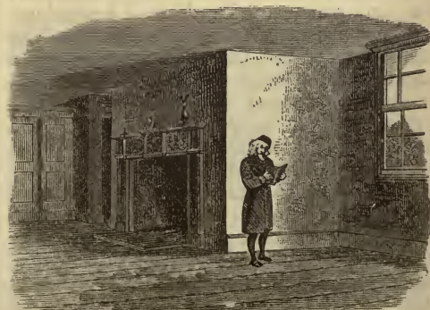
CHIMNEY OF BED-ROOM ON SECOND FLOOR.
