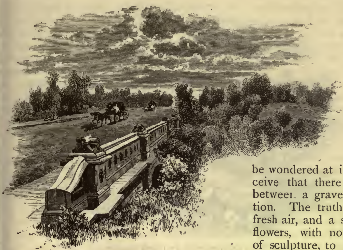
BALCONY BRIDGE, WEST SIDE.
