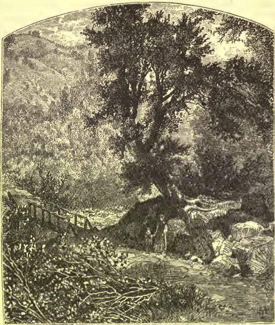
BRIDGE OVER PLUTON CREEK.
