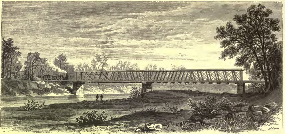
BRIDGE ACROSS NORTH FORK, CANADIAN RIVER—M., K. AND T. RAILWAY.
