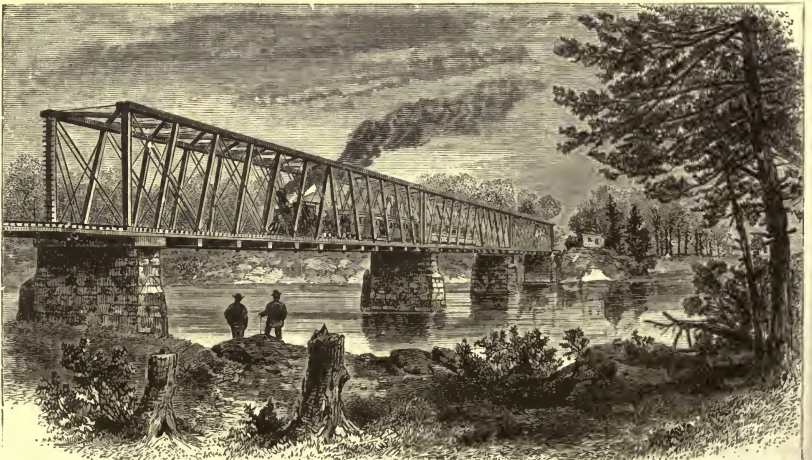
BRIDGE ACROSS THE SOUTH CANADIAN, M., K. AND T. RAILWAY.
