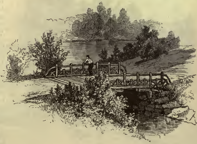
RUSTIC BRIDGE NEAR BALCONY BRIDGE, LOOKING WEST.
