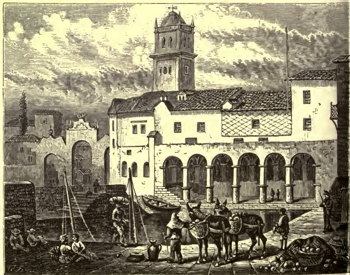
JETTY OF PONTO DELGADO, ST. MICHAEL.
