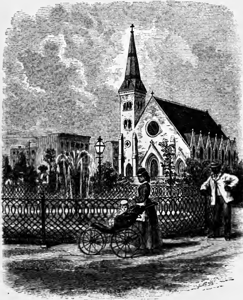
THE FRANKLIN SQUARE PRESBYTERIAN CHURCH, BALTIMORE.
