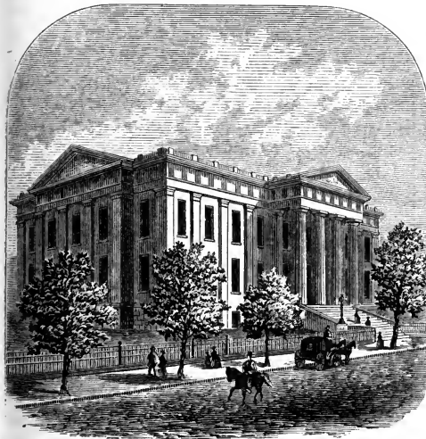
THE COURT-HOUSE — LOUISVILLE.
