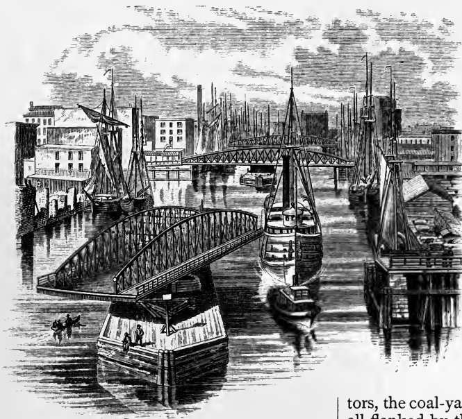
SWINGING BRIDGE OVER CHICAGO RIVER, STATE STREET.
