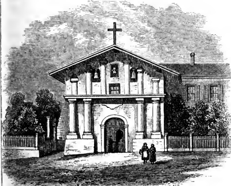
THE OLD MISSION CHURCH (RESTORED).
