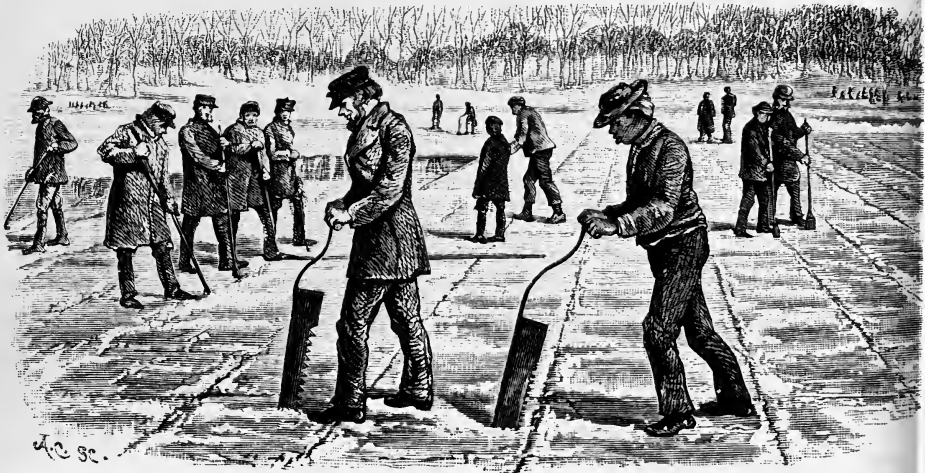
SAWING, CALKING AND BREAKING OFF.
