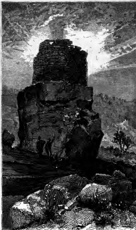
WATCH-TOWER AT MCELMO CAÑON.
