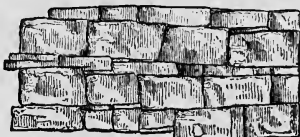
STONE WALL BY AN AMERICAN MECHANIC WHO DID NOT KNOW HIS BUSINESS.
