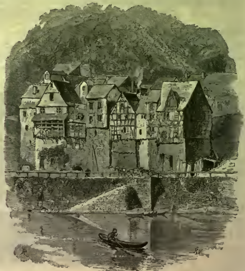
HOUSES ON THE QUAY AT KOCHER.
