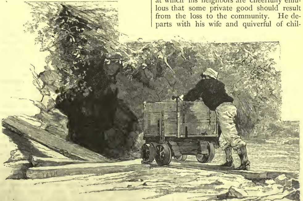
CORNISHMAN "TRAMMING" AT BUSH TUNNEL.
