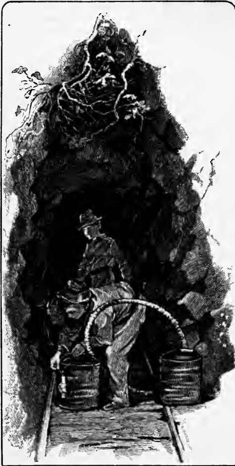
"PACKING" WATER FROM BUSH TUNNEL.
