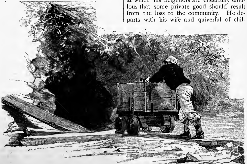
CORNISHMAN "TRAMMING" AT BUSH TUNNEL.
