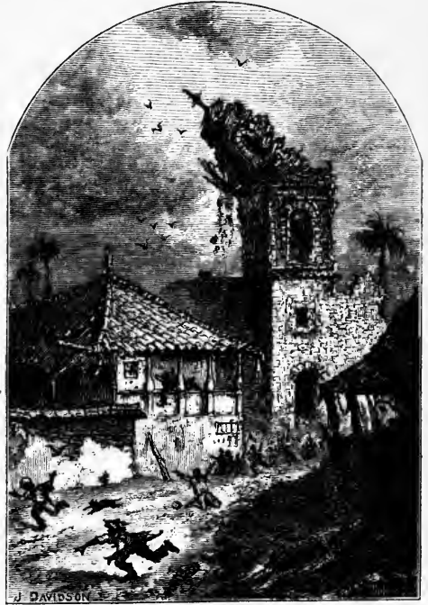
THE FALL OF THE CHURCH TOWER.
