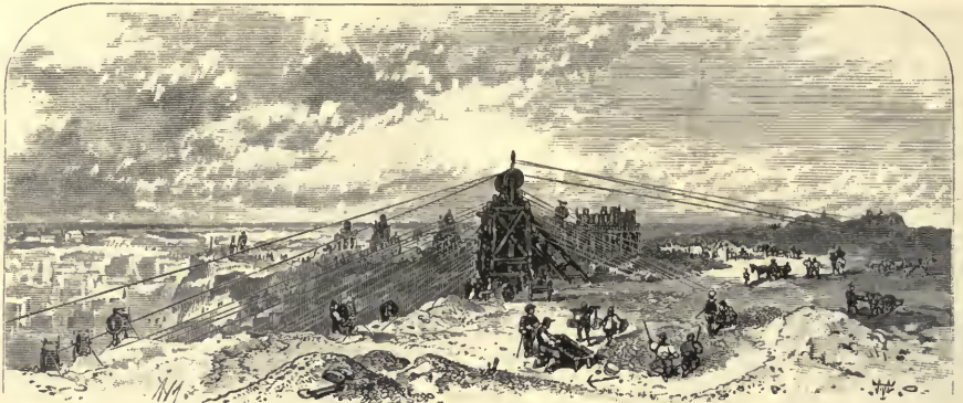
A SECTION OF "STAGING" ON THE EDGE OF THE KIMBERLEY MINE.
