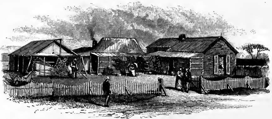
A RESIDENCE AT KIMBERLEY.
